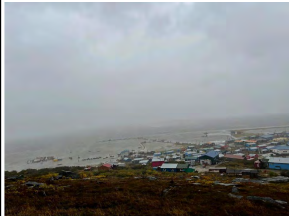
*2022 flooding of the runway (DGGs, 2023b). Note the two (red and blue) airport snow removal equipment buildings on the right side of the picture.
