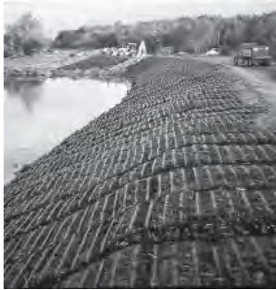
Figure 24. Example of a marine mattress used for erosion protection (Photo source: tensar.com)
