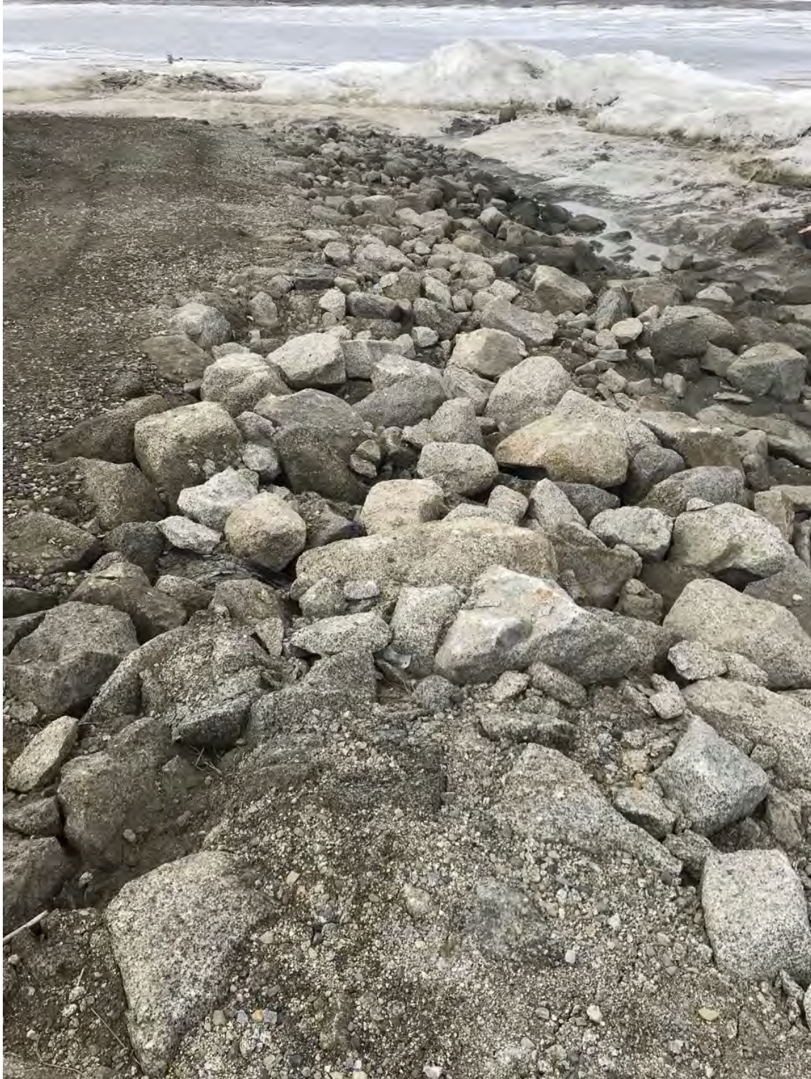
Figure 11. Armor rock protection at western terminal along north edge (looking west). Some rocks observed to be displaced.
