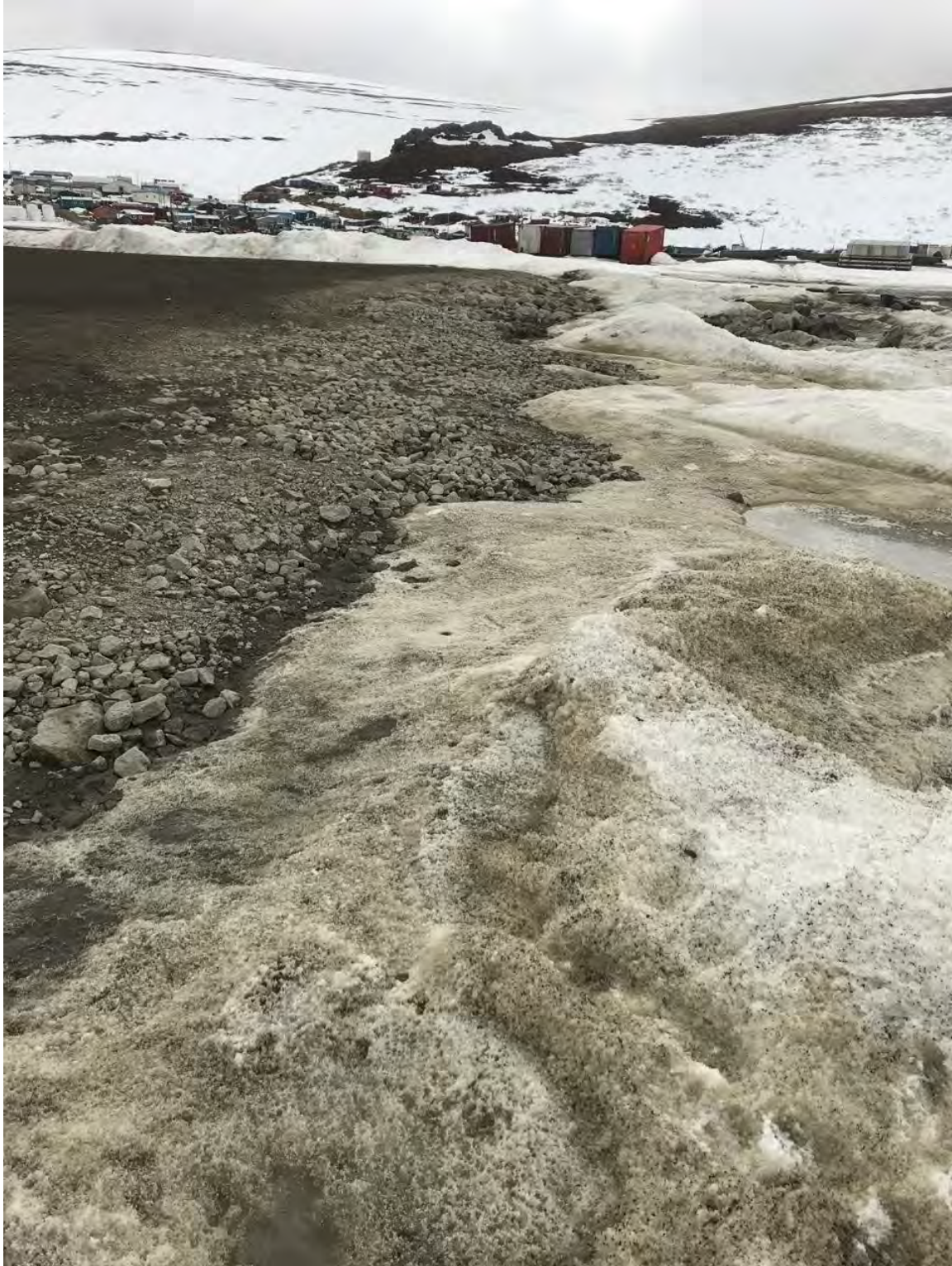
Figure 13. Western runway terminal. No armor rock observed.
