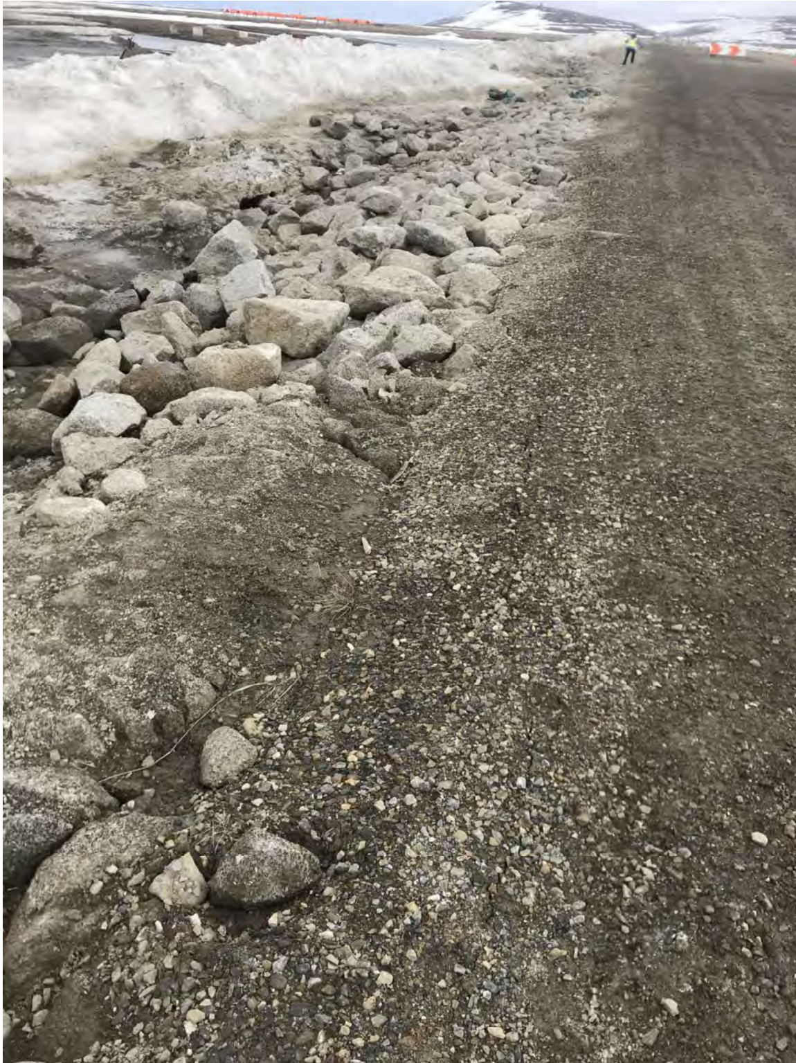
Figure 12. Armor rock protection at western terminal along north edge (looking east). Some rocks observed to be displaced but less than at the western end.
