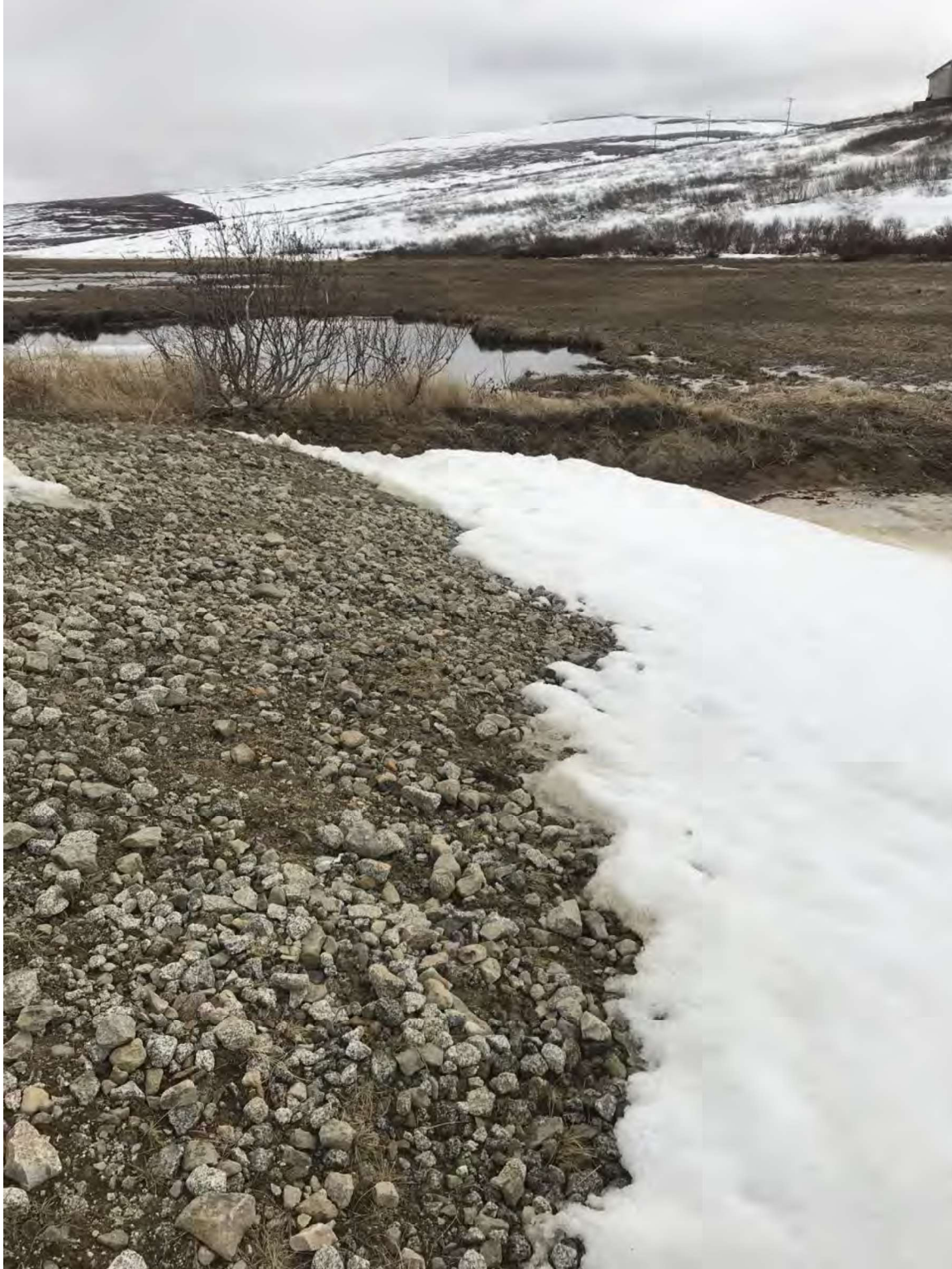
Figure 8. Side slope at windsock (closest point to adjacent elevation). No obvious scour or erosion caused by storm surge/waves.
