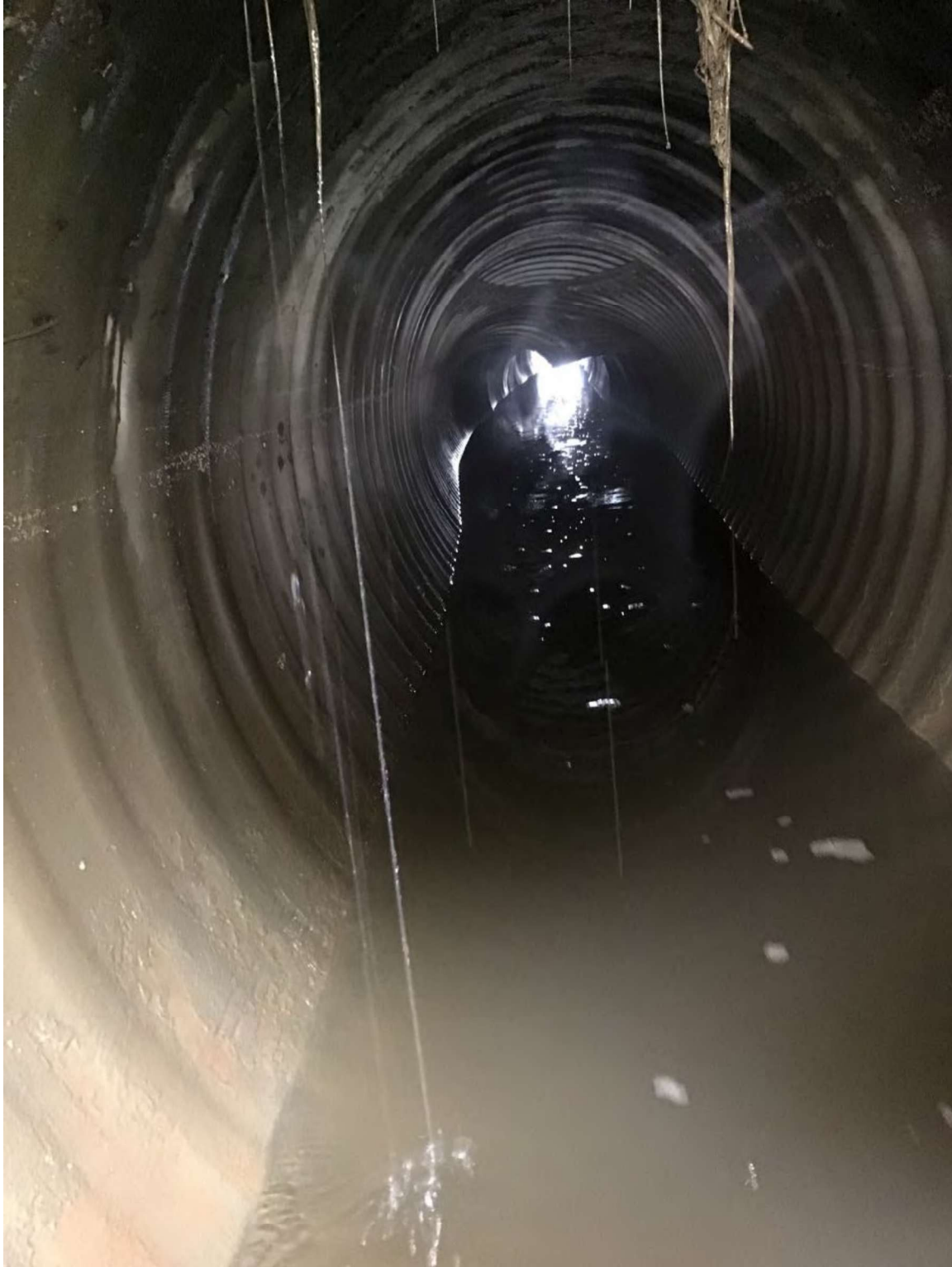
Figure 6. Inside runway culvert looking from outlet to inlet. The culvert was observed to have some sagging and partially collapse in three locations
