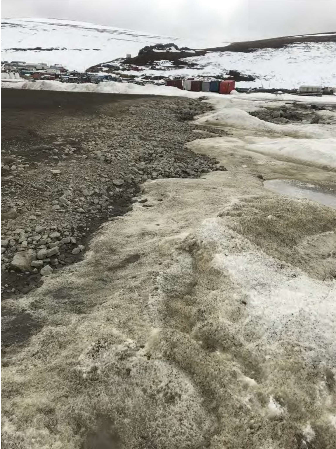
Figure 13. Western runway terminal. No armor rock observed.
