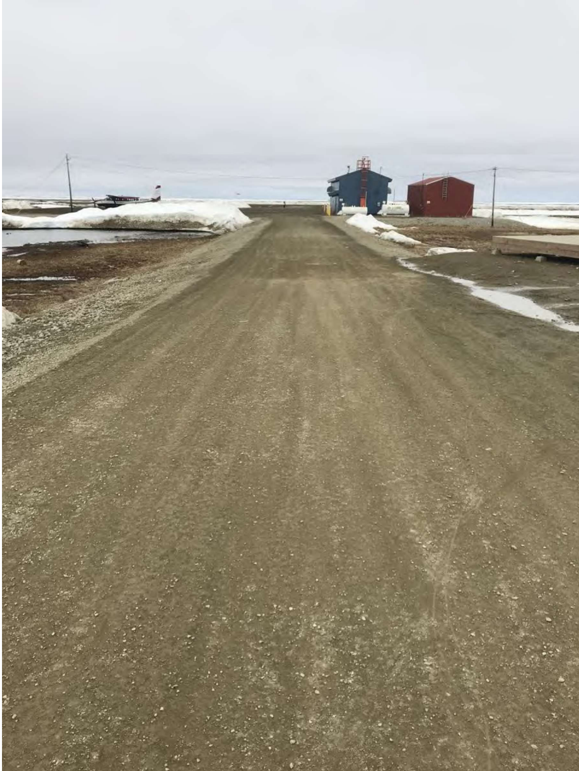
Figure 1. Runway access road. Side slopes appeared to be in good condition – no obvious signs of scour/erosion.
