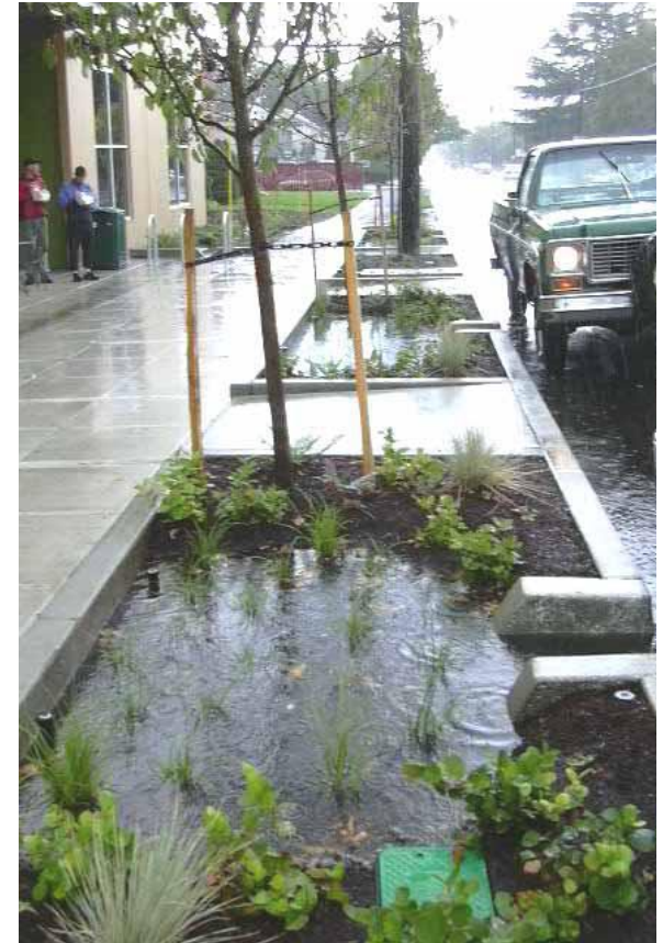
Left: Stormwater planter from National Precast Concrete Association https://precast.org/2014/12/rain-go/ Above Right: Photo from Wilkes East Neighborhood in Gresham, Oregon. http://www.wilkeseastna.org/node/628
