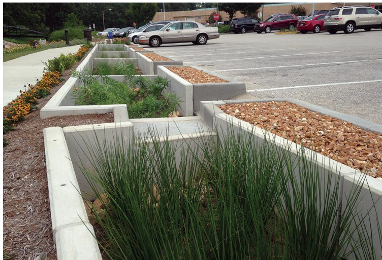
Left: Stormwater planter from National Precast Concrete Association https://precast.org/2014/12/rain-go/ Above Right: Photo from Wilkes East Neighborhood in Gresham, Oregon. http://www.wilkeseastna.org/node/628
