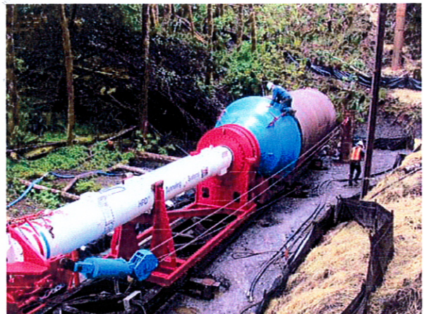
The 60,000-lb hammer is capable of delivering 6 million lbs of thrust
