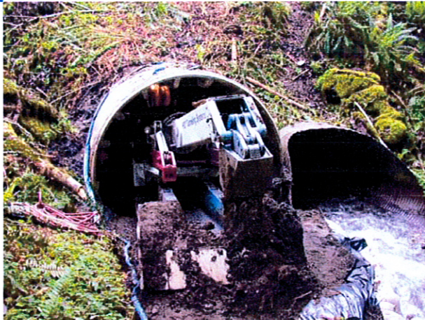
Workers drove 120-in. casing nearly 200 ft in order to replace a failing culvert that carried Quosantana Creek underneath a roadway.
