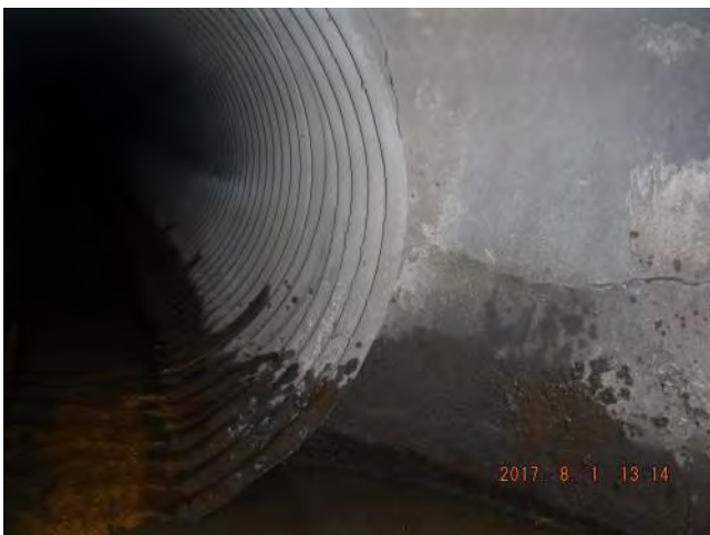
Crack in Base
