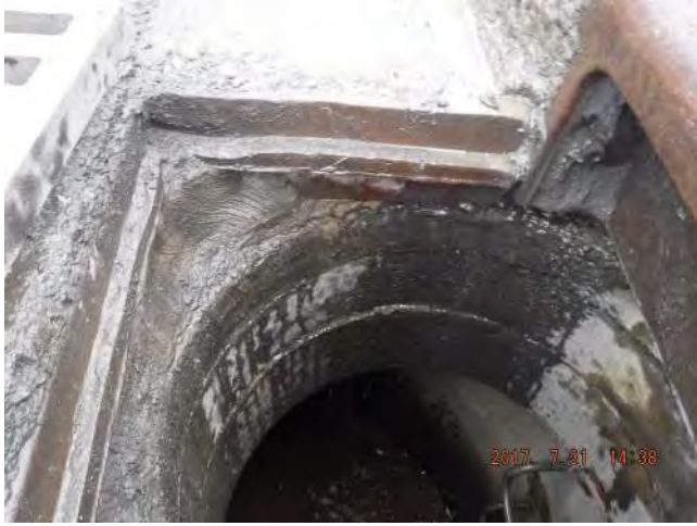
Frame and Chimney, Northeast is up
