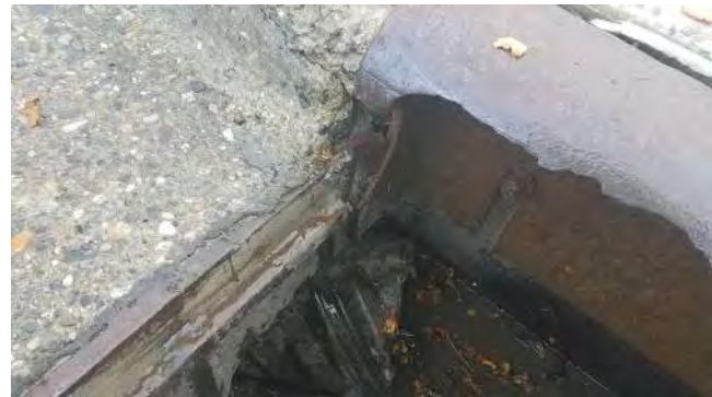
Frame, Broken Curb Inlet
