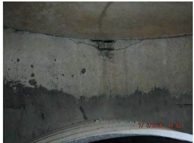
Crack in Barrel
