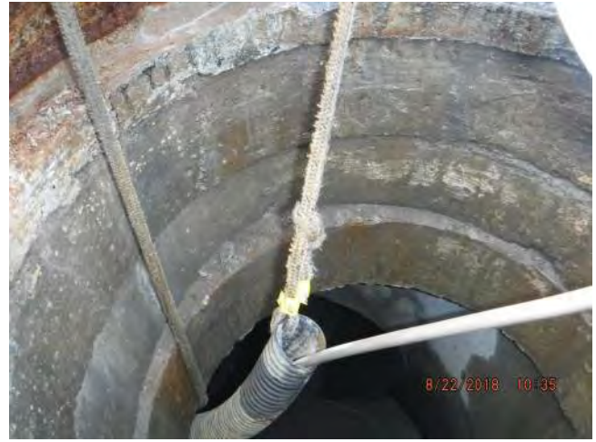
Chimneys and reducing slab
