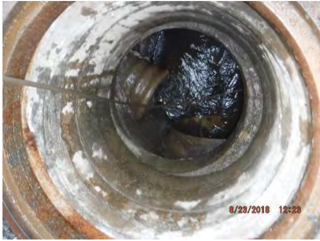
Chimney, offset from reducing slab
