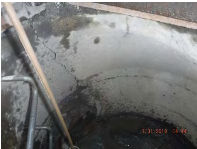
Crack in Base and Cone
