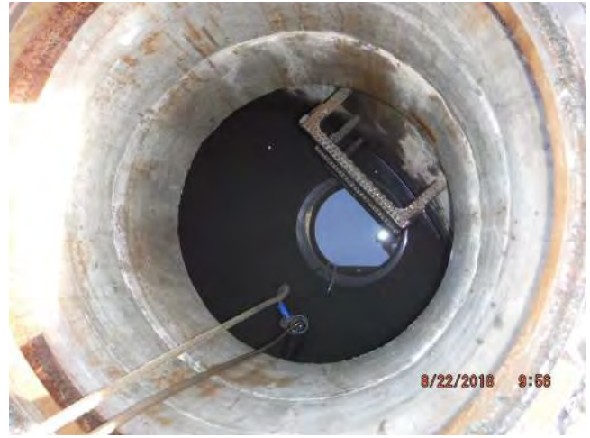
Chimney and reducing slab, north is up
