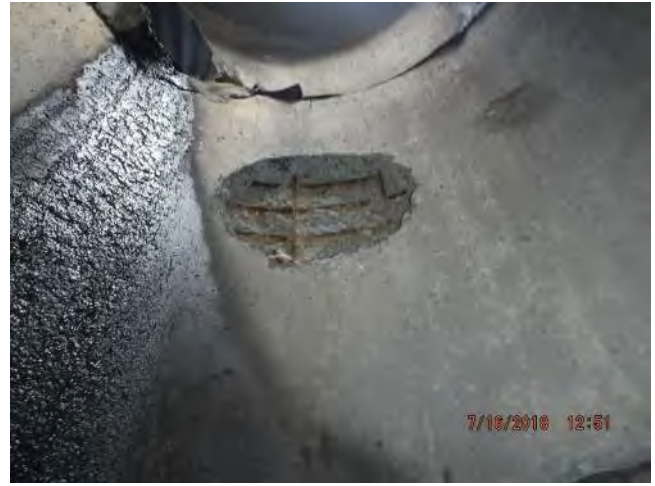
Patch repair to barrel
