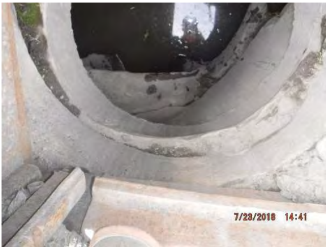
Chimney and Reducing Slab
