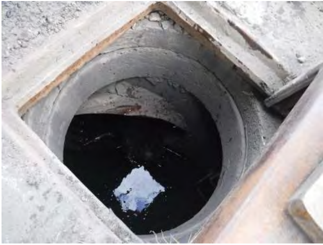
Frame and Chimney, northwest is up
