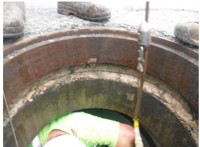
Frame, Chimney, and Reducing Slab
