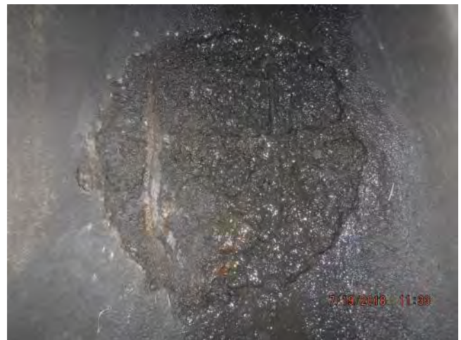
Repair to barrel section
