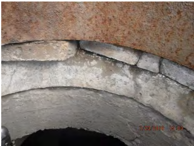
Chimney, Frame, Reducing Slab
