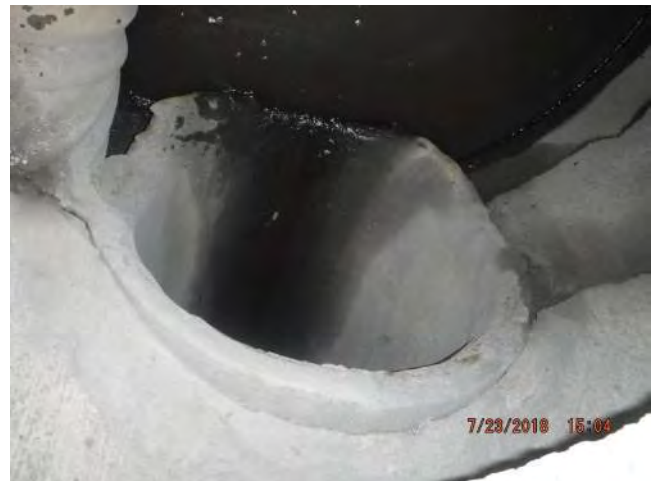
South effluent mainline connection
