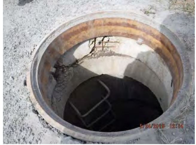
Exposed Rebar in Chimney
