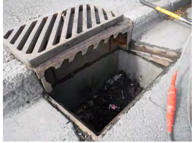
Broken curb inlet
