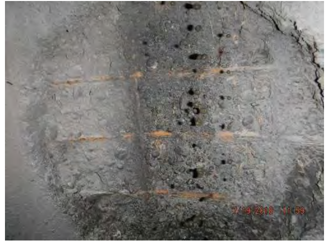
Repair to barrel section
