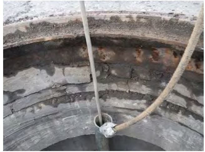
Damage to grade rings
