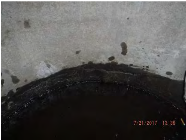
Circumferential crack in base
