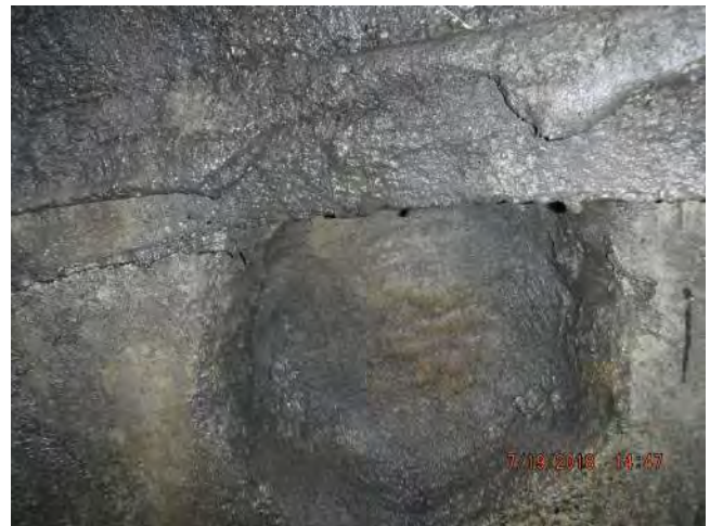
Patchwork done to barrel section
