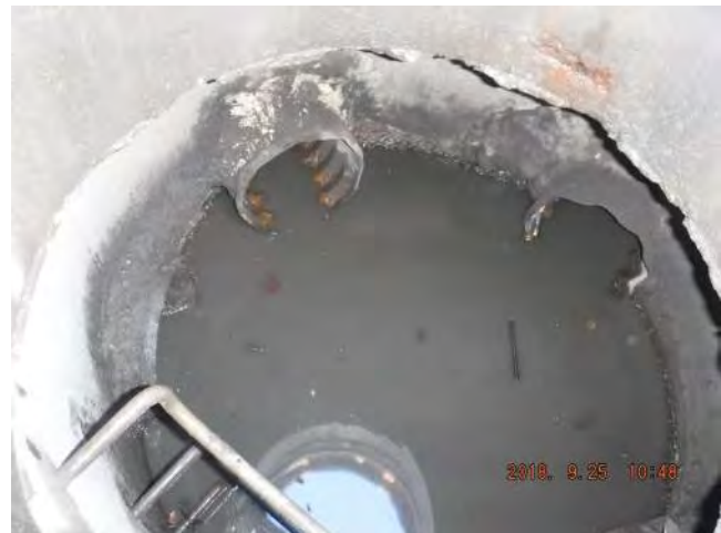
Influent pipe connections
