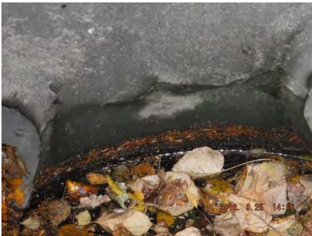
Crack in base
