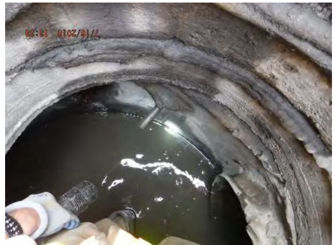
Broken Ladder Rung
