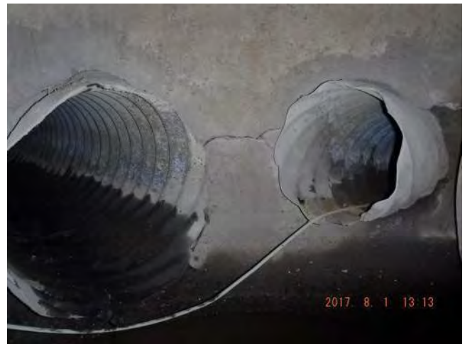
Pipes #6,1, Crack in Base
