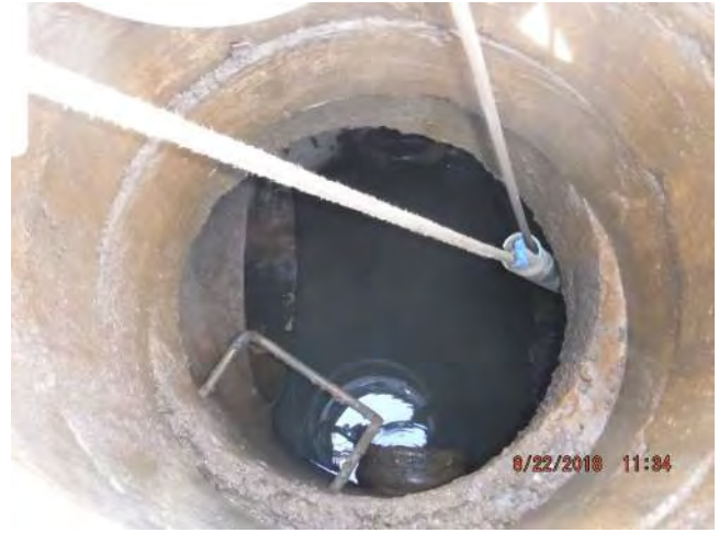
Chimneys and Reducing slab
