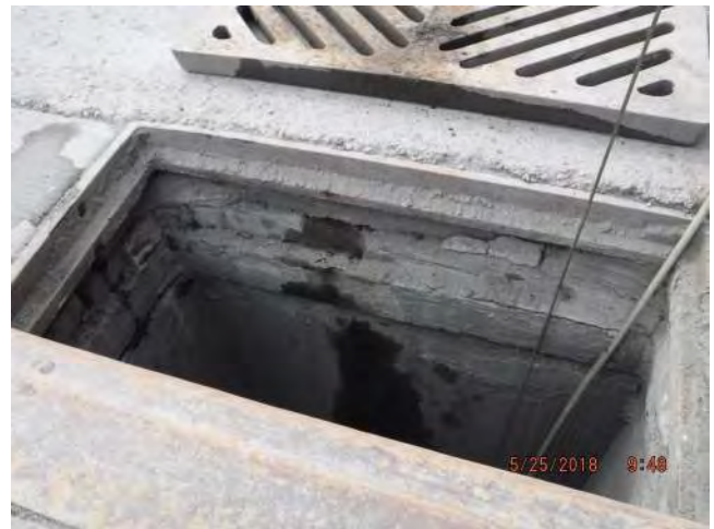
Broke Chimney
