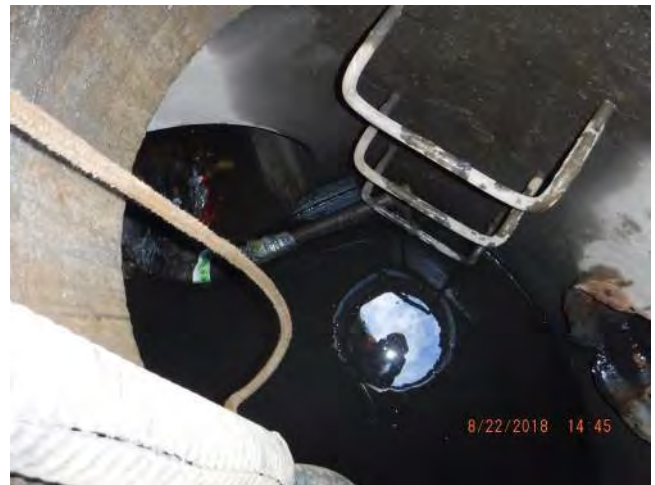
Thaw line in south effluent pipe
