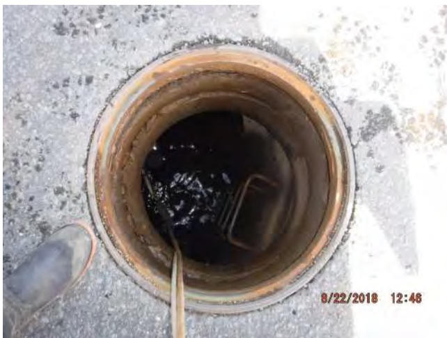
Frame and chimney, north is up
