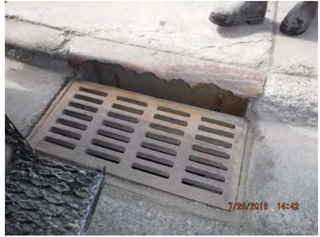
Broken curb inlet
