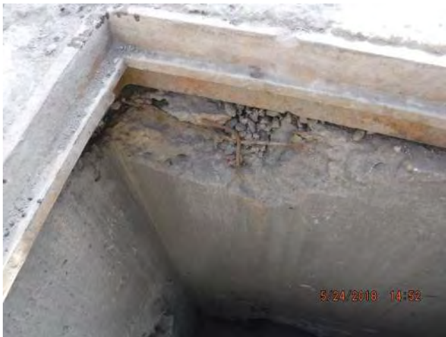
Exposed rebar in manhole wall
