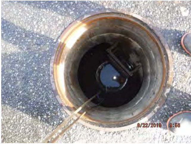
Frame and Chimney, North is up
