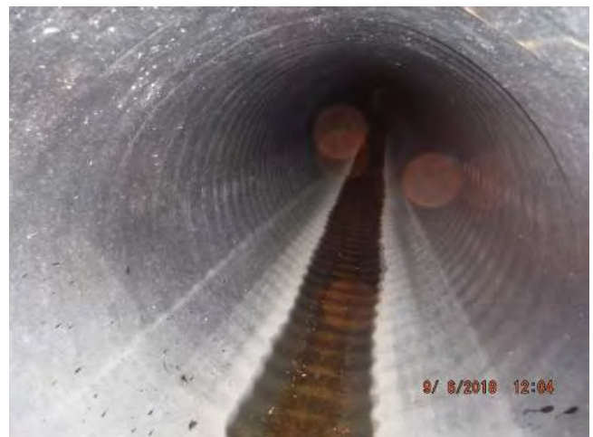
Interior of Pipe #2, CPEP, no defects visible from MH
