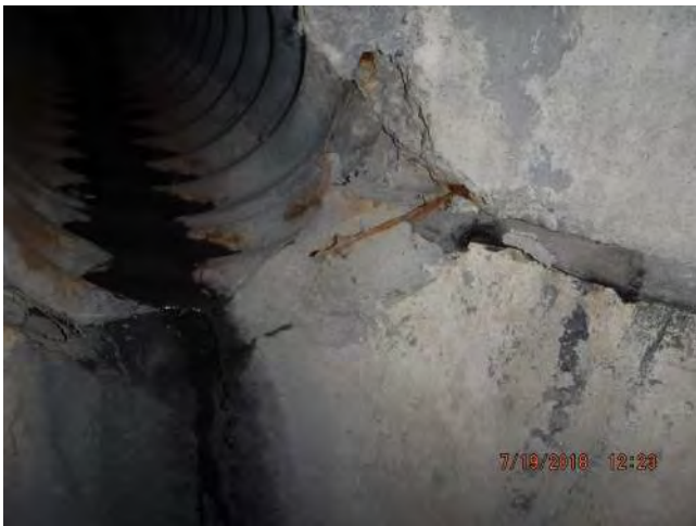
Damage to 554-308 to 554-129 downstream connection
