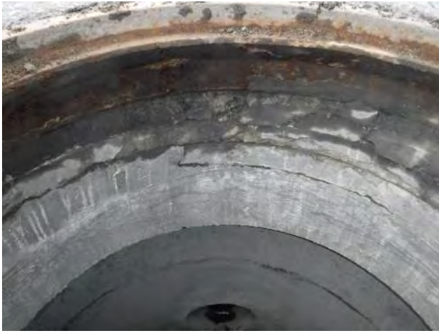
Damage to grade rings
