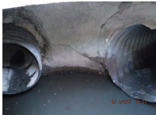
Crack in Base
