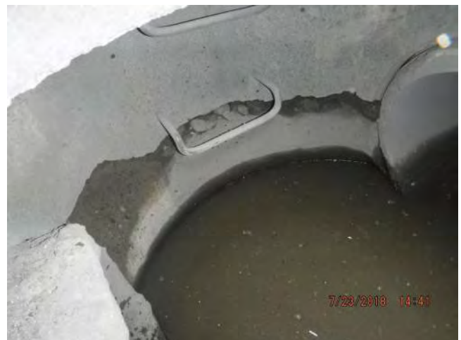
Crack in base
