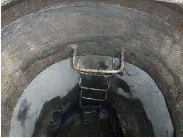
Ladder rung on reducing slab
