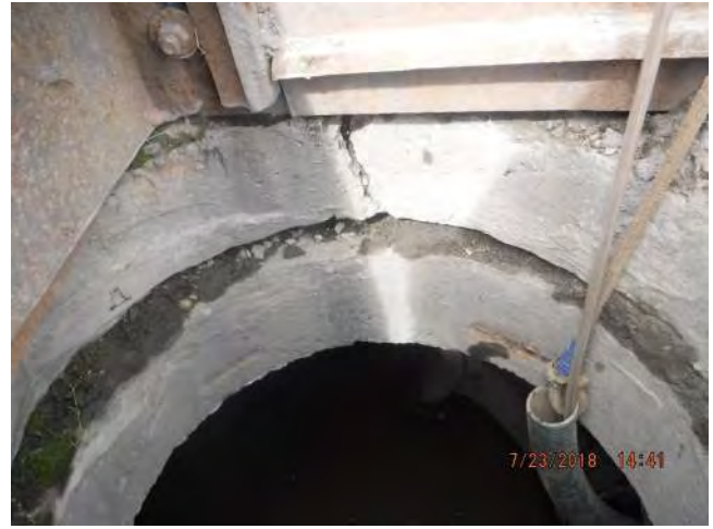
Chimney and Reducing Slab
