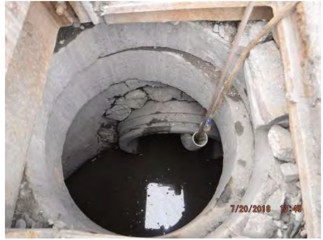
Chimney, Frame, and reducing slab. Missing grout on north influent pipe connection
