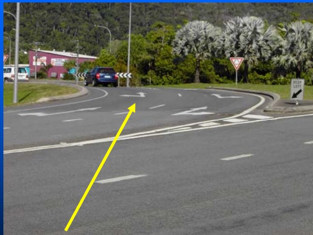
Approach markings to guide drivers to select correct lane at a multilane roundabout 62
