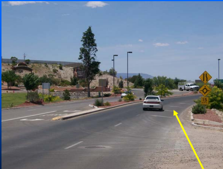
Approach markings narrowed to a single lane on multi-lane roadway 64
