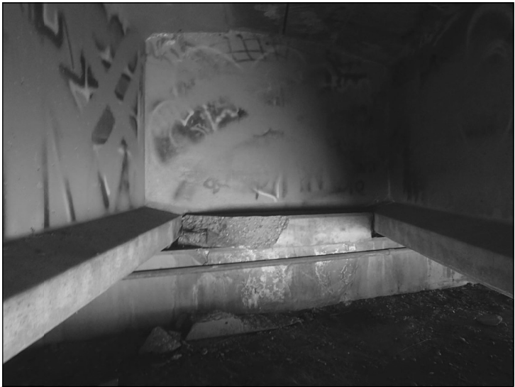
ABUTMENT 3 BAY 10 SHEAR KEY
