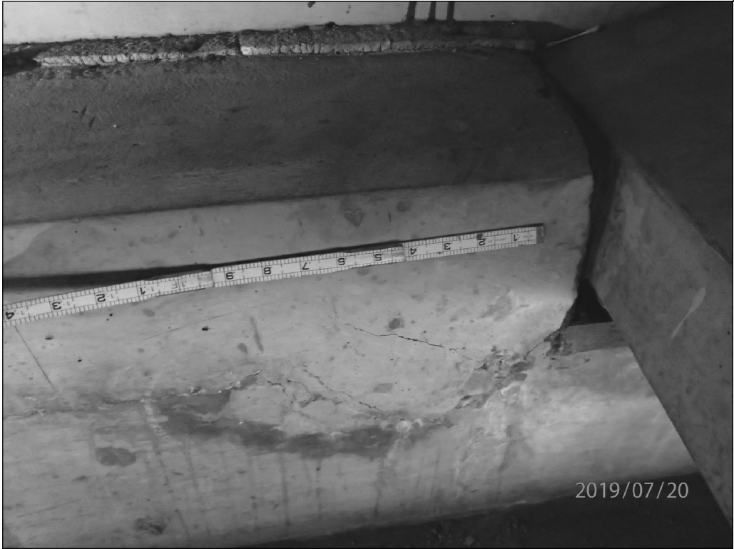
ABUTMENT 1 BAY 3 SHEAR KEY
