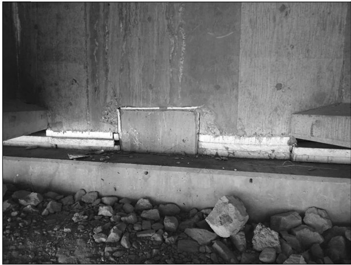
ABUTMENT 1 BAY 7 SHEAR KEY
