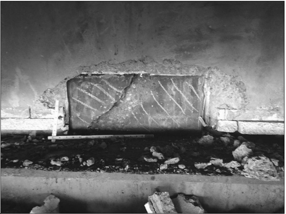
ABUTMENT 6 BAY 7 SHEAR KEY
