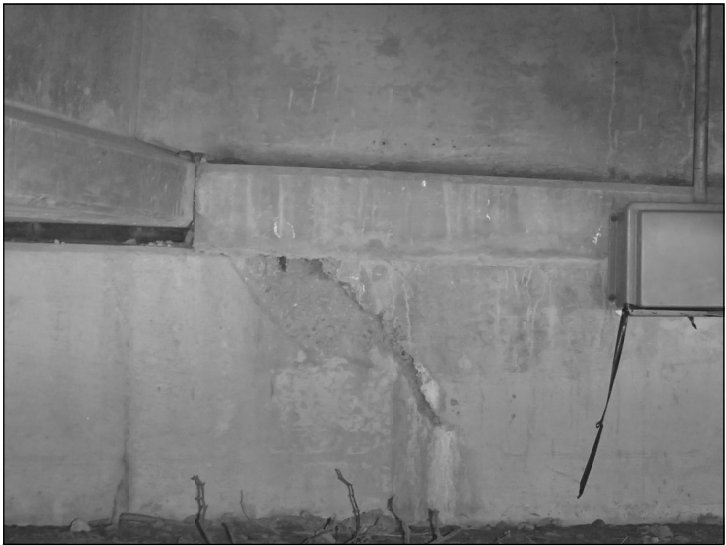
ABUTMENT 1 BAY 3 SHEAR KEY
