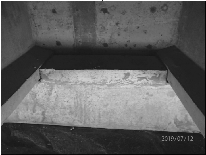
ABUTMENT 1 BAY 4 SHEAR KEY
