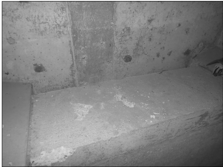
ABUTMENT 1 BAY 2 SHEAR KEY
