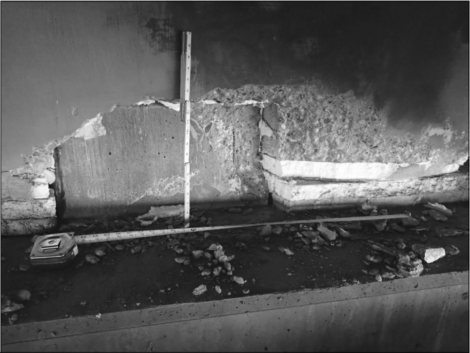
ABUTMENT 4 BAY 4 SHEAR KEY
