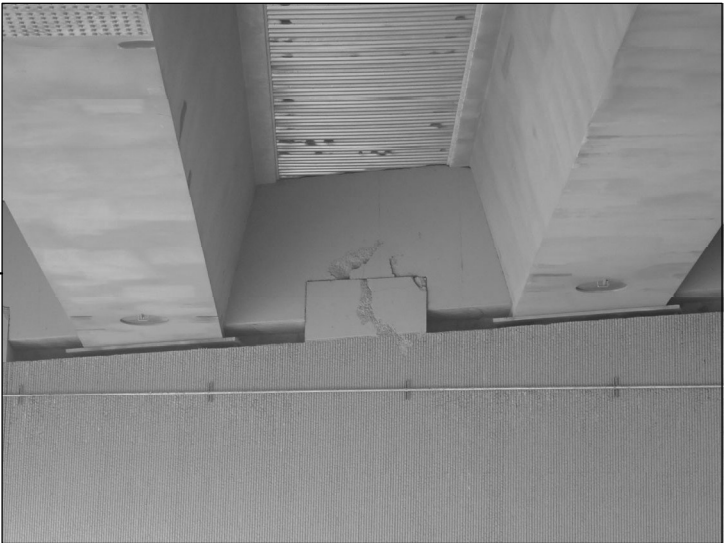
ABUTMENT 1 BAY 2 SHEAR KEY
