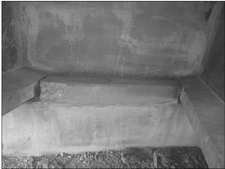
ABUTMENT 1 BAY 12 SHEAR KEY
