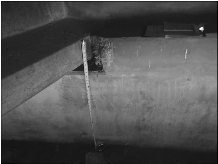
ABUTMENT 1 BAY 8 SHEAR KEY
