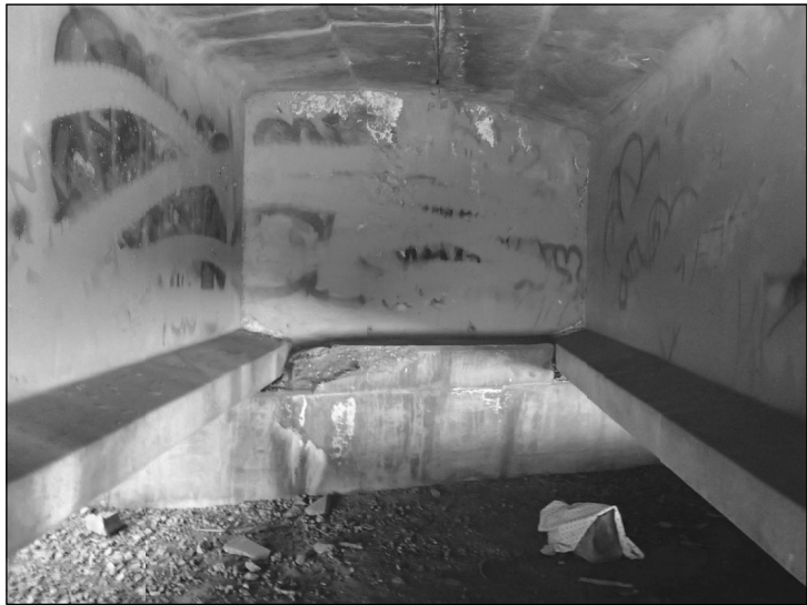
ABUTMENT 3 BAY 1 SHEAR KEY
