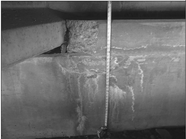
ABUTMENT 1 BAY 10 SHEAR KEY
