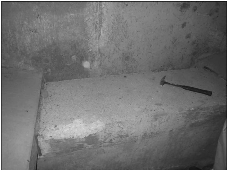
ABUTMENT 1 BAY 2 SHEAR KEY
