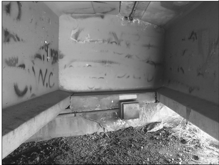
ABUTMENT 3 BAY 12 SHEAR KEY
