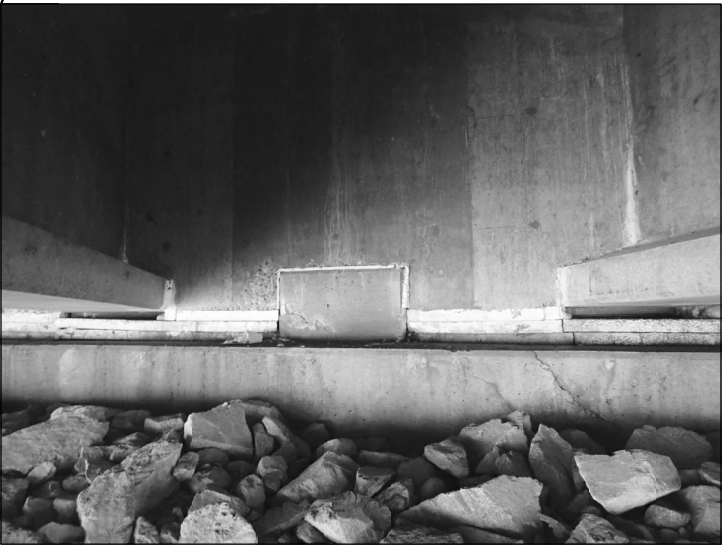
ABUTMENT 1 BAY 4 SHEAR KEY
