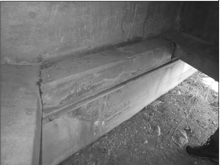
ABUTMENT 1 BAY 1 SHEAR KEY
