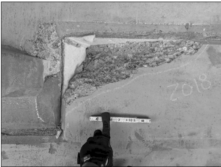
ABUTMENT 2 BAY 2 SHEAR KEY
