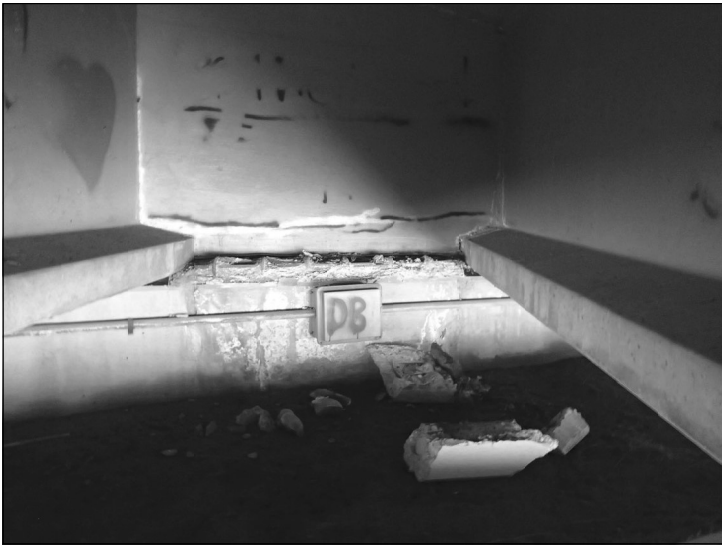
ABUTMENT 3 BAY 8 SHEAR KEY
