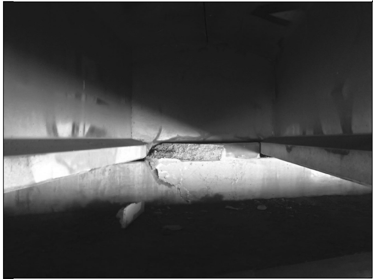
ABUTMENT 3 BAY 3 SHEAR KEY
