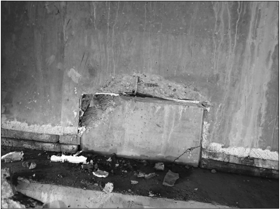
ABUTMENT 1 BAY 10 SHEAR KEY
