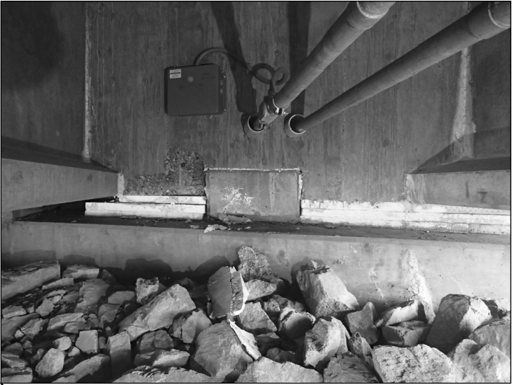
ABUTMENT 1 BAY 1 SHEAR KEY
