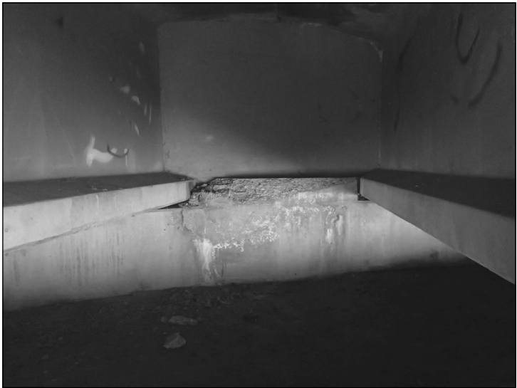
ABUTMENT 3 BAY 5 SHEAR KEY
