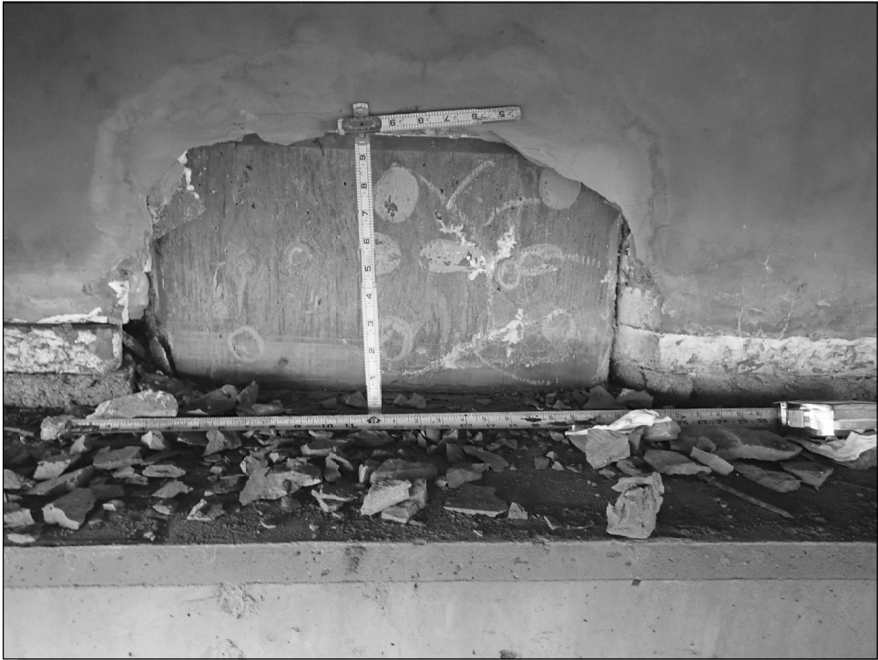
ABUTMENT 4 BAY 1 SHEAR KEY
