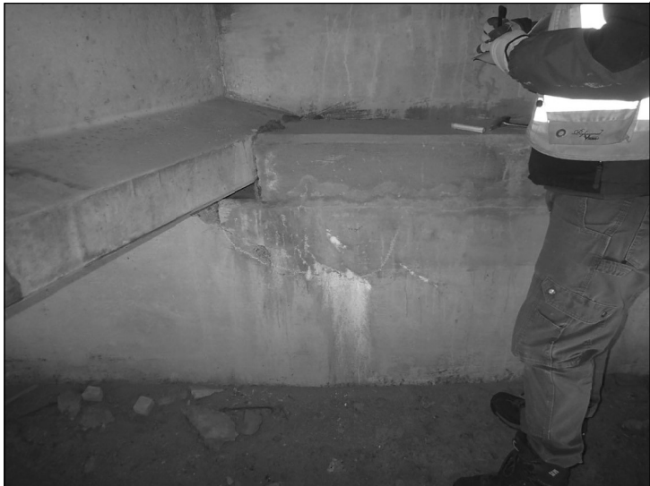
ABUTMENT 1 BAY 5 SHEAR KEY
