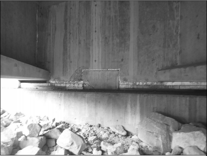
ABUTMENT 1 BAY 10 SHEAR KEY
