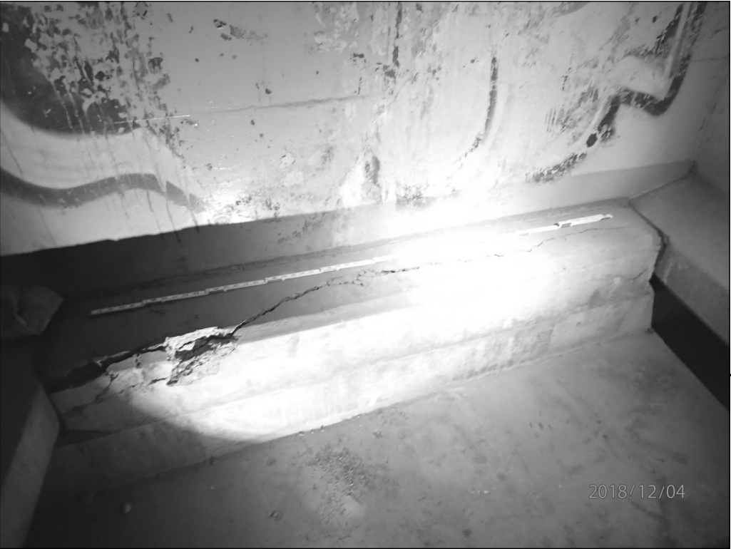
ABUTMENT 3 BAY 5 SHEAR KEY
