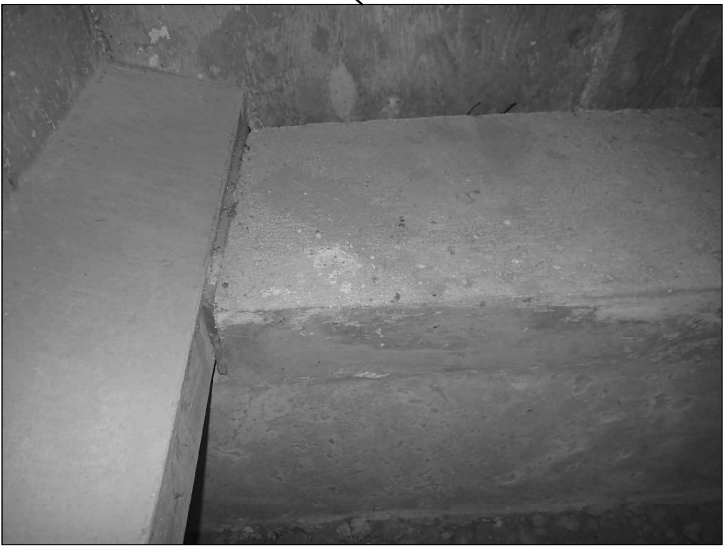
ABUTMENT 1 BAY 4 SHEAR KEY
