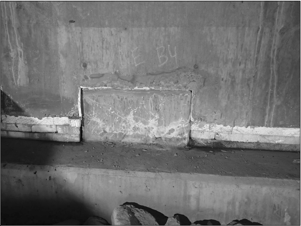
ABUTMENT 1 BAY 4 SHEAR KEY
