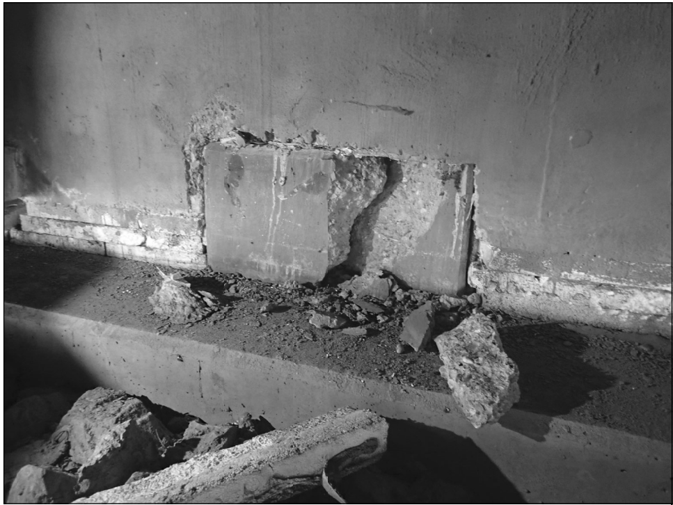
ABUTMENT 6 BAY 4 SHEAR KEY
