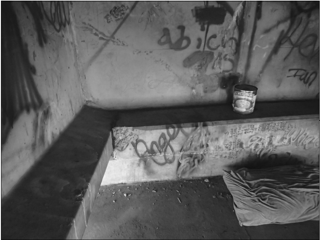
ABUTMENT 1 BAY 5 SHEAR KEY
