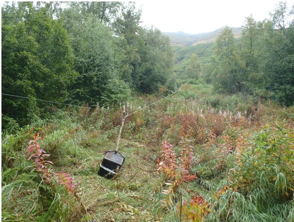
Using a zip line to drag equipment up to power line trail at TH14-22
