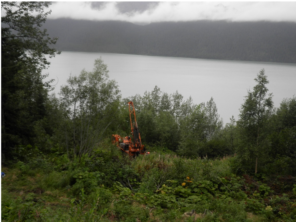
Rig set up below power line access at TH13-16
