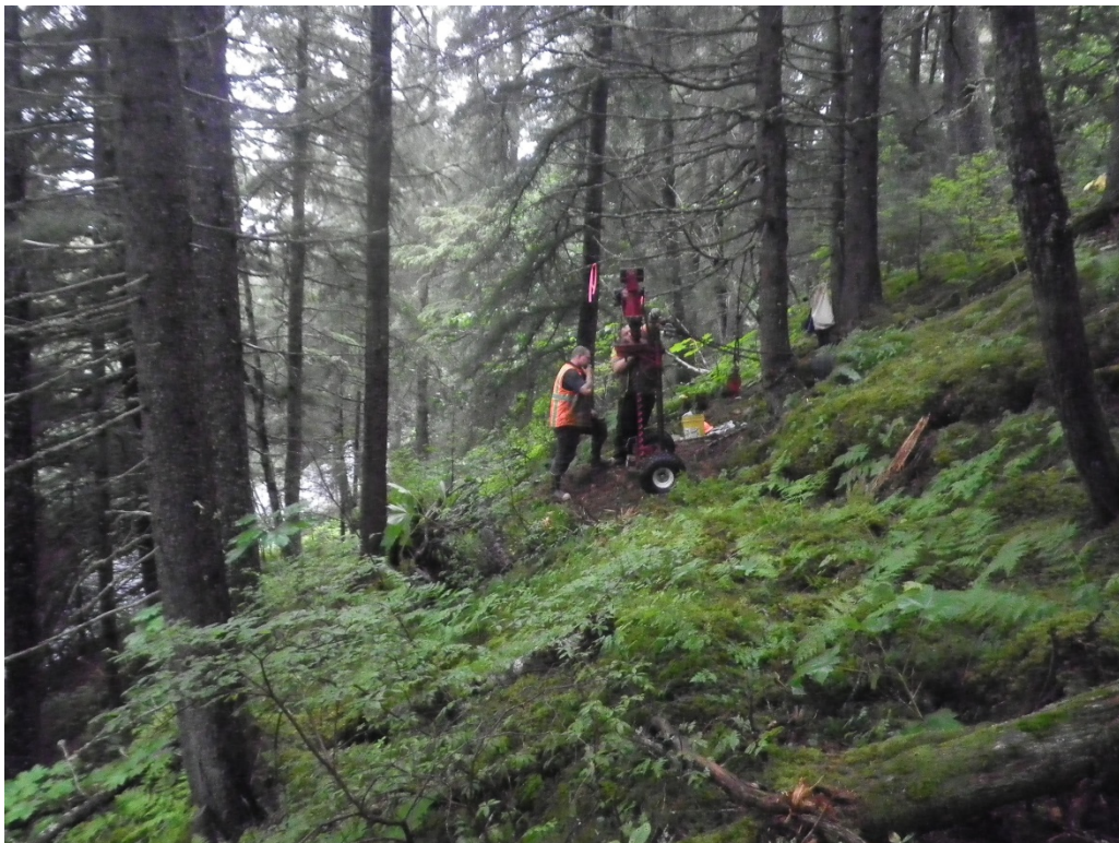
Minuteman drill on slope above road
