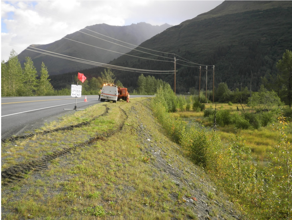
TH13-14 Looking east toward Snow River bridge(s)
