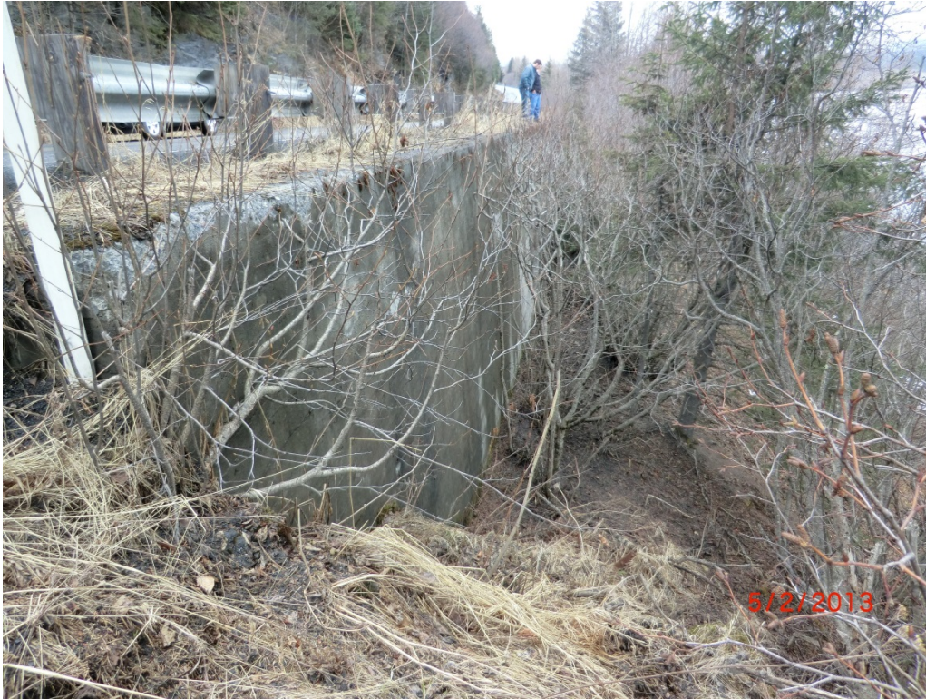
Concrete retaining wall at STA 182+50
