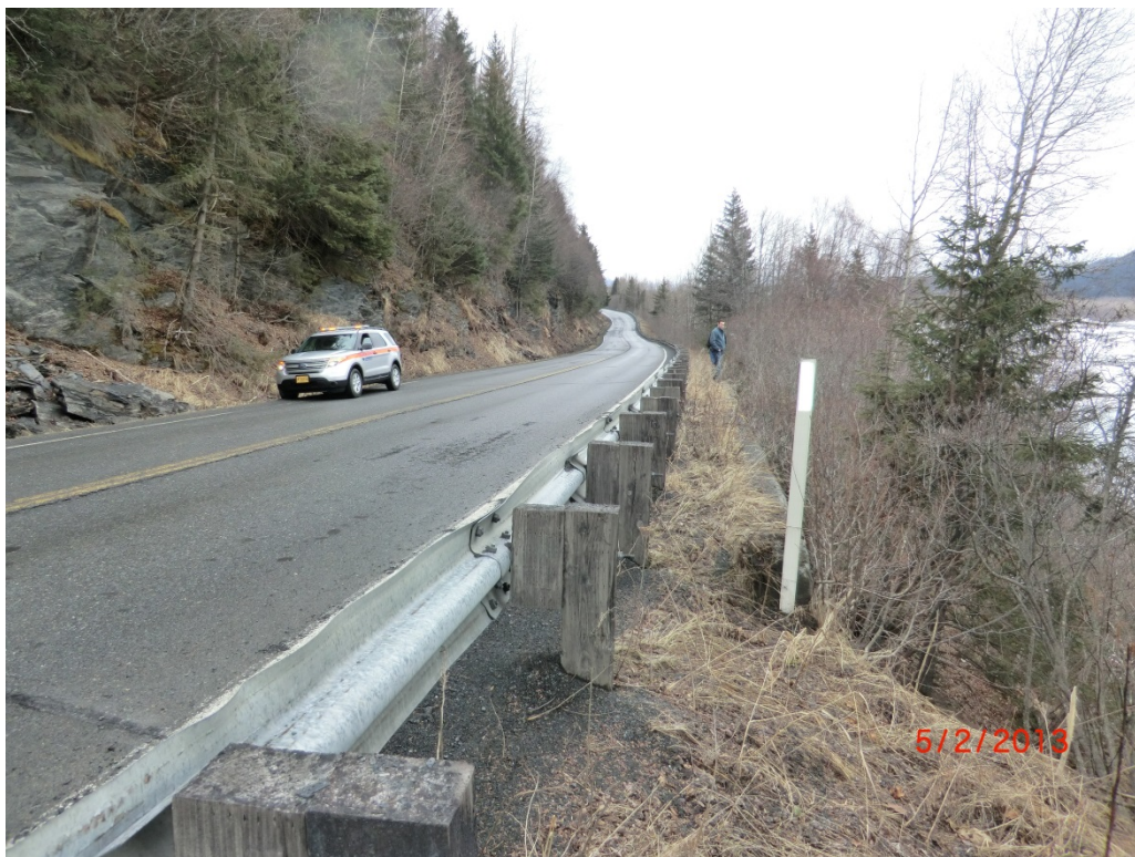
Concrete retaining wall at STA 182+50
