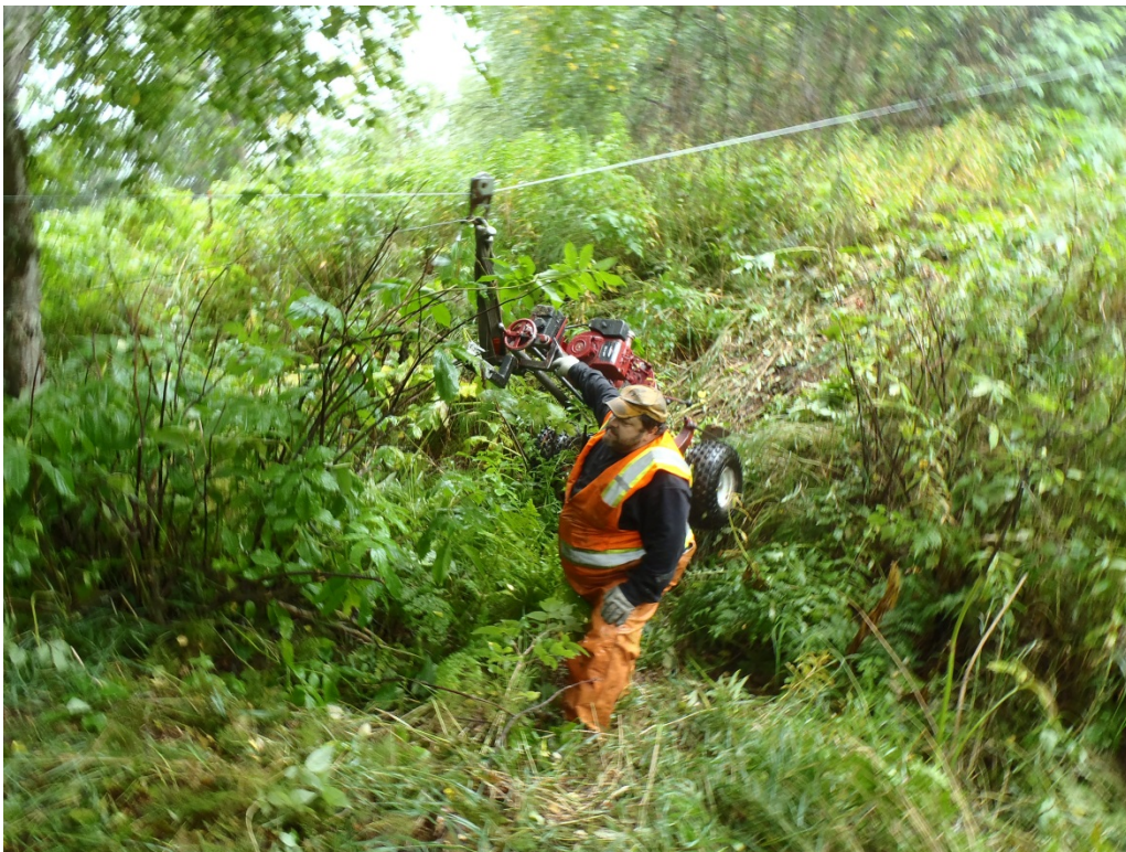
Maneuvering Minuteman to boring location using zip line during 2014 field efforts
