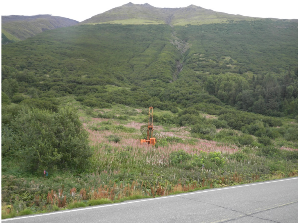
Drill rig set up in the "horse pasture" at TH13-05, looking east
