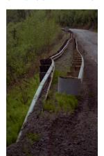
Top of W-Beam guardrail less than 26 - 1/2" when spliced at post only (2017 and earlier installations.)
