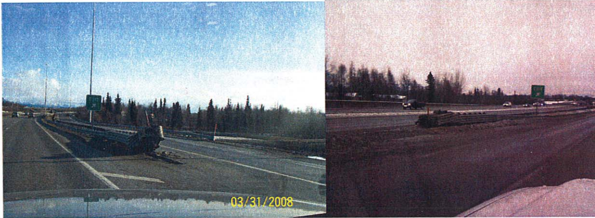
2008 and 2013 Crash cushion failures on Minnesota Drive. Interlock at ground level.
