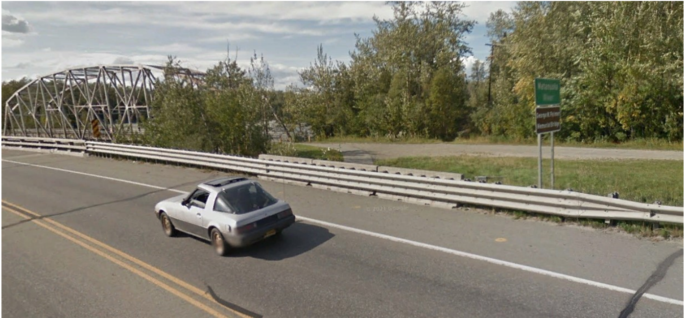
1994 Long Span Concrete Barrier and symmetric three beam transition over pipe and shallow gas main, Old Glenn Hwy Palmer
