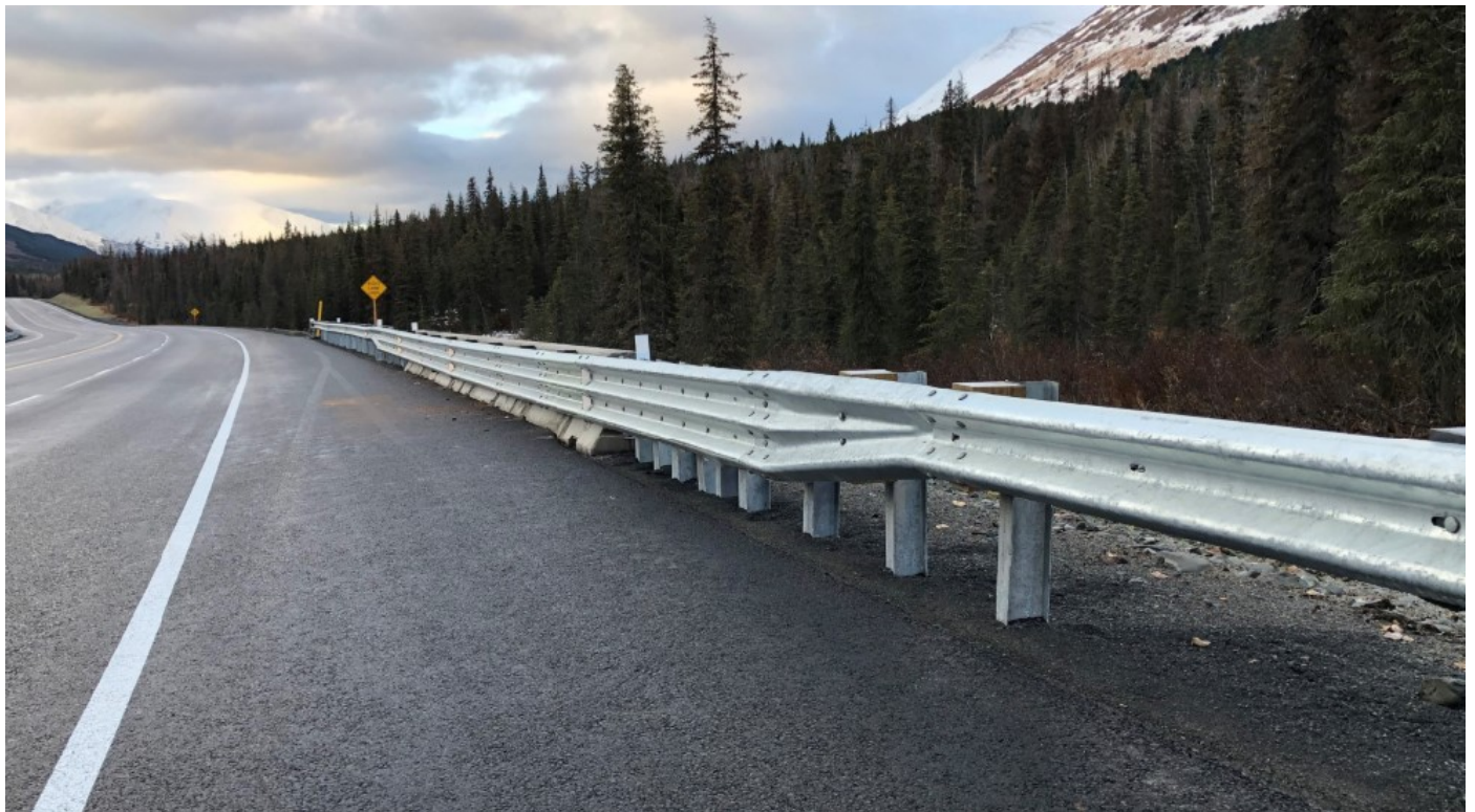
2022 CR-G-28 Implementation of W31 to Asymmetric Thrie Beam to Concrete Barrier over Low Fill Pipe Arches, Seward Hwy Summit Lakes area (1 of 4)
