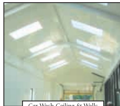
Car Wash Ceiling & Walls
