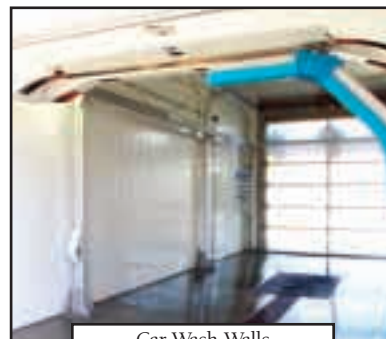
Car Wash Walls
