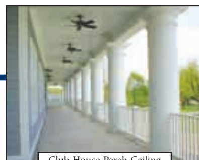
Club House Porch Ceiling
