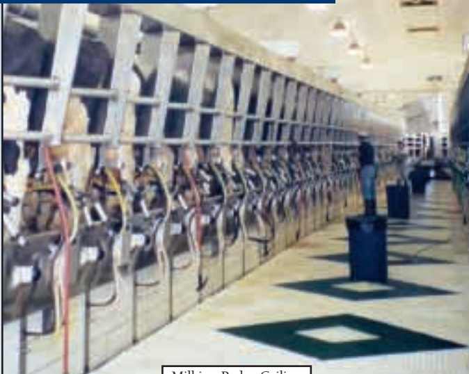
Milking Parlor Ceiling
