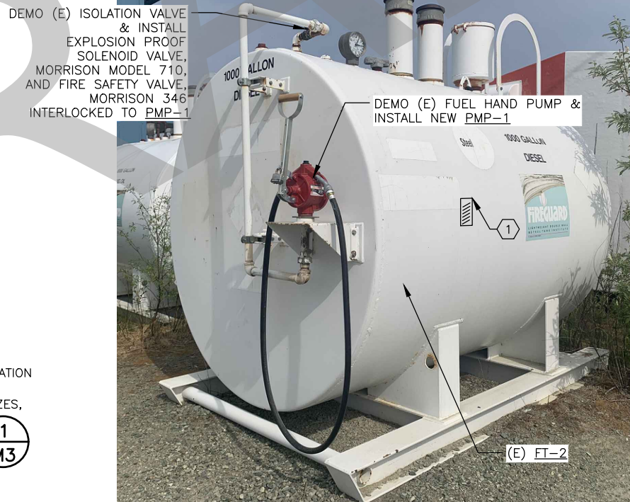
5 FUEL DISPENSING TANK DETAIL M3 NOT TO SCALE
