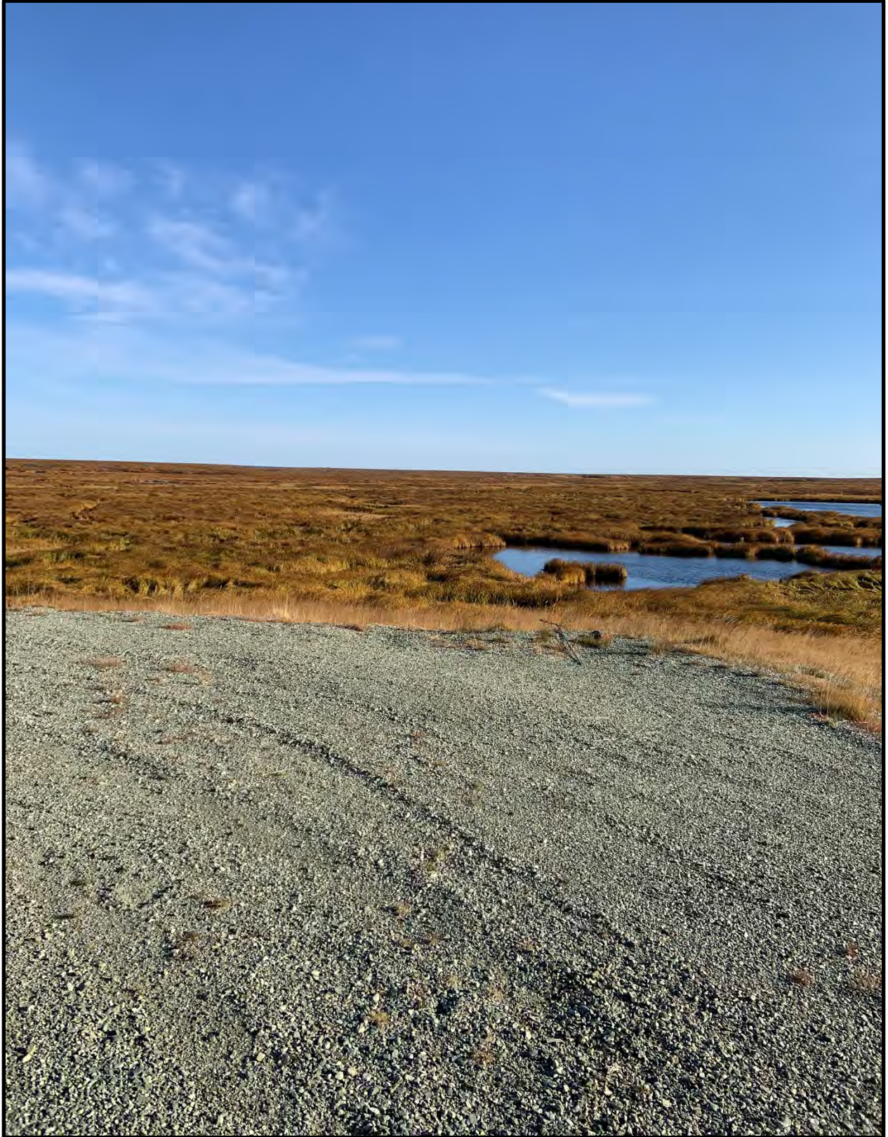
Figure 4c. Site Photos of Expansion Areas, north RSA extension from above. From Central Region Aviation Design Section.
