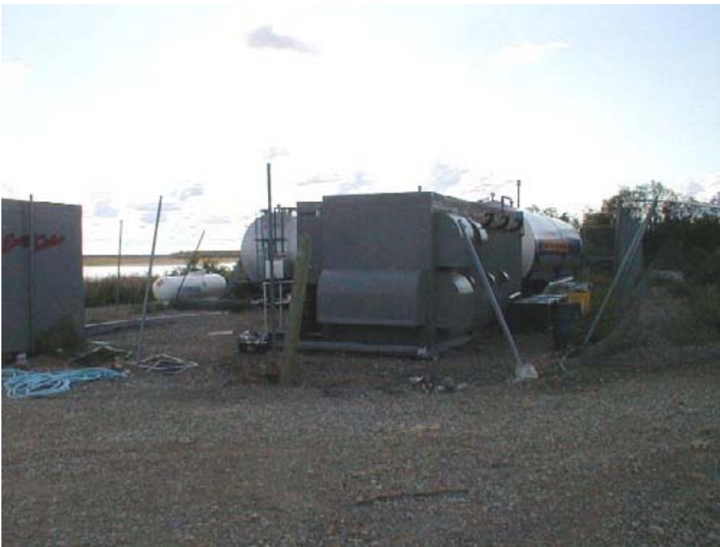
City's power plant - new generator and bulk fueling tanks (generator not operational)
