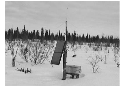
Photo 2 – Solar Panel used for strobe lights at ends of the runway
