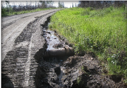
Failing Drainage
