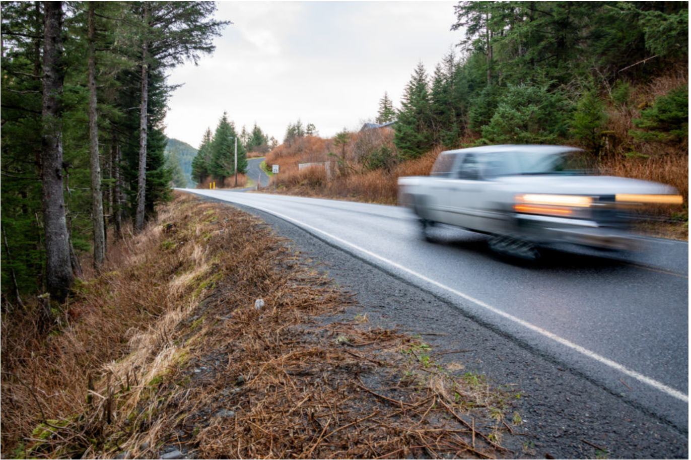
Lack of a dedicated shoulder along Whitshed Road poses a hazard to pedestrians and cyclists, according to the Department of Transportation & Public Facilities. (Dec. 12, 2019) Photo by Zachary Snowdon Smith/The Cordova Times
