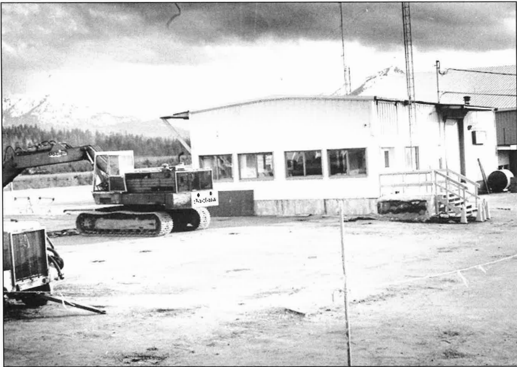
In June 1991 Alaska Airlines began construction of a new passenger terminal at the Petersburg airport. The existing 2,275 sq. ft. terminal, built in 1973, was remodeled to house cargo, maintenance and service operations for the airline. Initially, the airline operated from a trailer parked near the gravel runway.
