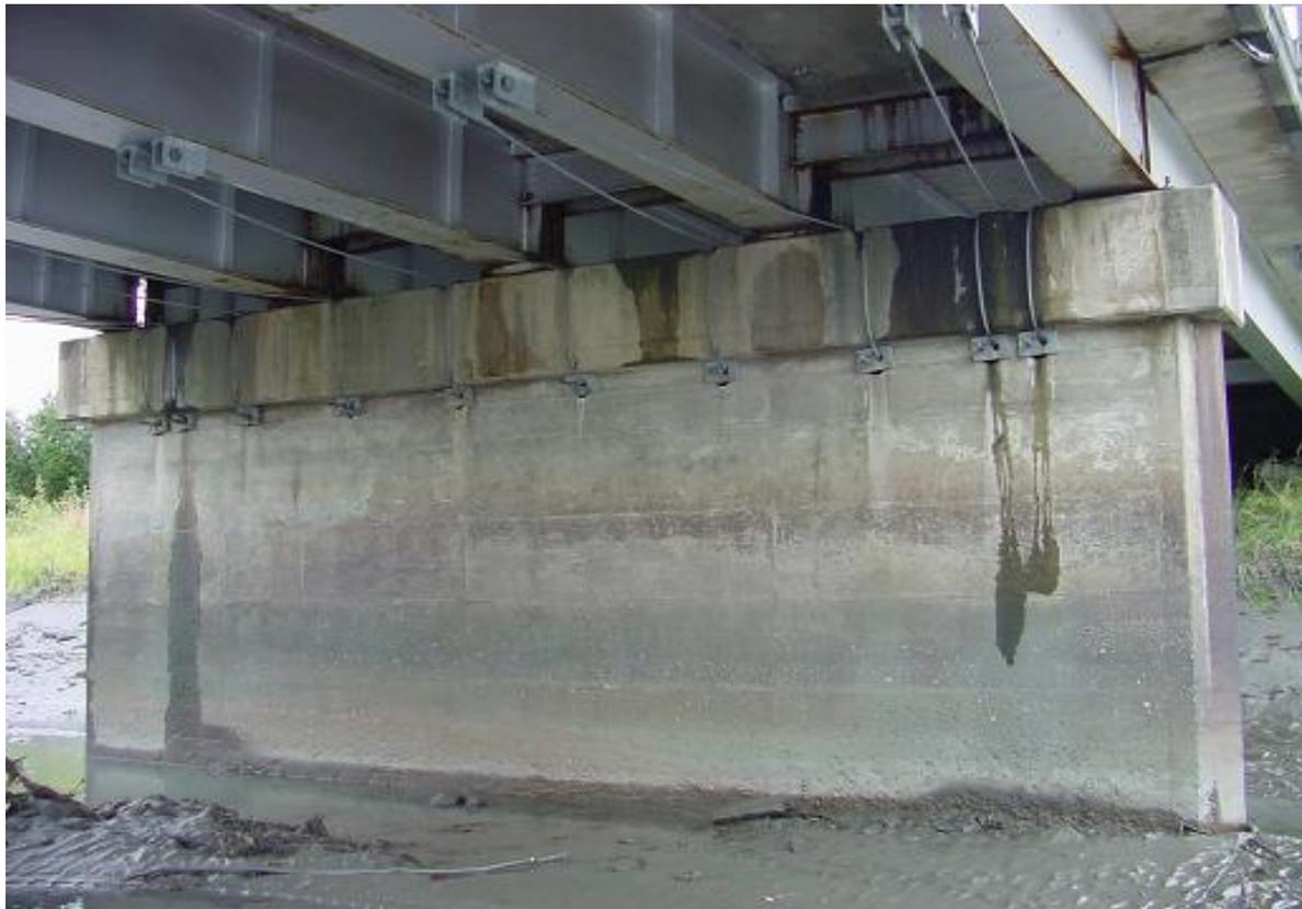
Figure 10. Phase 1 Seismic Retrofit Using Cable Restrainers
