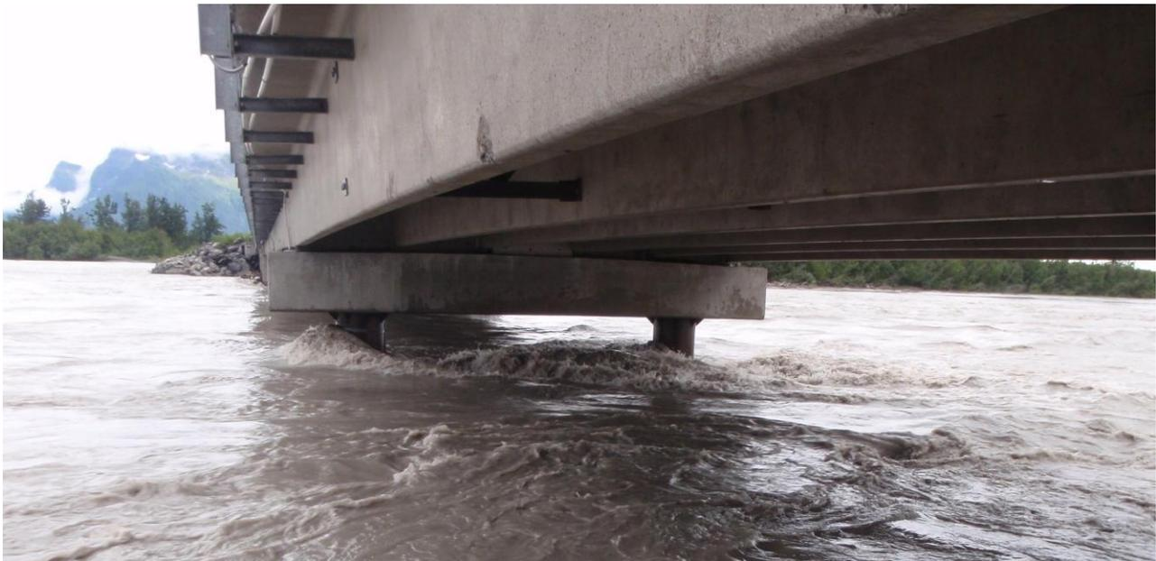
Figure 8. Active Scour on Bridge #339, Copper River Highway
