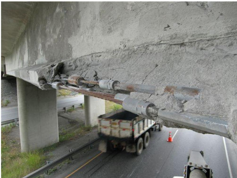
Figure 13. Highway Overpass Damaged by a Vehicle Collision
