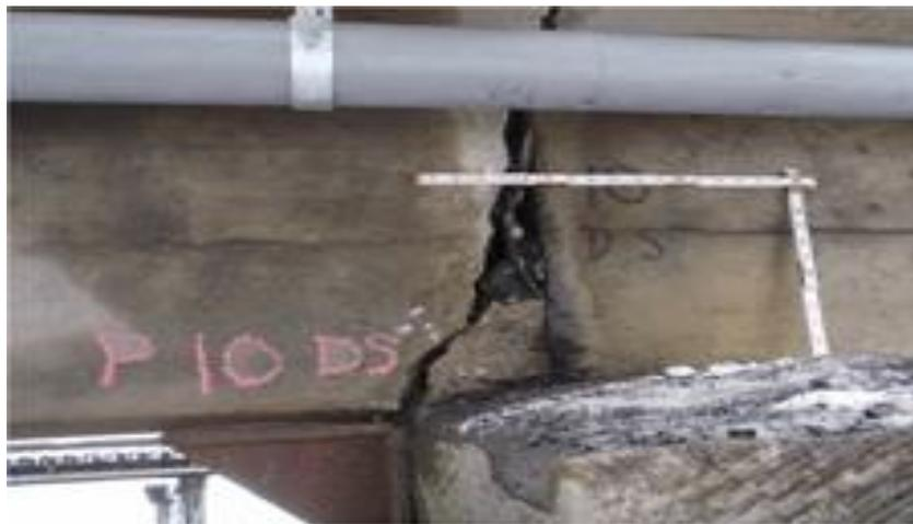
Figure 6. Deteriorating Concrete Trail River Bridge
