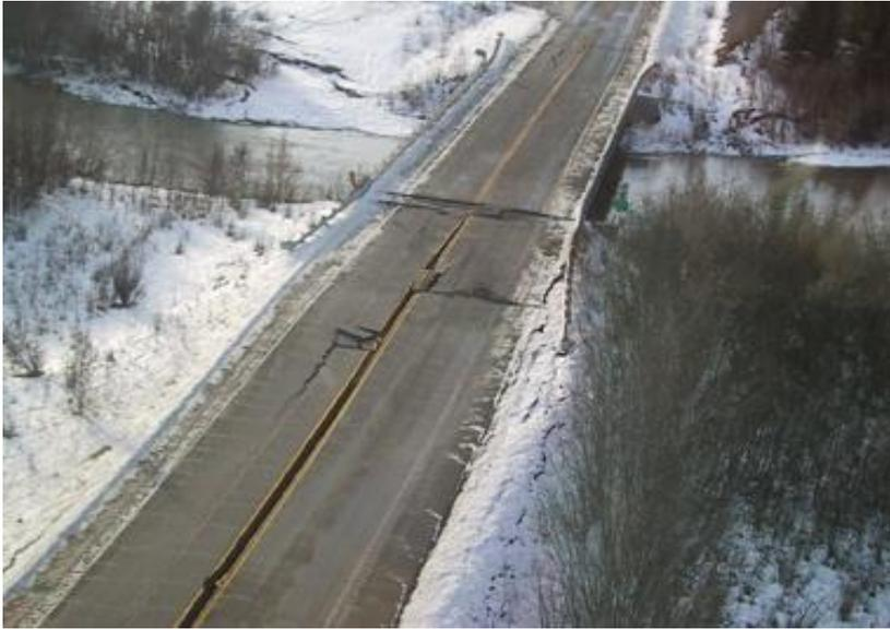
Figure 9: Earthquake Damage on the Richardson Highway
