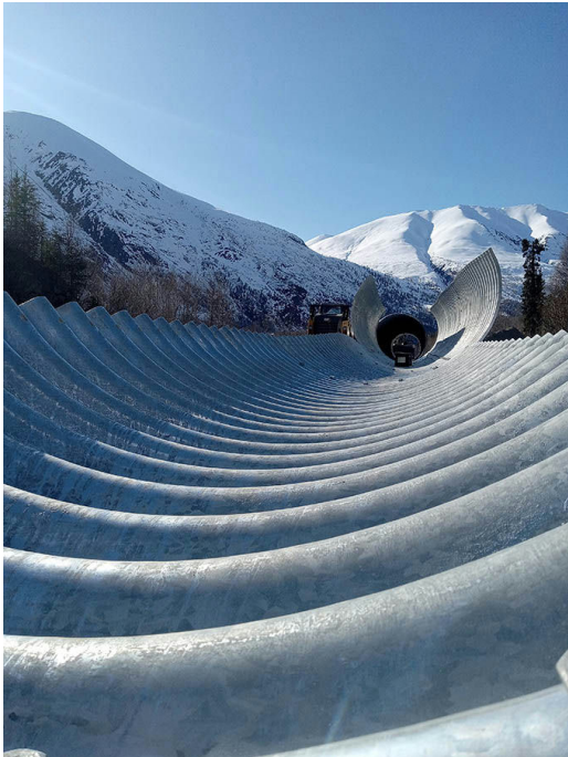
Photo Credit: "Mary Brunner, DOT&PF" Description: Structural plate pipe assembly, Richardson Highway MP 40-51 Resurfacing.
