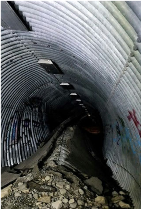
Photo Credit: "Staff , DOT&PF" Description: Earthquake Culvert Repair
