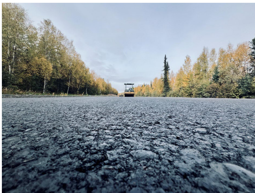
Finish roller follows the rest of the paving train on Richardson Hwy MP 266-341 Passing Lanes project, summer 2024. Photo by Chris Plutt, Alaska DOT&PF
