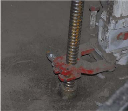
Figure 4.18 Drilling Bit with Welded Bit Teeth
