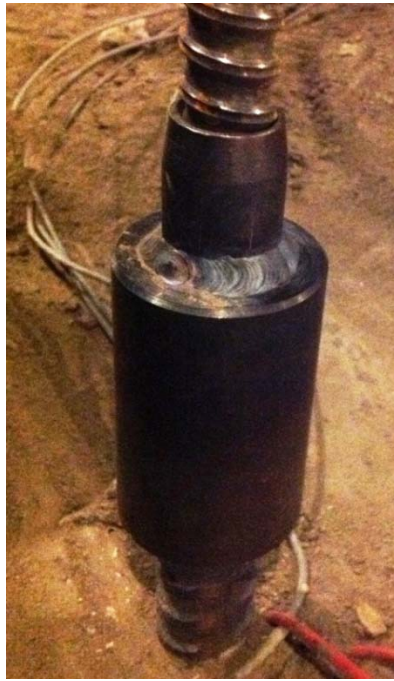
Figure 4.39 Anchor with Connecting Couple
