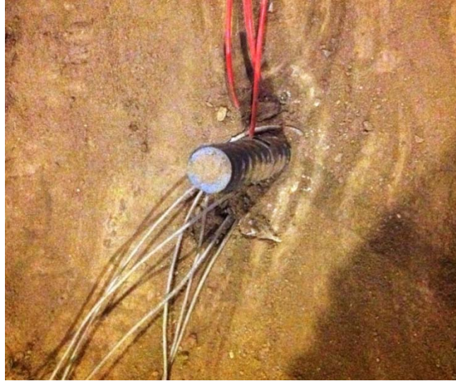
Figure 4.38 Cleaning Ground Surface
