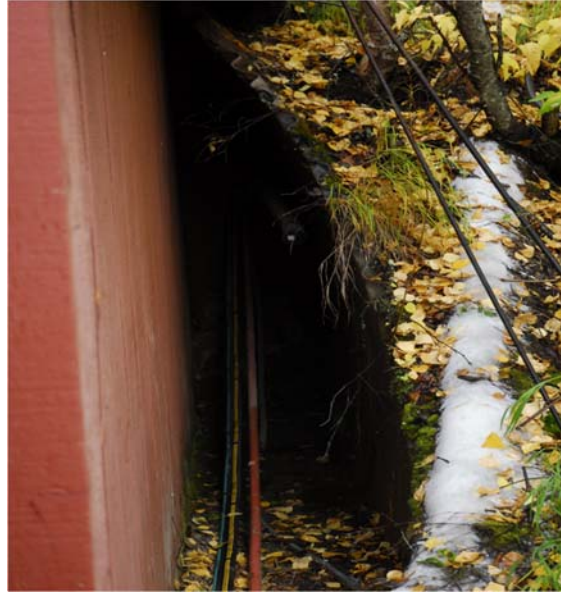
Figure 4.15 Open Hole for Hydraulic and Compressed Air Lines
