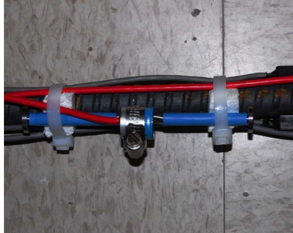
Figure 4.26 Geokon Vibrating Wire Strain Gage Installation
