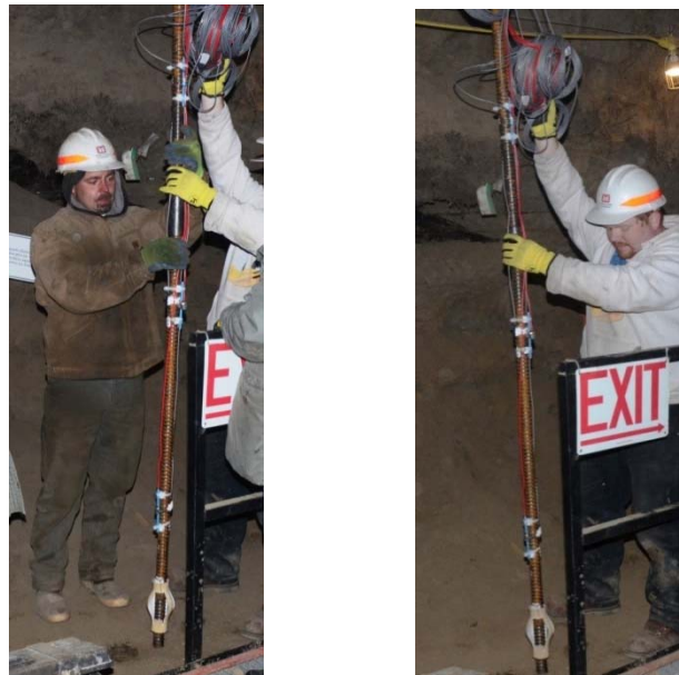
Figure 4.29 Anchor Installation Process
