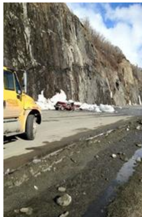
Photo: Seward Highway MP 113.2 crash caused by icefall April 6th, 2012.
