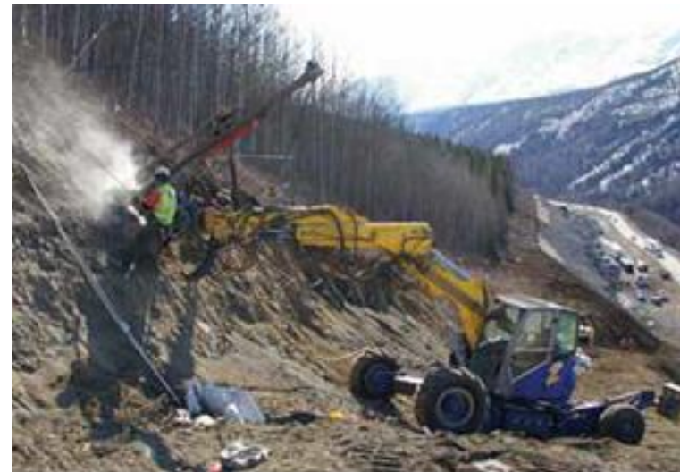
Drilling of the soil and rock slope on Glenn Highway Photo: Terry Barber
