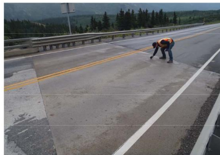
Bridge No. 1141 Br. Name Antler Creek Date 07/16/17 Inspector Murray / Knapp Frame 2 NE Approach Slab
