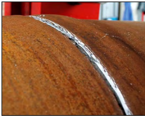
Figure 3-63: Rupture on top of the pile, ductility 4 pull 3, \Delta = 13 inches
