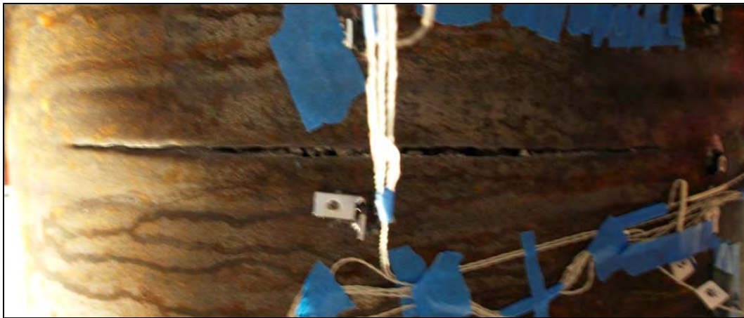
Figure 3-30: Rupture during the second push of ductility six, at a displacement of 12.5 inches
