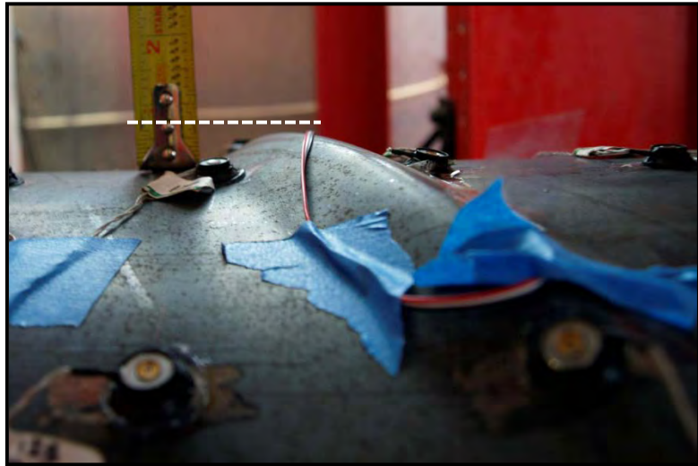
Figure 3-134: Buckle on top of pile in between loading points, ductility 3, \Delta = 8.4 in
