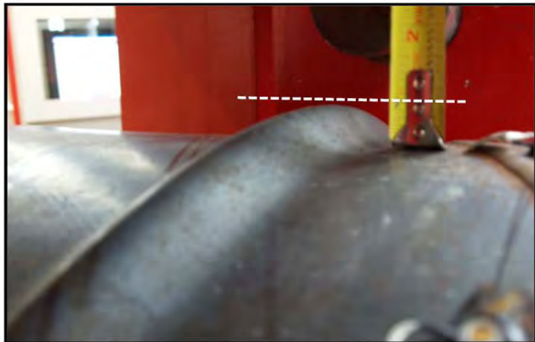
Figure 3-132: Buckle on top of pile under loading point, ductility 3, \Delta = 8.4 in
