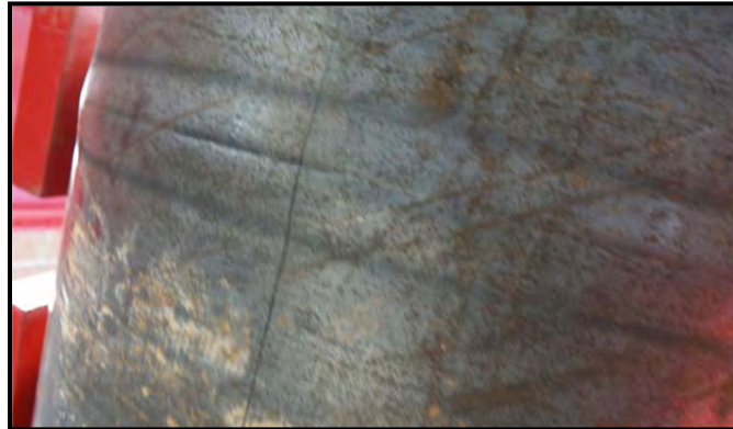
Figure 3-159: Crack on the underside of pile leading to the first push of ductility 5, \Delta=8.3 in
