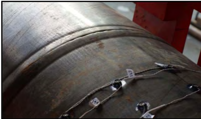
Figure 3-163: Rupture on top of the pile, first pull of ductility 5, \Delta=11.5 in
