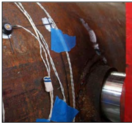
Figure 3-76: Initial rupture of the steel pipe during the first pull of ductility seven
