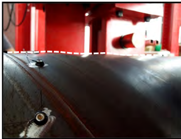
Figure 3-171: Ripples on steel pile, ductility 3 – 1st push, \Delta = 6.0 inches
