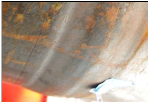
Figure 3-50: Tension cracks under the pile during the third push of ductility 5 ( \Delta=15 in)
