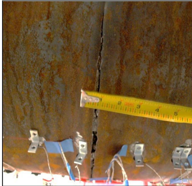
Figure 3-39: Rupture at ductility six, push three, displacement = 12 inches
