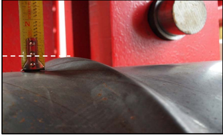
Figure 3-128: Buckle located under one of the loading points, ductility 2, \Delta=5.7 in
