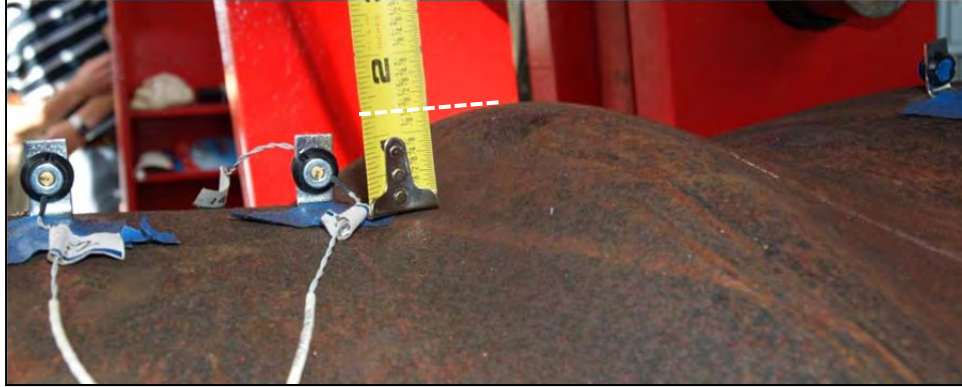
Figure 3-23: Buckling under north loading at ductility 5 push 2, at a displacement of 17.07 inches
