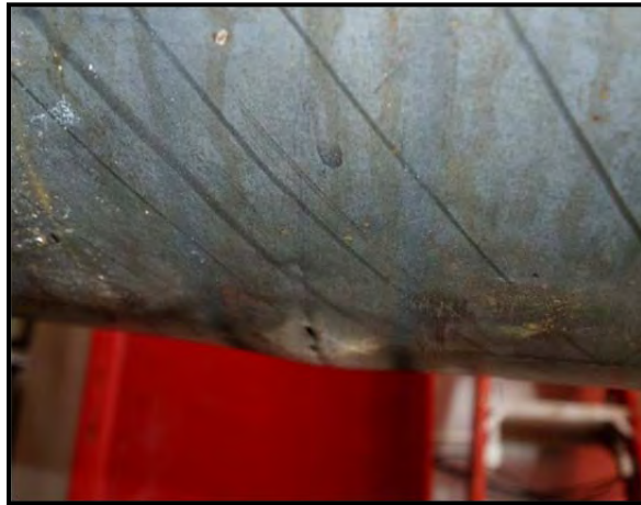
Figure 3-118: Steel pipe tensile crack, \Delta=8.40 in
