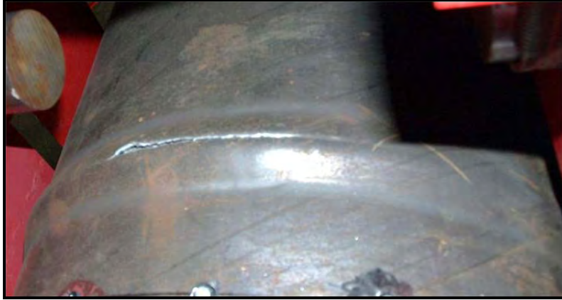
Figure 3-211: Second rupture under north loading point, en route ductility 6, \Delta=3.45 in
