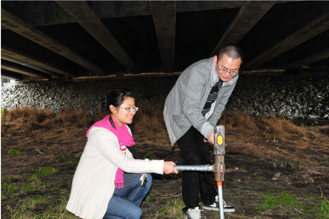
Figure 2.1 Installation of a temperature monitoring conduct at the Campbell Creek bridge site.
