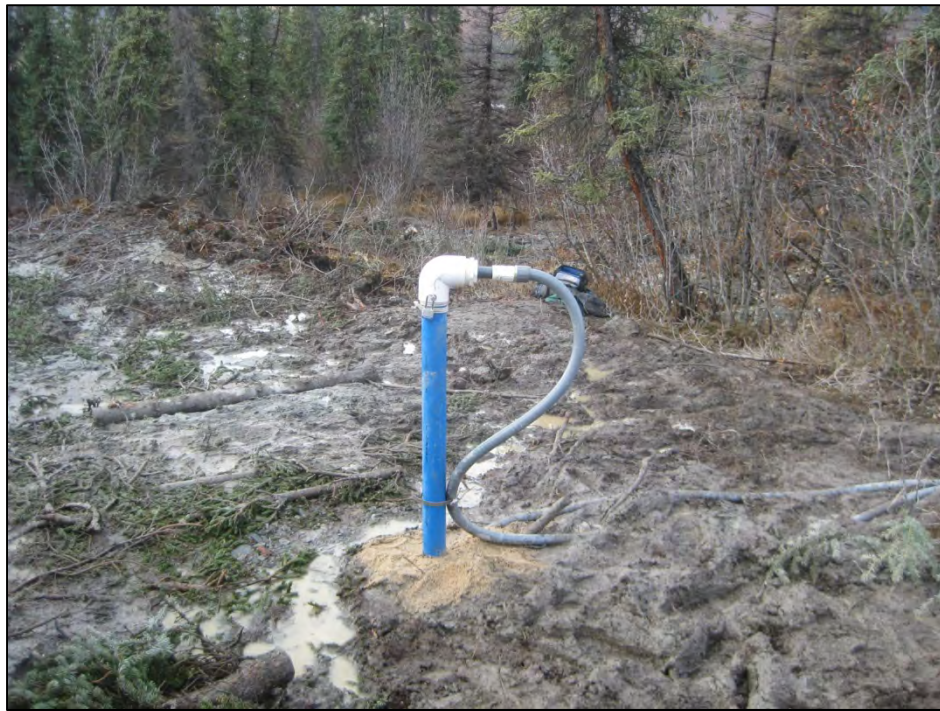
Figure B-8. Completed casing and instrument installation in TH12-9004. (Photograph by M. Darrow)
