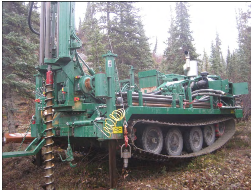
Figure B-1. Typical rig set-up for hollow-stem auger, with the CME 850X track-mounted drill. Photograph taken while drilling TH12-9000. (Photograph by M. Darrow)
