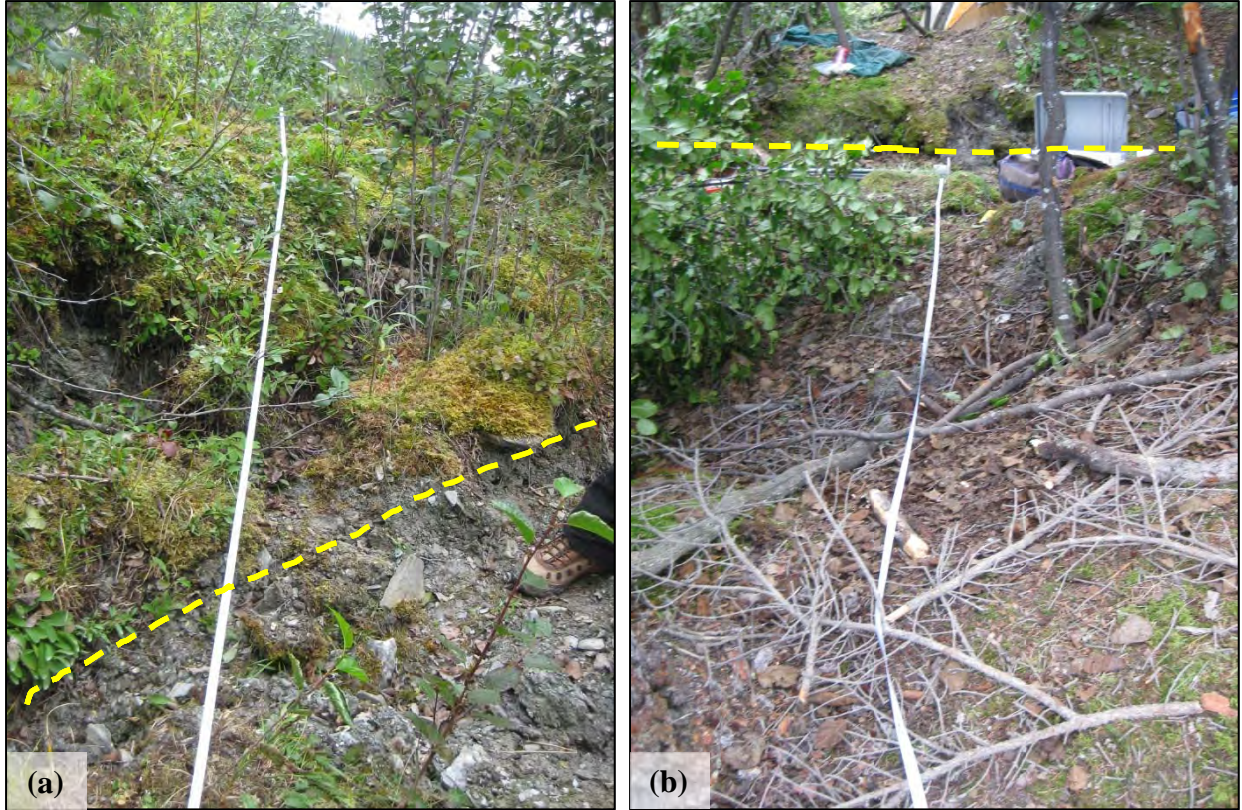
Figure A-1. Cracks (indicated by dashed yellow lines) along seismic Line 1 on FDL-A. (a) Crack between Shots 2 and 3; photograph was taken towards the south, facing the left-flank of FDL-A (photograph by M. Darrow); (b) crack between Shots 11 and 12; photograph was taken towards the south. (Photograph by J. Simpson)
