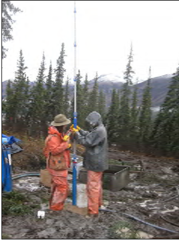
Figure B-7. Installing the MEMS-based in-place inclinometer (M-IPI) within the slotted casing in TH12-9004. (Photograph by J. Simpson)
