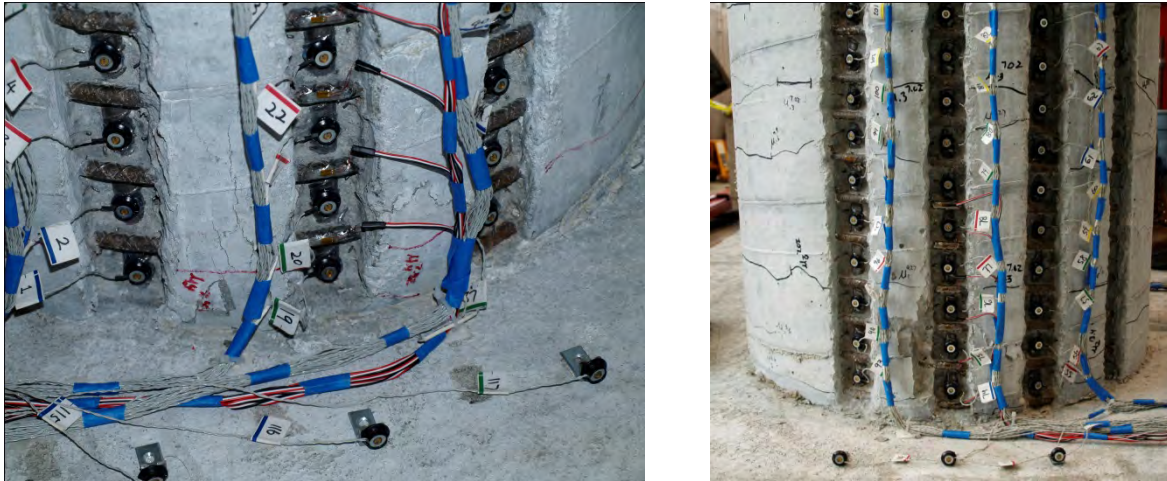
Figure 2-77. Test 10 – (Left) Concrete Crushing of South Side of the Column during ( \mu_{2.0}^{13.40 \text{ sec}} = 1.70'' ) and (Right) Crushing of North Side during ( \mu_{-1.7}^{13.72 \text{ sec}} = -1.39'' )
