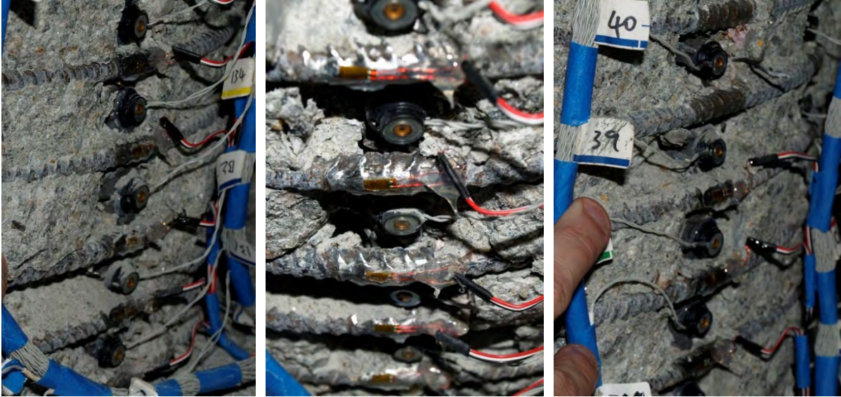
Figure 2-315. Test 17 – (Left) Additional Deformation in Buckled Bar N3 during ( \mu_6^{-3} = -5.00'' ), (Middle) Permanent Deformation in Spiral Layers over Buckled Region of Bar N3 during ( \mu_6^{+4} = 5.00'' ), and (Right) Additional Deformation in Buckled Bar S3 during ( \mu_6^{+4} = 5.00'' )
