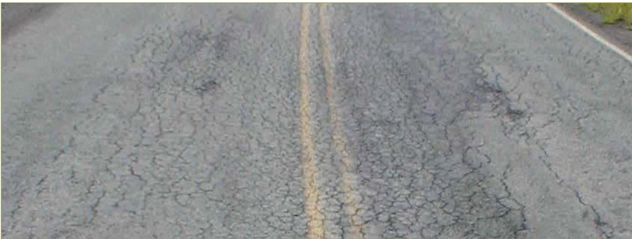
Figure 3–34. Alligator cracking
