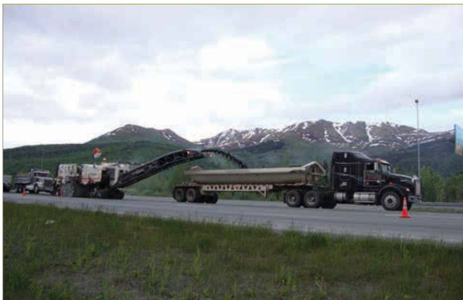
Figure 3–49. General milling operations
