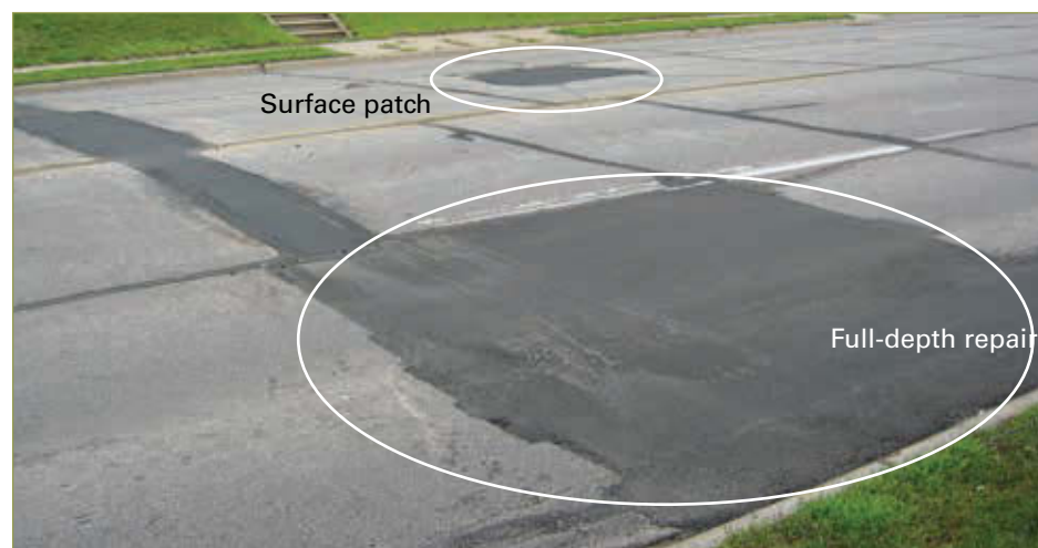
Figure 3–39. Surface patch and full-depth repair (CCEE/ISU)
