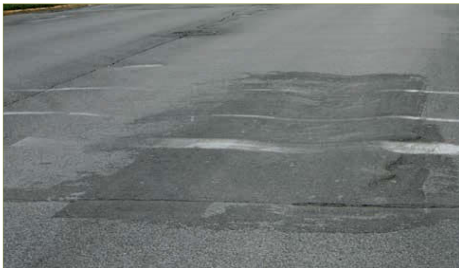
Figure 3–30. Rutting on an asphalt street
