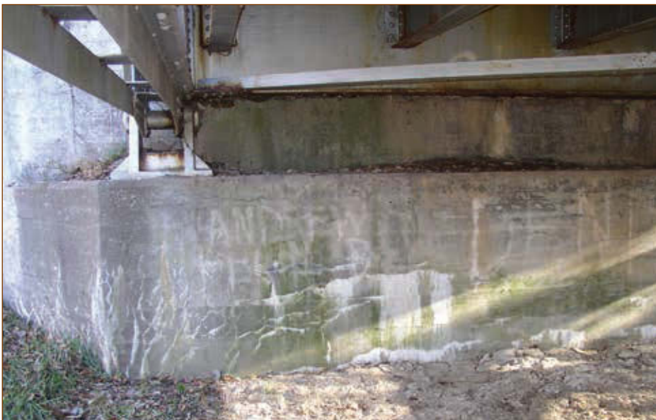
Figure 6–10. Abutments, bearings, and backwall with erosion and corrosion problems (Lee Co.)
