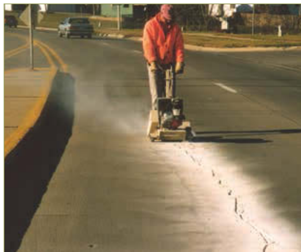
Figure 3–60. Routing cracks (WDM)
