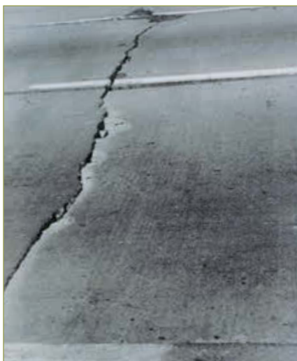
Figure 3-57. Faulting (FHWA)
