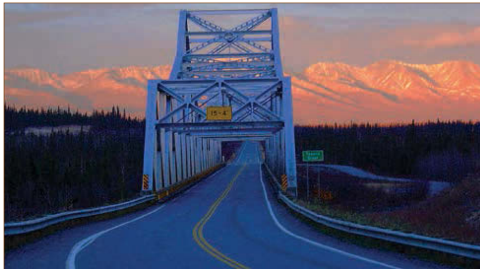
Figure 6-4. Visible object markers at a bridge
