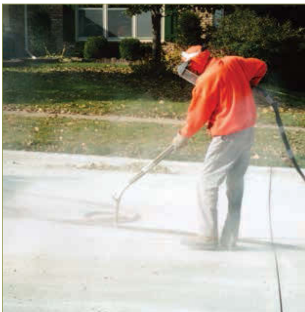
Figure 3–61. Cleaning joints before applying sealant (WDM)
