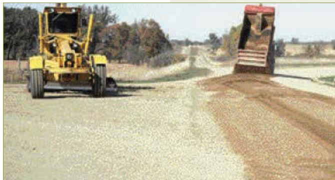
Figure 3–22. Placing new material on roadway (optional) (LTAP-SD)
