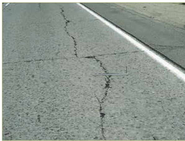
Figure 3-52. High-severity longitudinal cracks (FHWA)
