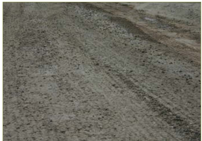
Figure 3–28. Adequate moisture for applying dust control material
