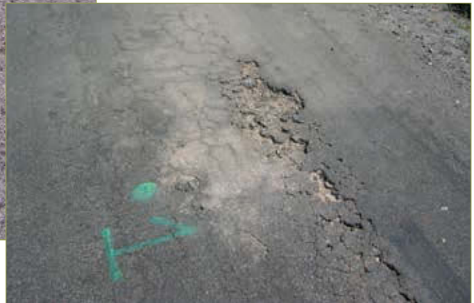
Figure 3–32. High-severity fatigue cracking (CCEE/ISU)
