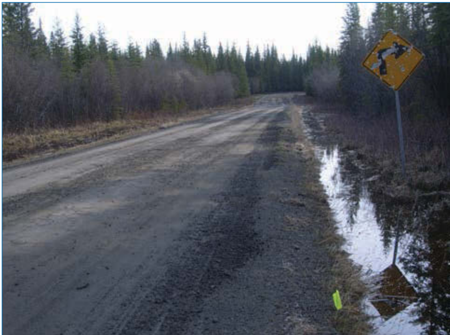
Figure 5–3. A flat ditch may not drain properly
