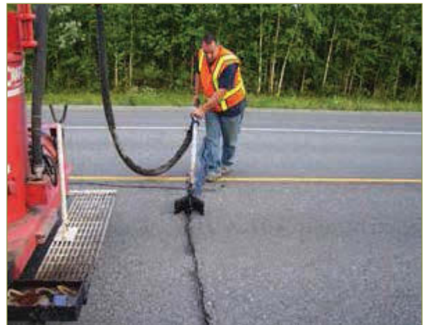
Figure 3–38. Crack sealing
