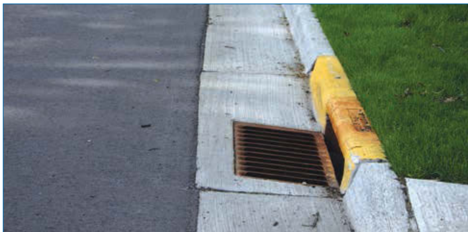
Figure 5–4. Water-tight joints at an inlet
