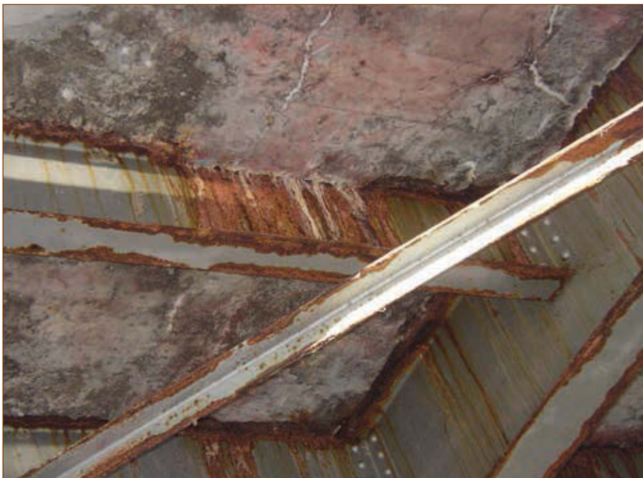
Figure 6–7. Evidence of deck seepage (Lee Co.)
