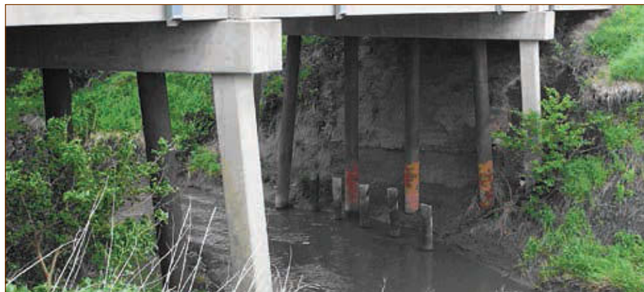
Figure 6–8. Erosion around base of piers (Ettema, et al.)
