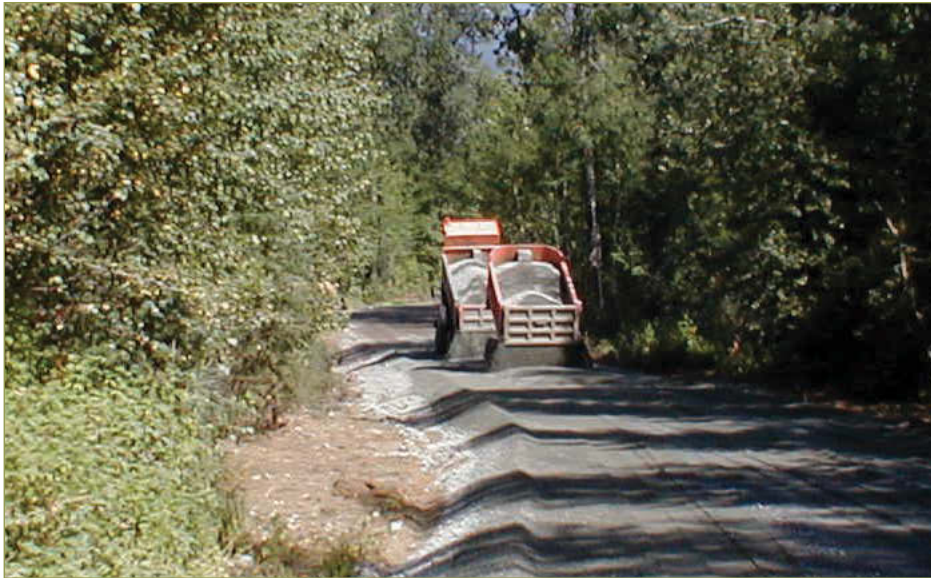
Figure 3–19. Placing new material on the roadway
