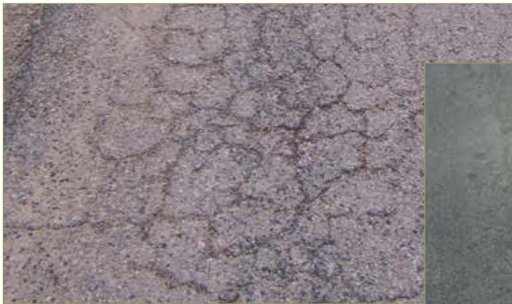
Figure 3–31. Fatigue cracking (CCEE/ISU)
