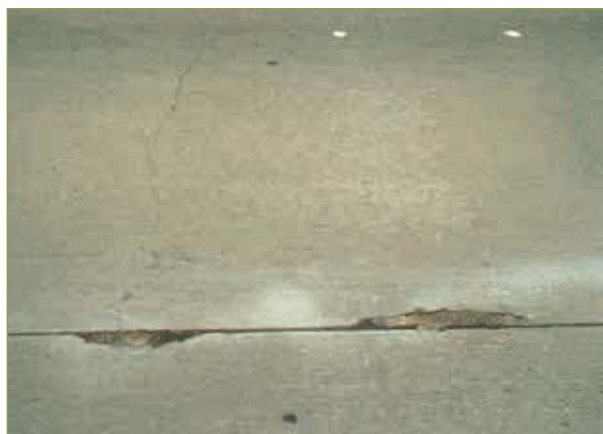
Figure 3–55. Spalling (FHWA)
