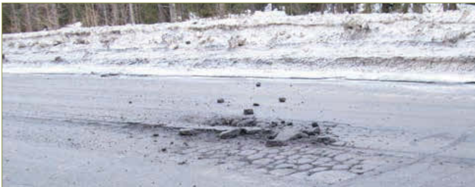
Figure 3–37. Pothole in asphalt pavement
