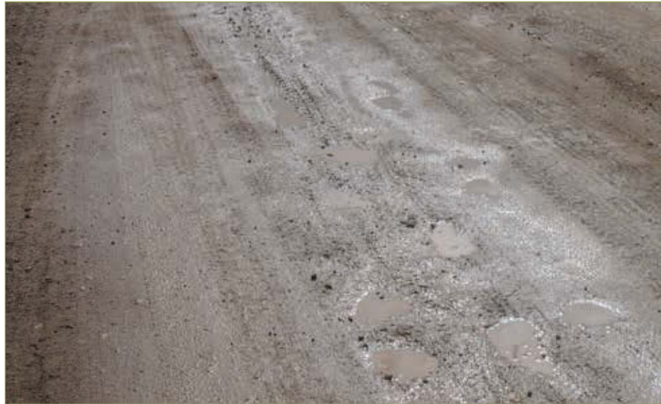
Figure 3-26. Potholes
