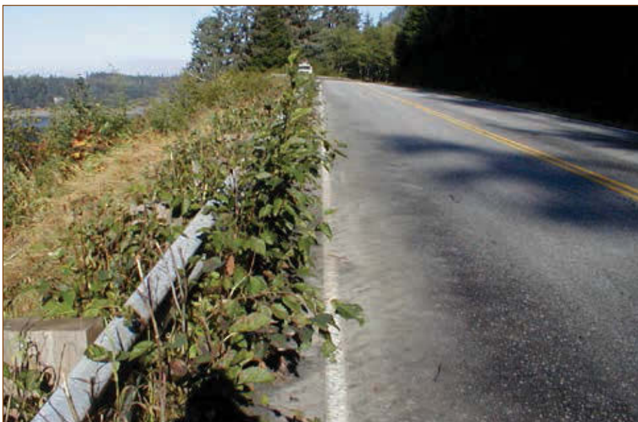
Figure 6–2. Overgrown vegetation at guardrail
