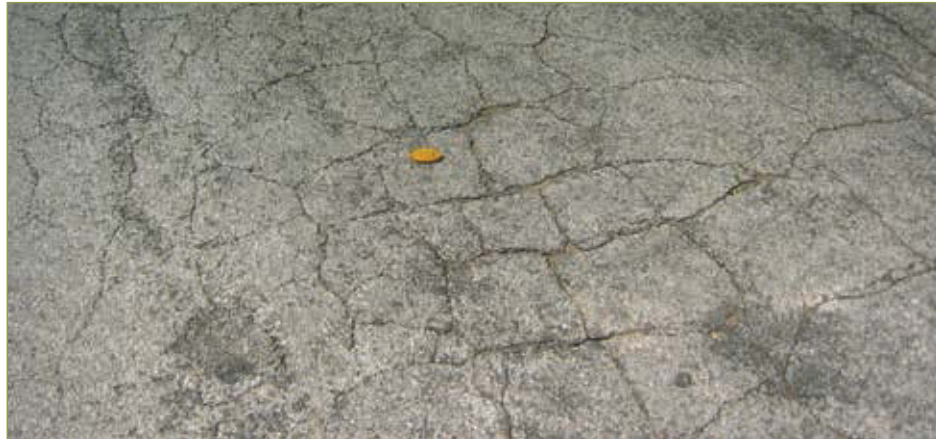
Figure 3–33. Block cracking (CCEE/ISU)
