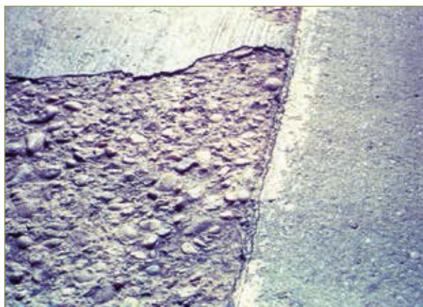
Figure 3–56. Scaling (FHWA)
