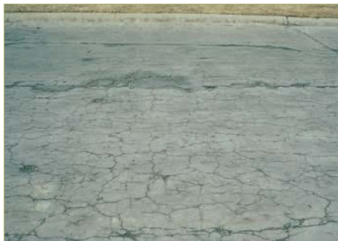
Figure 3-54. Map cracking (FHWA)
