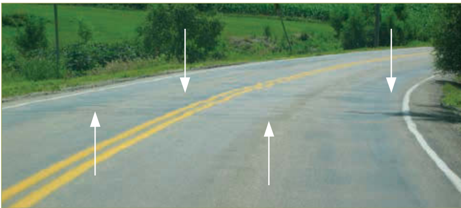
Figure 3–36. Washboards (CCEE/ISU)
