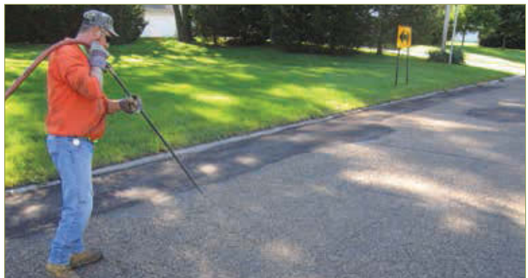
Figure 3–45. Cleaning the existing pavement surface (CCEE-ISU)
