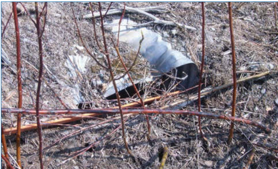
Figure 5–8. Debris accumulation at culvert
