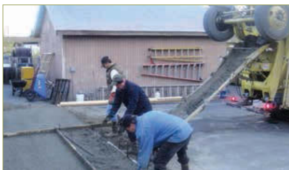
Figure 3-66. Placing concrete
