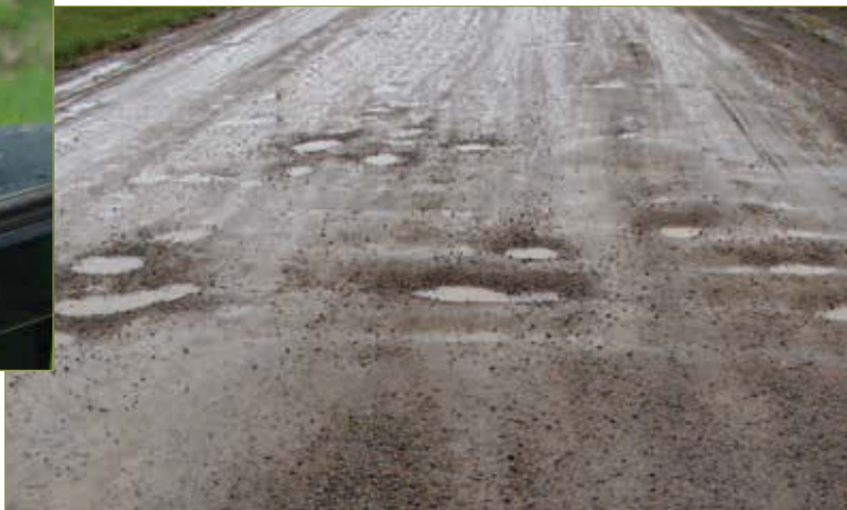
Figure 3–6. Poor crown shape
