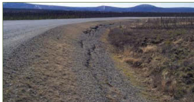
Figure 4-6. Erosion of the foreslope should be repaired before it becomes extreme
