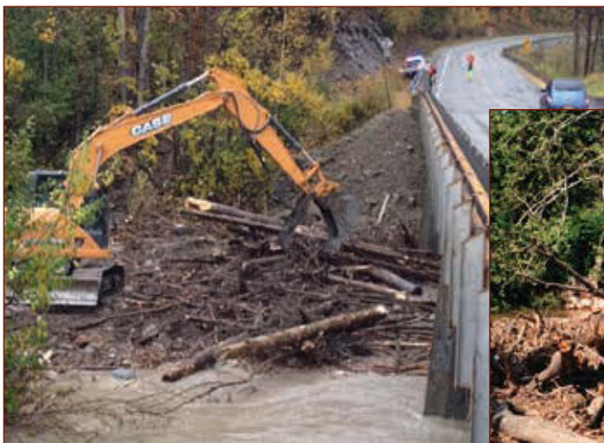
Figure 6–11. Debris collected around a pier
