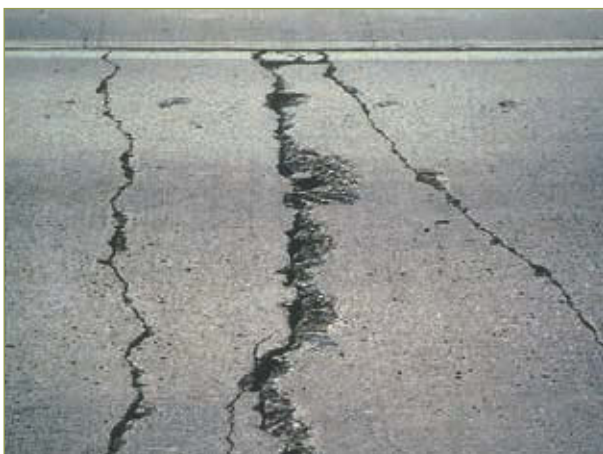
Figure 3-51. High-severity transverse cracks (FHWA)
