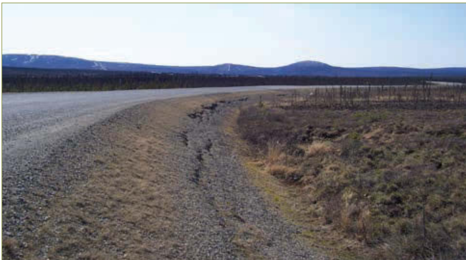
Figure 3–15. Slope slide from excess water
