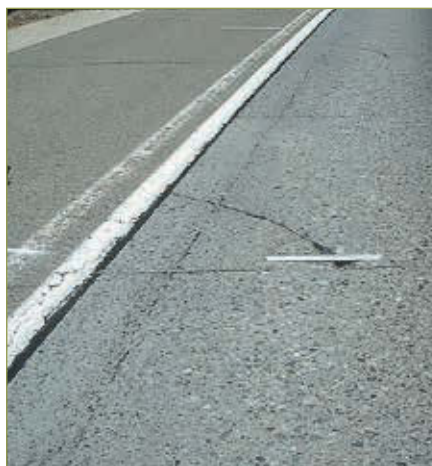
Figure 3-58. Corner break (FHWA)
