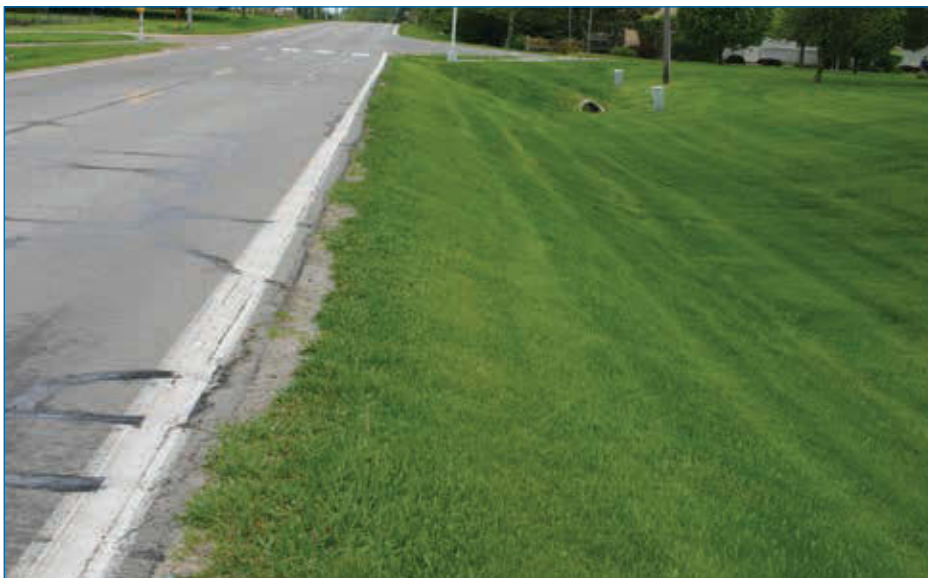
Figure 5–1. Ditch with good drainage
