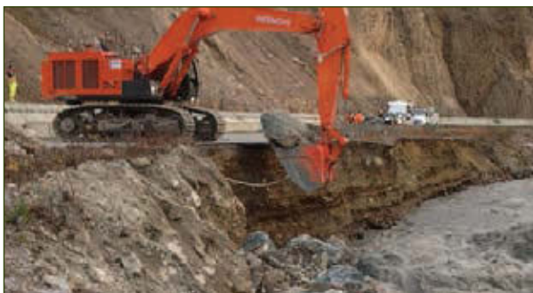
Figure 4-5. Erosion- slide repair of roadway embankment
