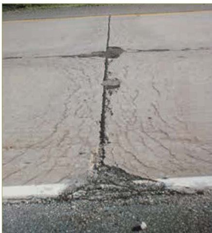
Figure 3-53. High-severity D cracks (FHWA)
