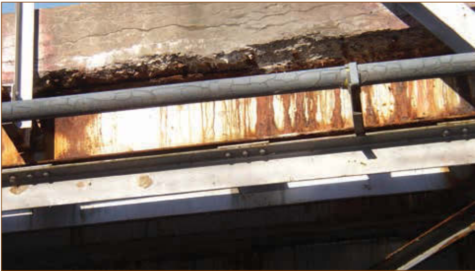
Figure 6–9. Corroded, discolored steel beams (Lee Co.)
