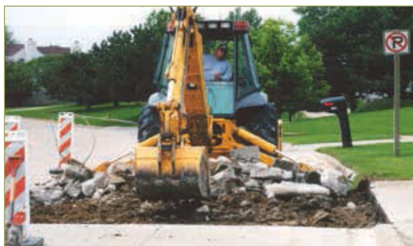
Figure 3-65. Removing full depth of slab (WDM)
