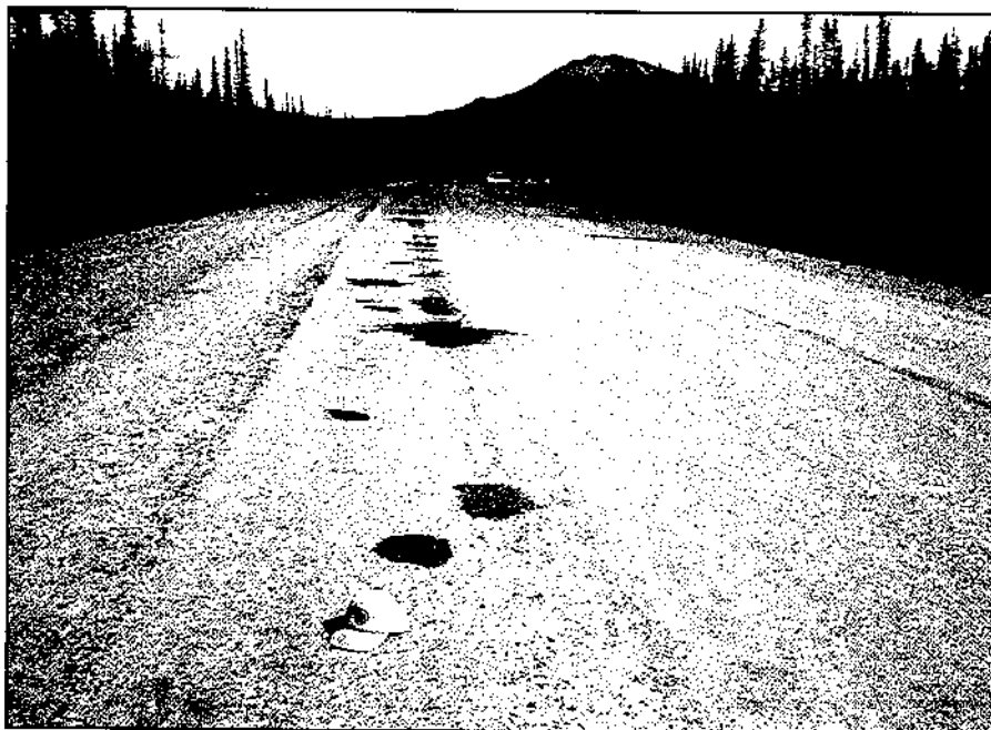
1995 Bituminous Surface Treatment failures at kilometer 1878 of the Alaska Highway. Pothole strings continued to develop for several weeks following application of BST. Potholing locations could not be associated with a single type of failure.
