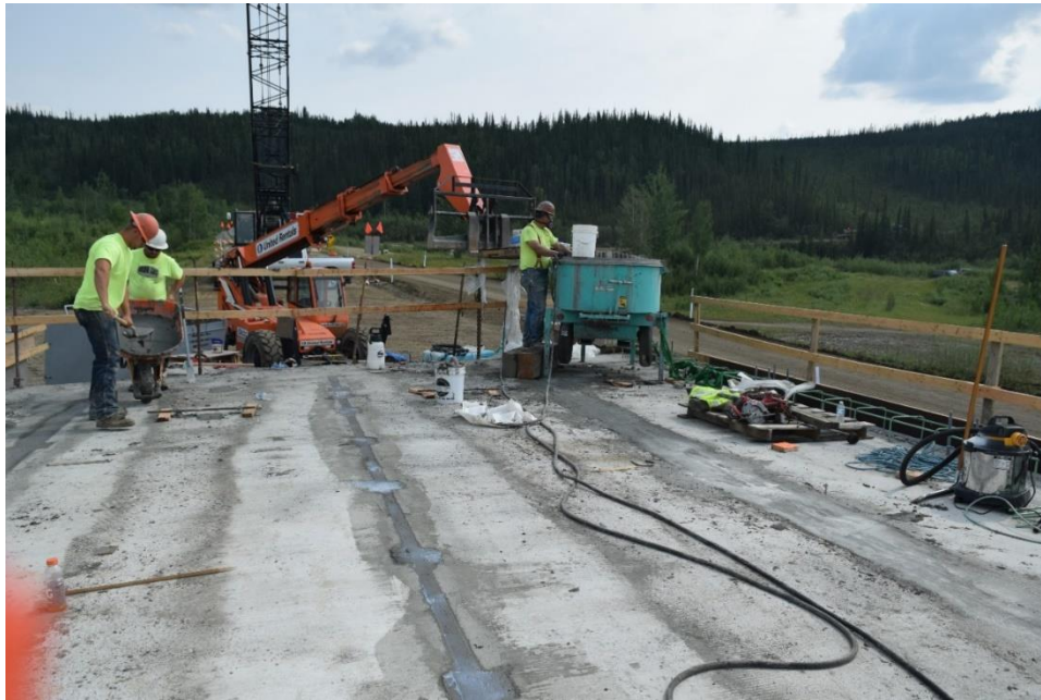
Figure G-2. Longitudinal keyways of the bridge
