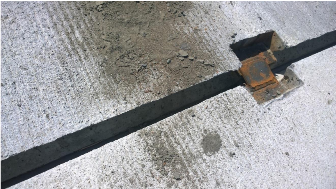
Figure G-12. Empty keyway just before grouting
