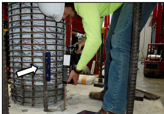
Figure 5.6: Installation of two-part epoxy into footing
