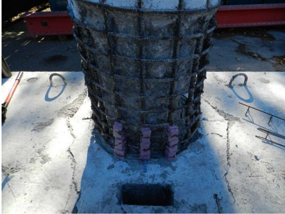
Figure 4.3: Foam Board to Bloc-out Grout on Straight Bars
