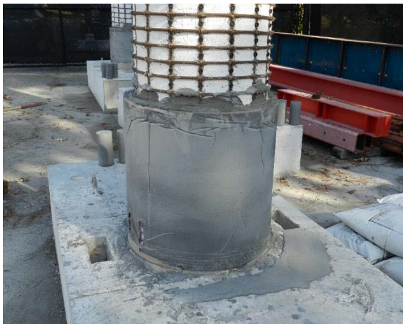
Figure 4.5: Restored Circular Concrete Section
