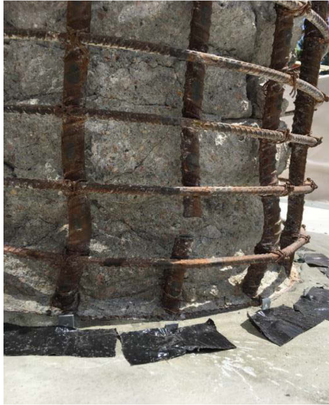
Figure 5.13: A Column after Removal of Loose Concrete
