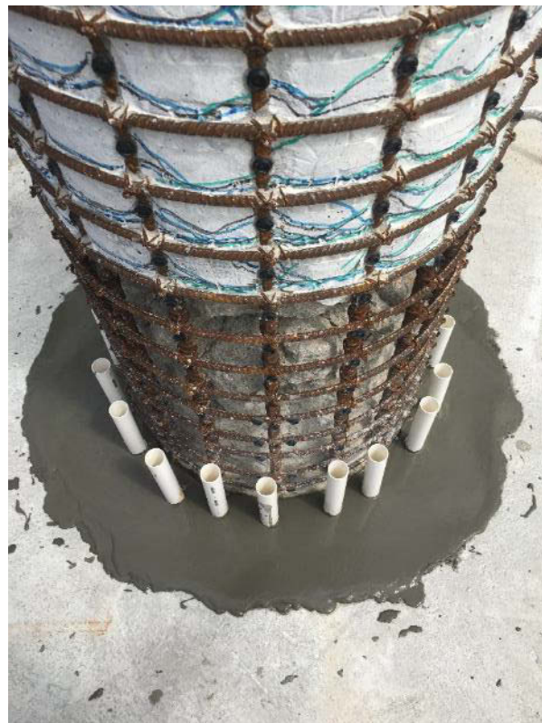
Figure 5.16: Restoration of Footing Cover Concrete with Grout
