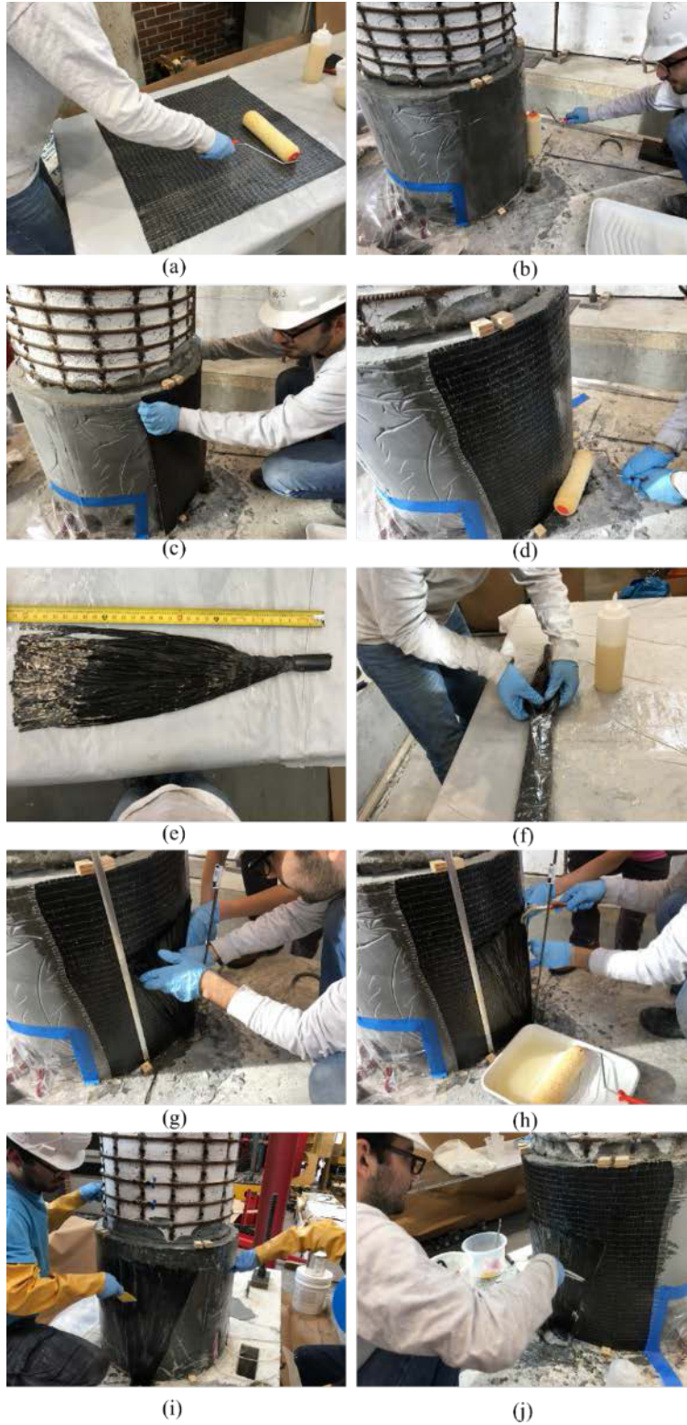
Figure 4.7: Anchor Preparation Process
