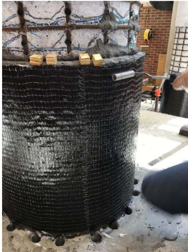
Figure 5.20: Air Removal with a Rib Roller
