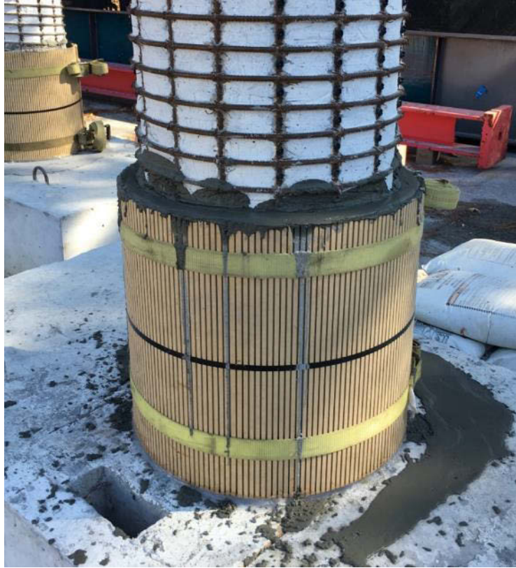
Figure 4.4: Form Work and High-Strength Grout
