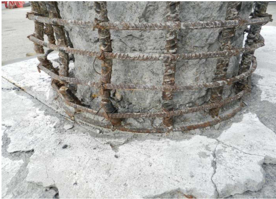
Figure 4.2: Removal and Cleaning of Loose Core Concrete
