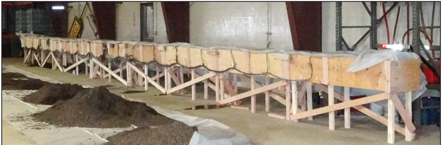
AUTC constructed a 73-foot long test flumes to evaluate the wicking effect of the fabric. All flumes were constructed on a level grade.
