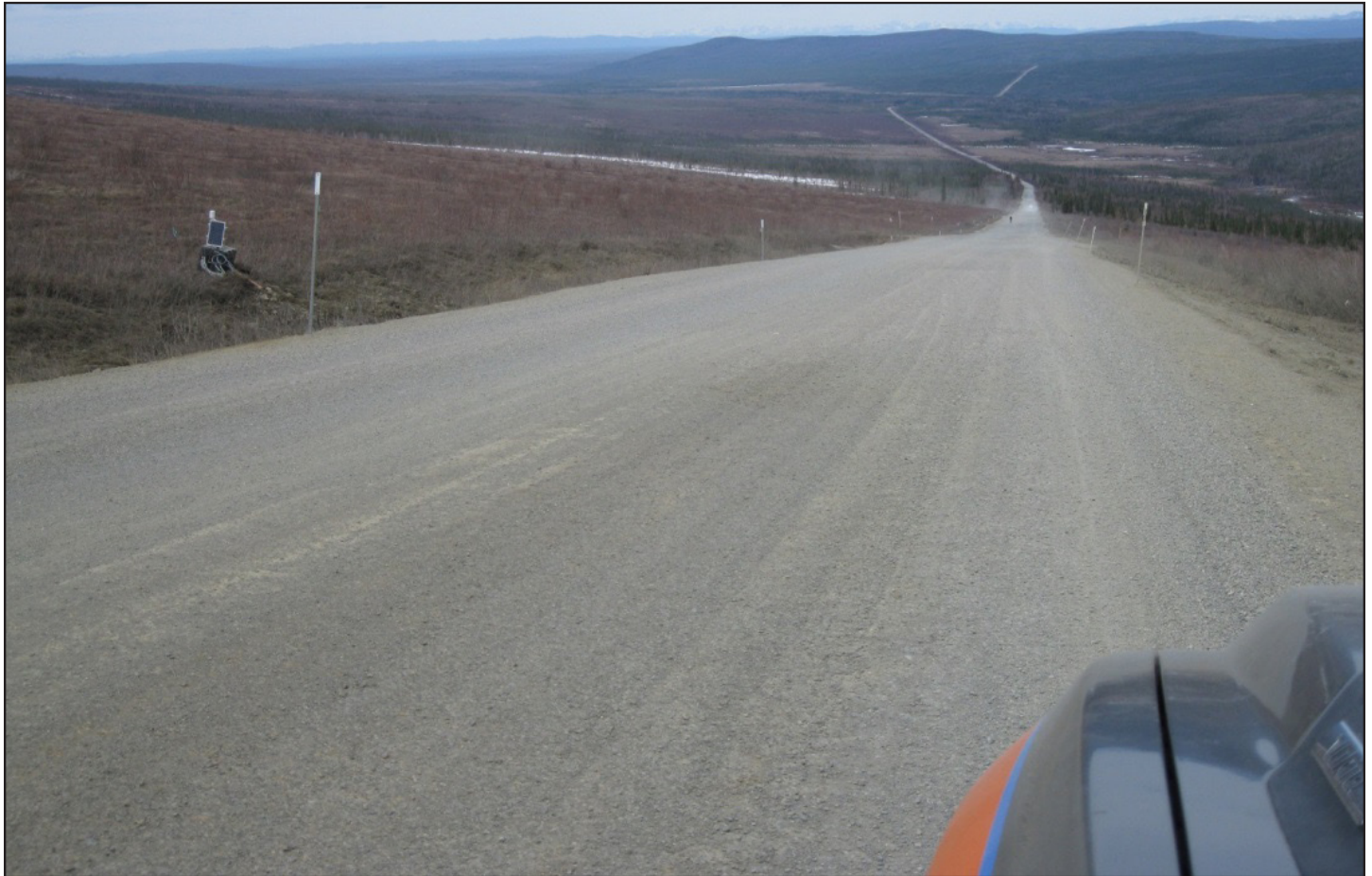
Milepost 110.5 on the Dalton Highway on May 24, 2011, after installation of H2Ri wicking fabric.
