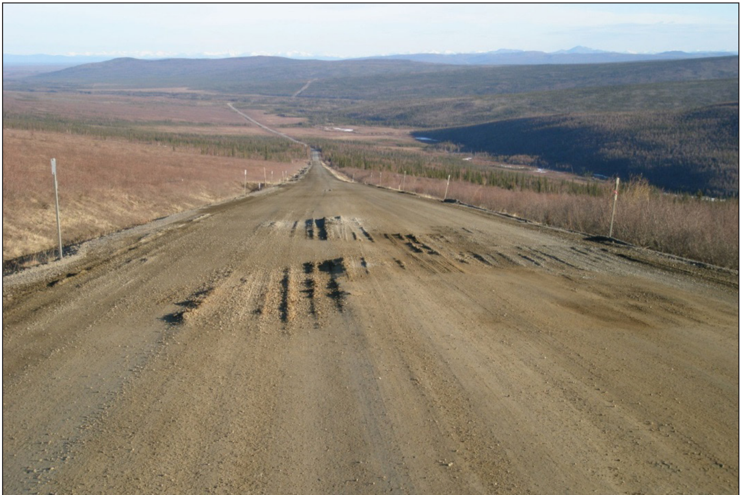
A problematic section of road known as the Beaver Slide at milepost 110.5 on the Dalton Highway, May 12, 2010.
