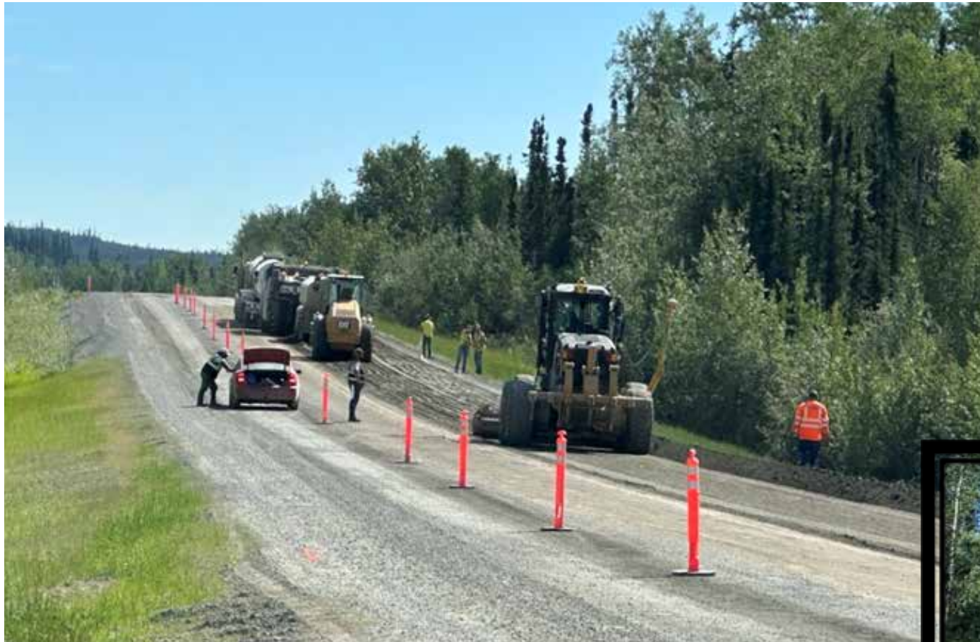
Foaming Train w/Motor Grader after the second pass commences
