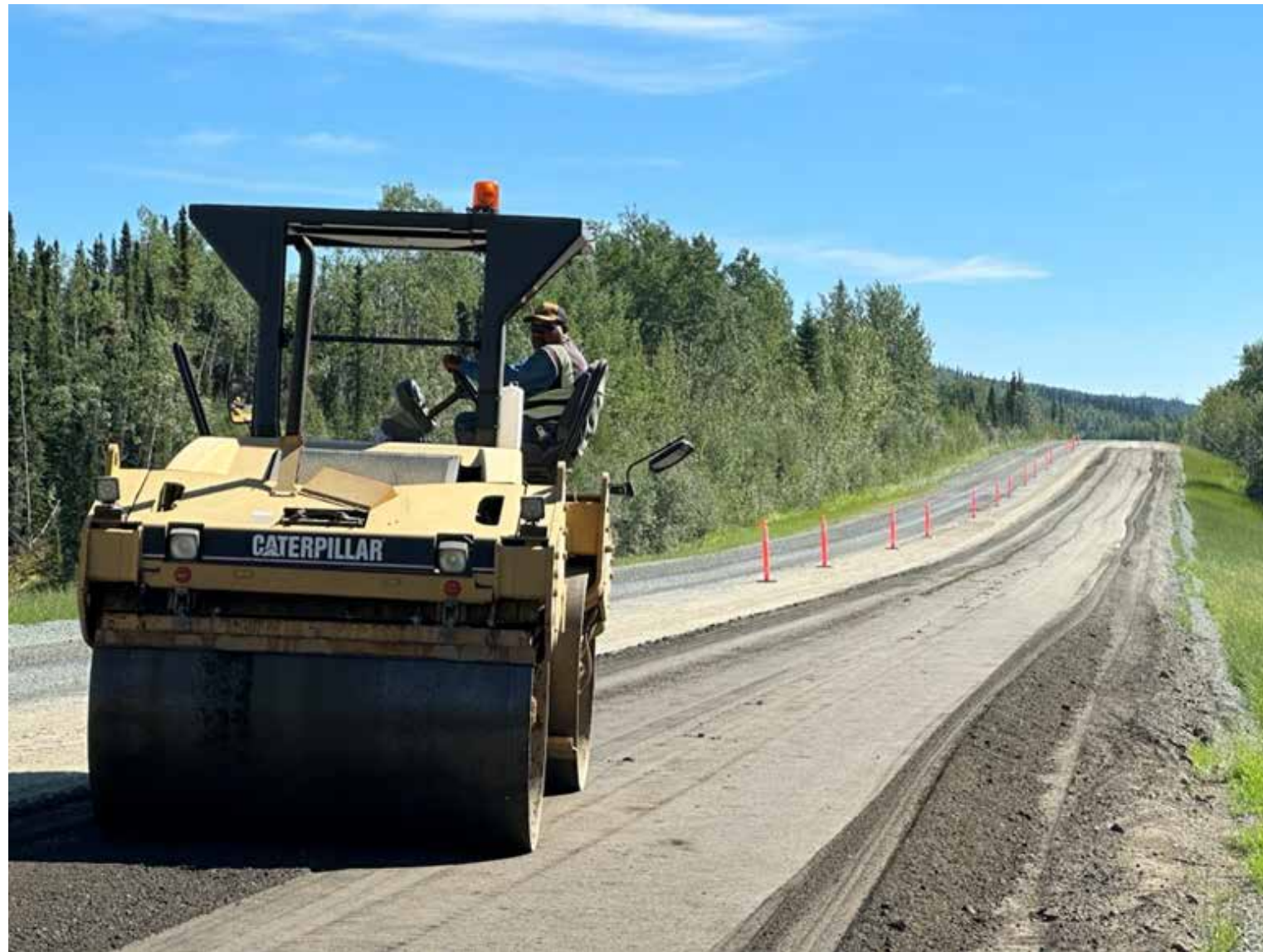
Double Vibe Steel Drums – secondary compaction after Motor Grader
