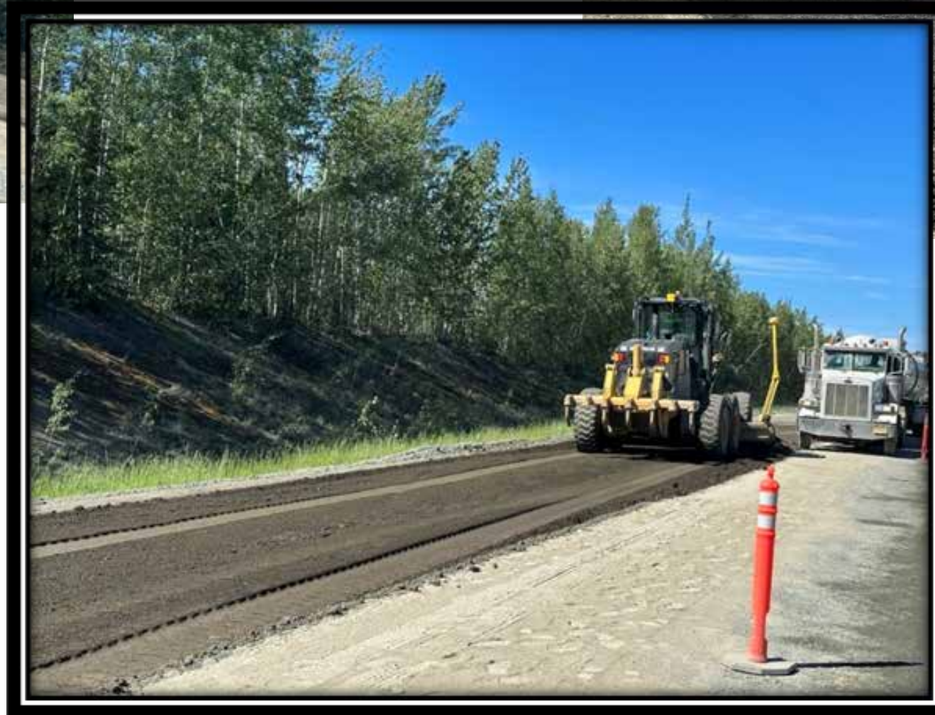
Second Water Truck working with Motor Grader
