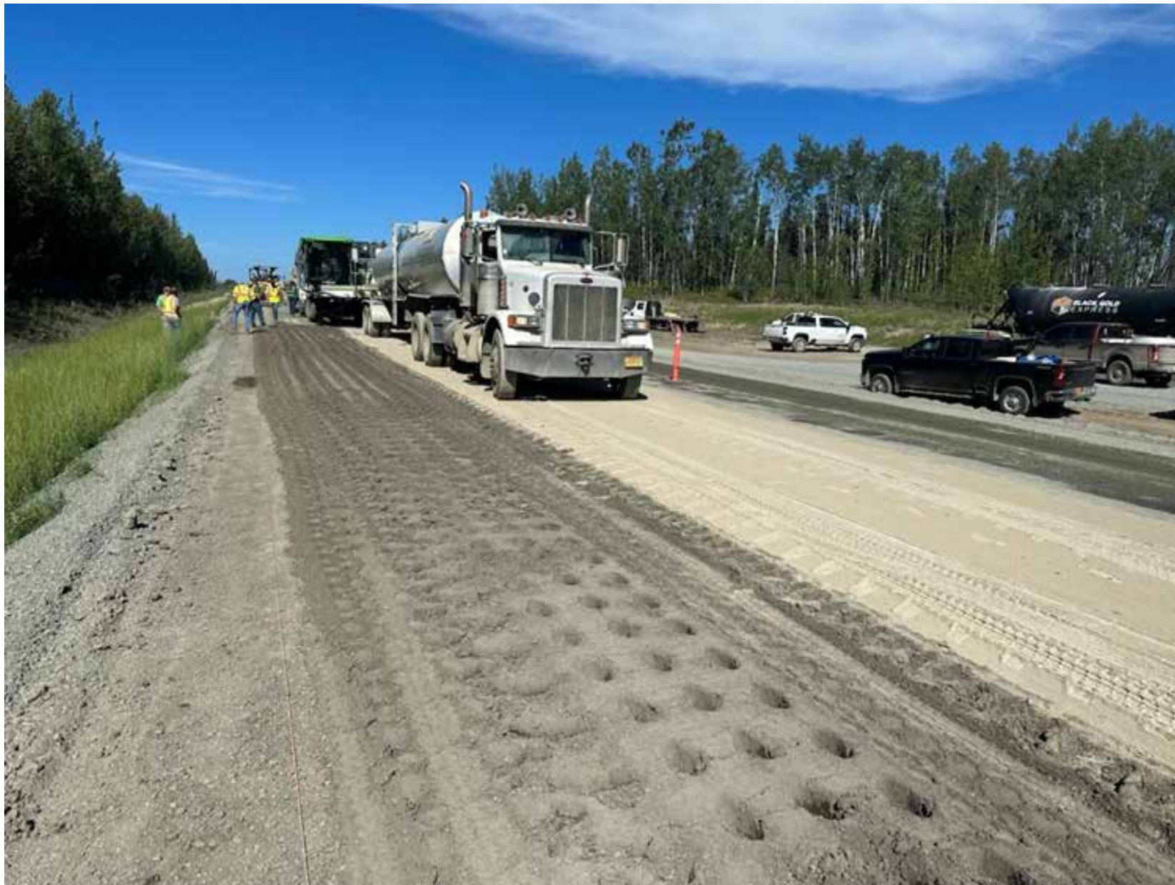
Foaming Train after Cement spread
