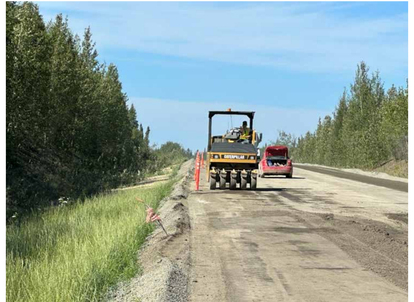
Pneumatic Tire Roller doing Finishing
