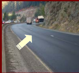
Streak – either down the center of the paved lane or either side of center.
