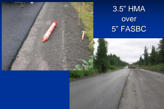
HMA paving - Seward Hwy MP 37-43
