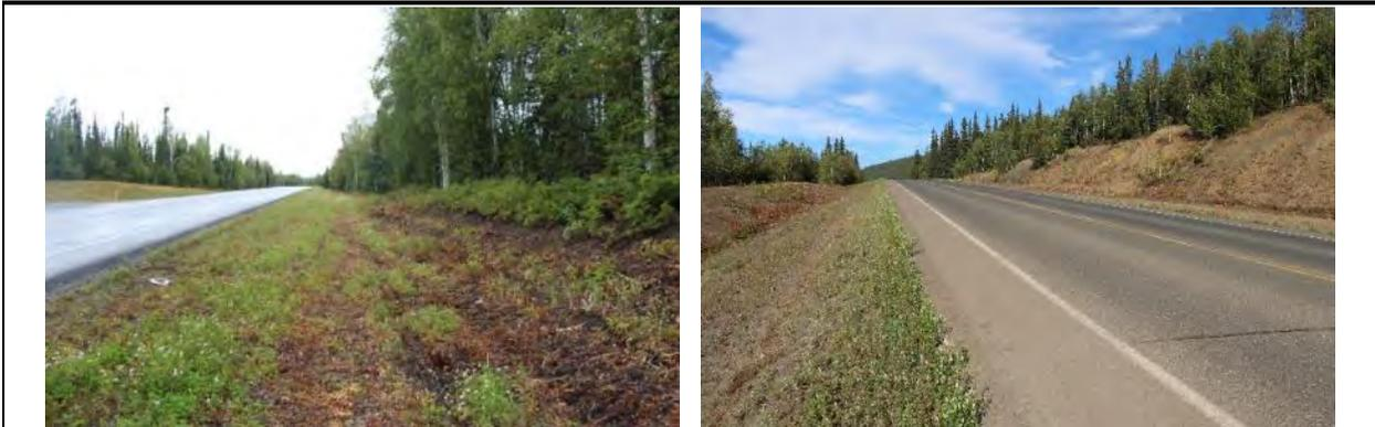
*Figures 10 (view facing southeast) and 11 (view facing northeast). Typical roadbed showing extent of wide embankment.*
