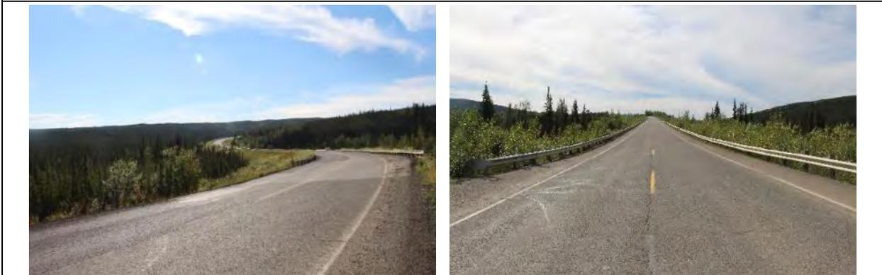
*Figures 12 (view facing east) and 13 (view facing north). Typical roadbed showing extent of elevated embankment due to borrow/fill.*
