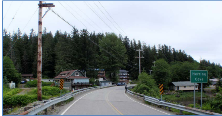
Figure 6. Herring Cove Bridge
