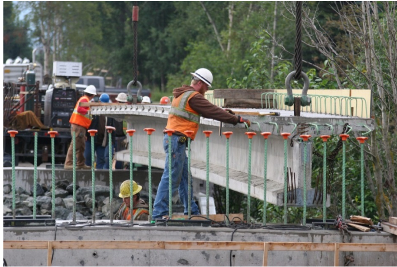
Figure 2 "Alaska-Style" Prestressed Girder Installation
