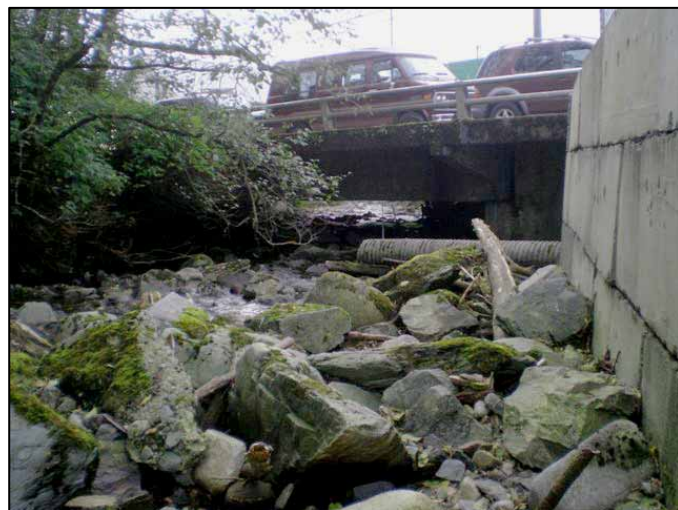
Figure 2. Hoadley Creek Bridge
