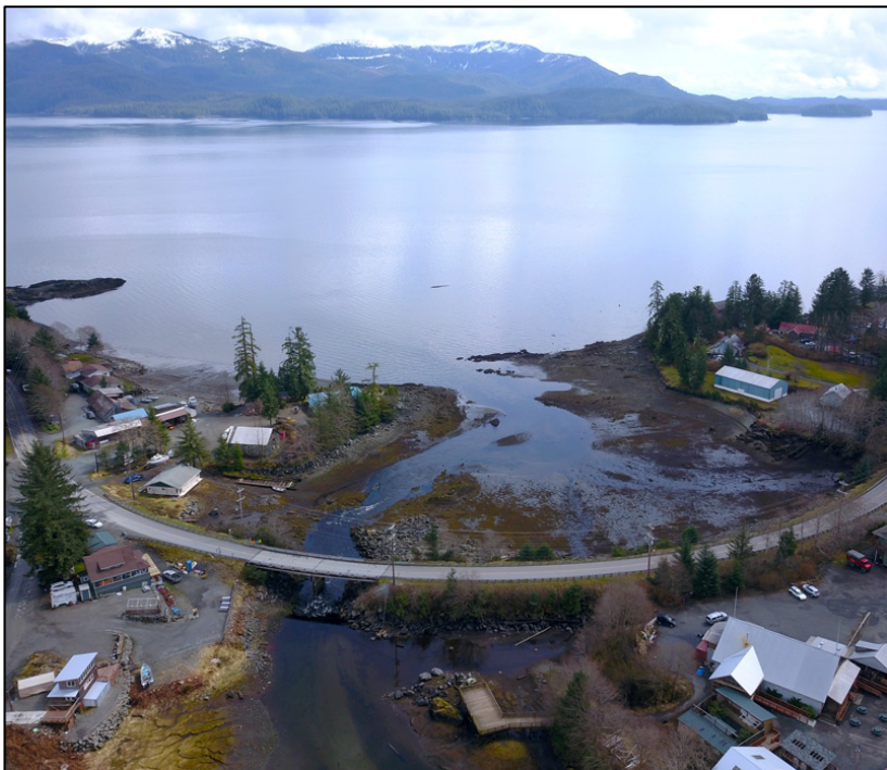
Figure 1. Herring Cove Bridge
