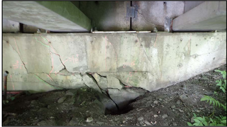
Figure 4. Ward Creek Bridge North Abutment Cap
