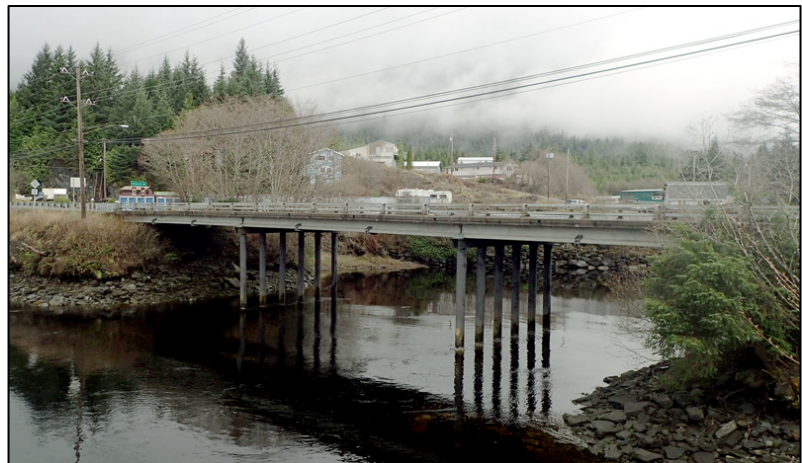
Figure 3. Ward Creek Bridge
