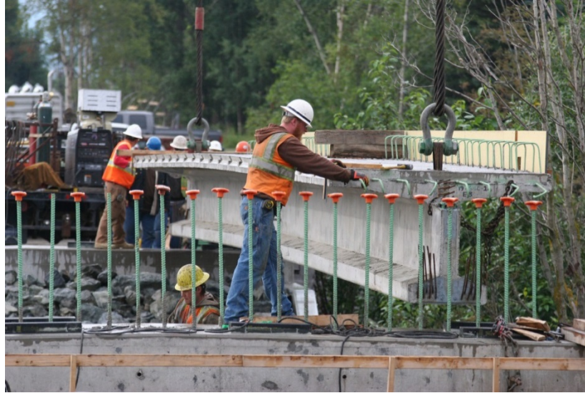
Figure 2 "Alaska-Style" Prestressed Girder Installation
