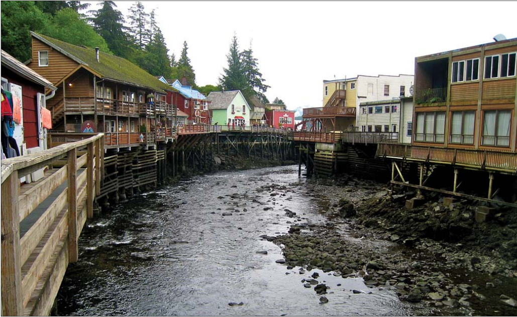
At left, Ketchikan Creek runs along historic Creek Street, a boardwalk on pilings. Photo by Jay Galvin
