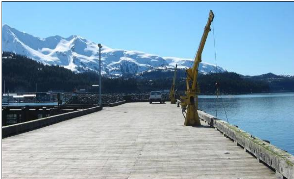
Figure 6.5.3: Timber Dock at Cordova.
