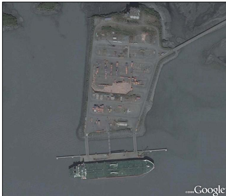
Figure 6.5.12: Valdez Container Terminal.
