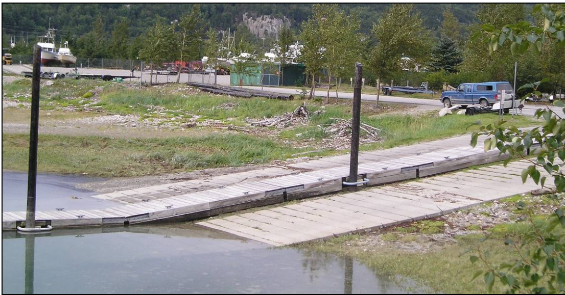
Figure 6.1.13: Launch ramp at Skagway small boat harbor.
