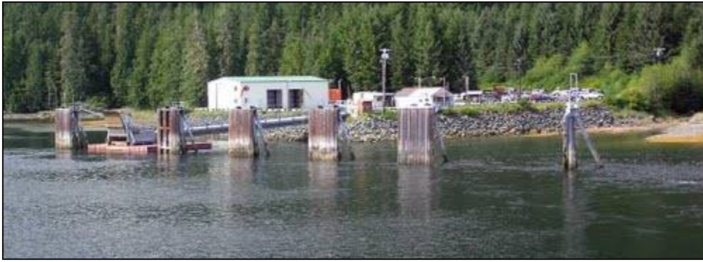
Figure 6.2.4: State Ferry landing facility at Hollis.
