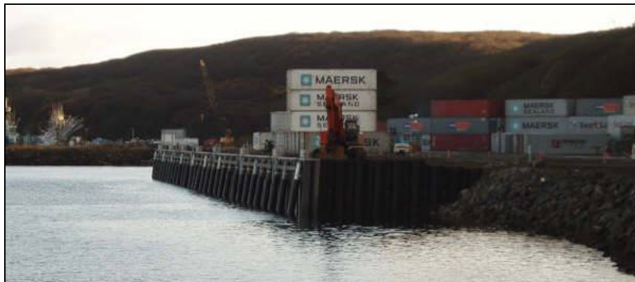
Figure 6.3.17: New sheetpile bulkhead wharf.
