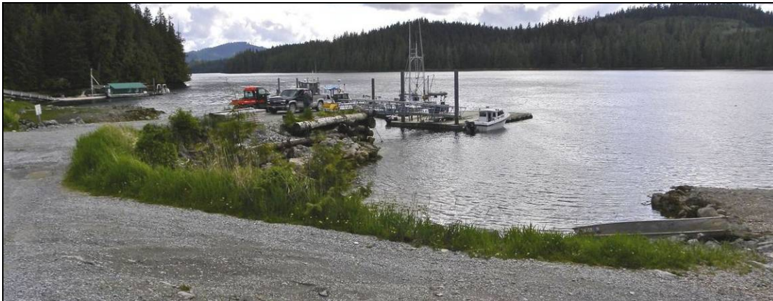
Figure 6.2.8: Waterfront Facilities at Naukati Bay.
