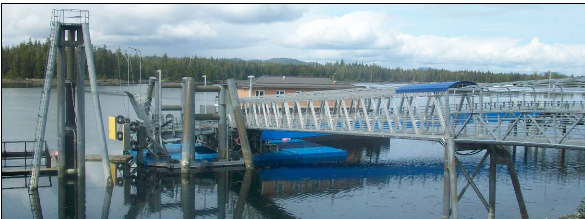
Figure 6.2.2: Coffman Cove ferry terminal.
