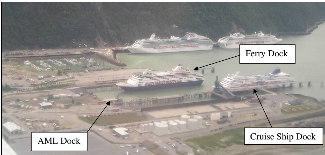
Figure 6.1.12: Skagway marine facilities.
