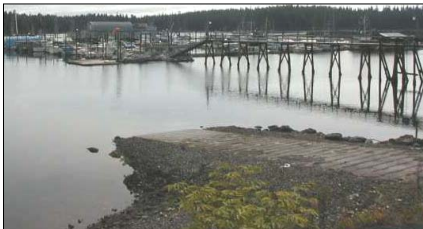
Figure 6.1.11: Kake's launch ramp landing, at the harbor in Portage Bay.
