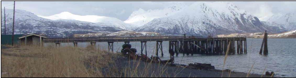
Figure 6.4.4: City Dock at Old Harbor.
