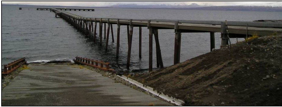
Figure 6.3.3: City dock and concrete ramp at Cold Bay.
