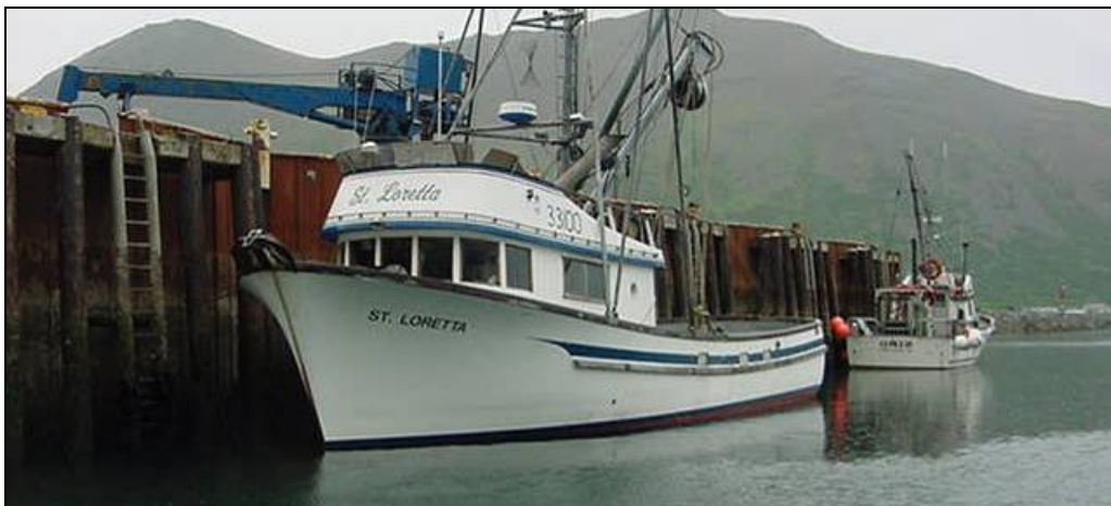
Figure 6.3.8: Sheetpile dock located in the King Cove old harbor area.
