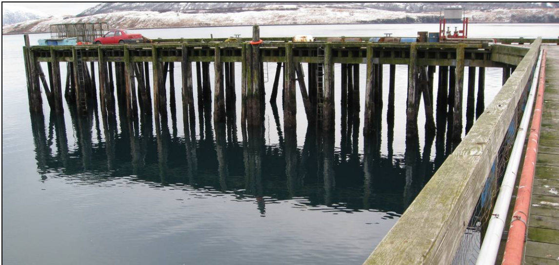
Figure 6.4.5: Fuel pipeline and header on City Dock at Old Harbor.
