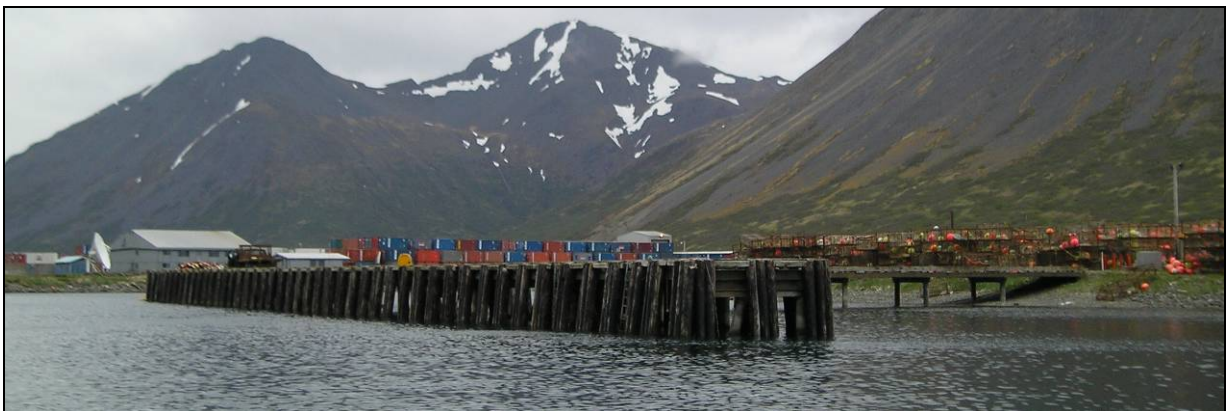
Figure 6.3.9: Timber dock located in the King Cove old harbor area.
