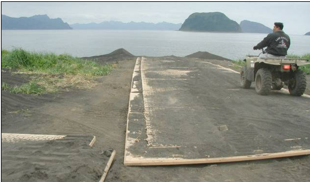
Figure 6.3.12.: Cargo Mats at Perryville barge unloading area.
