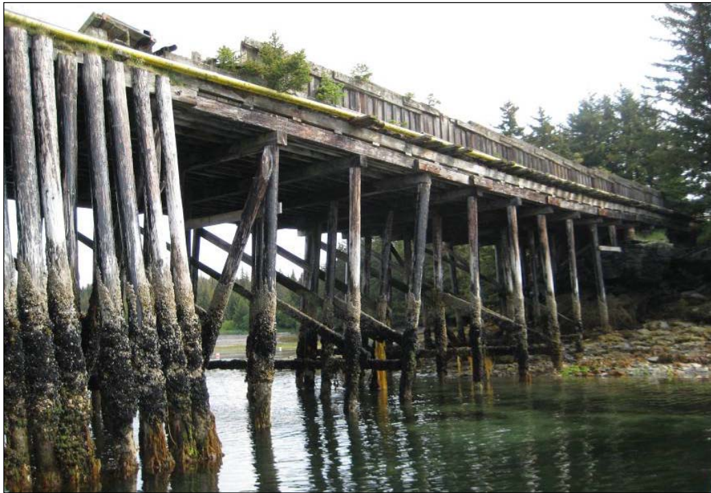
Figure 6.4.8.: Port Lions City Dock is aged and has reduced capacity.
