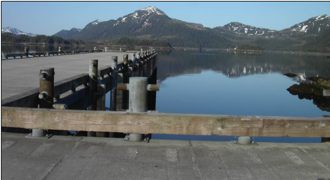
Figure 6.5.2: Existing Ferry Dock at Chenega Bay.
