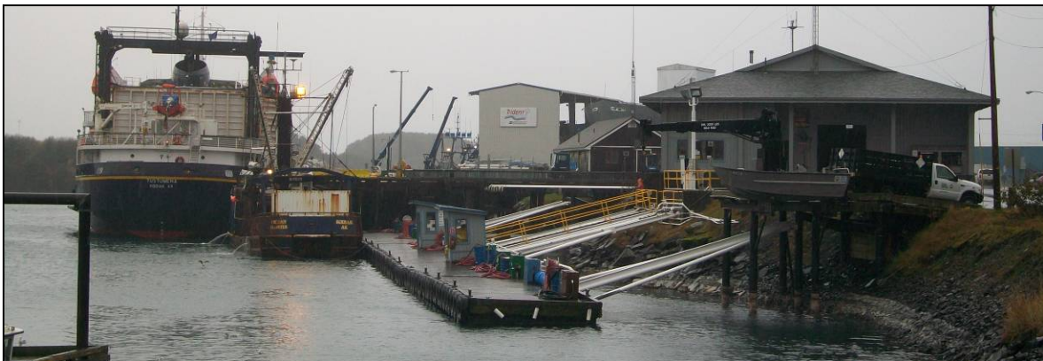
Figure 6.4.3: Ferry dock (background) and fuel float at Kodiak.
