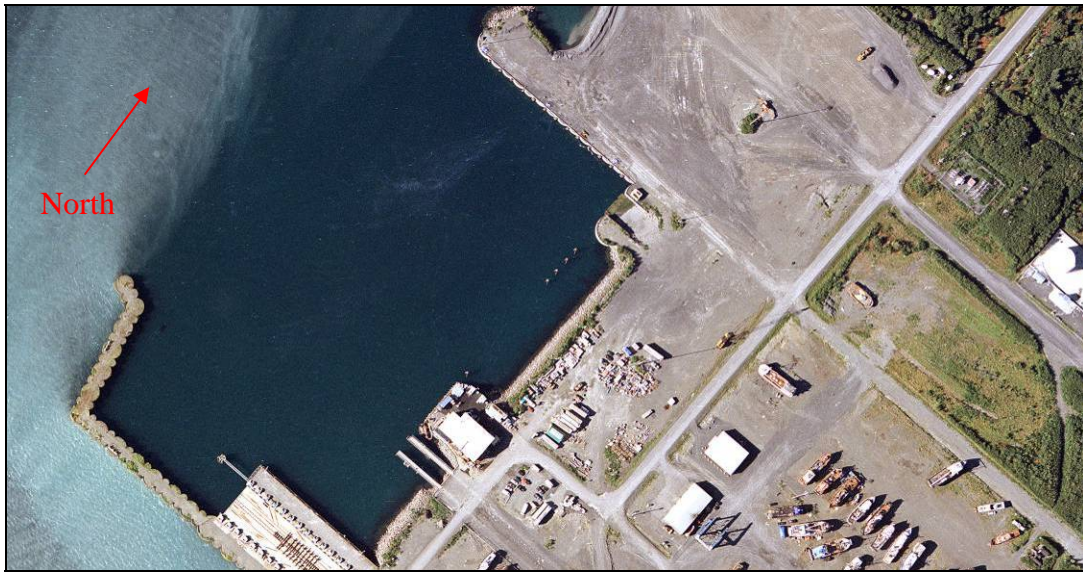
Figure 6.5.10: Seward Marine Industrial Center (©Aerometric, 2001).
