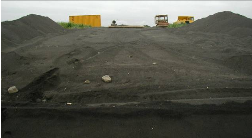
Figure 6.3.13: Freight barge landing area at Perryville, viewed from the water line.
