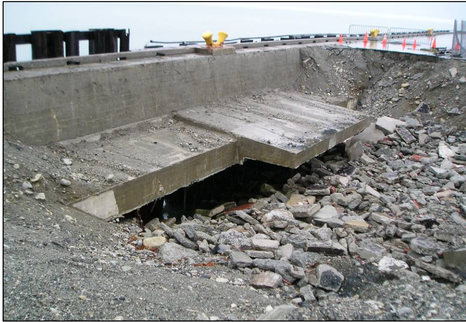
Figure 6.1.8: Areas of damage/subsidence at Lutak Dock.
