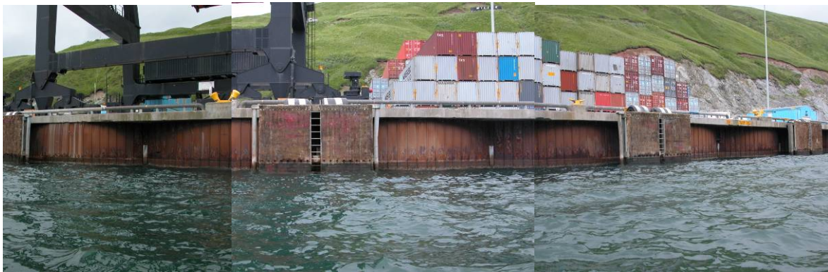
Figure 6.3.19: Unalaska Marine Center crane/freight unloading area.
