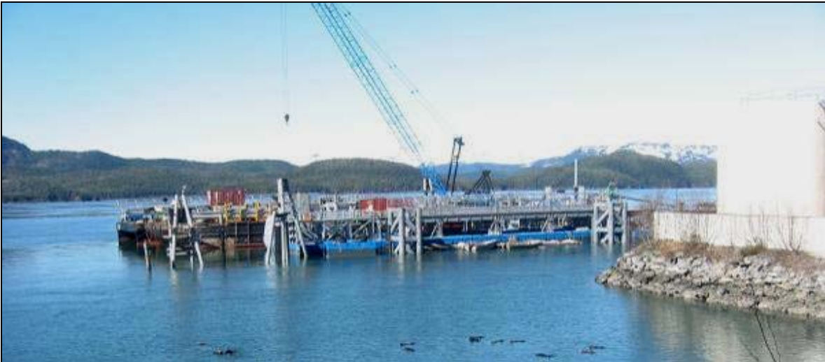
Figure 6.5.4: Ferry terminal at Cordova is used for offloading fuel and freight.
