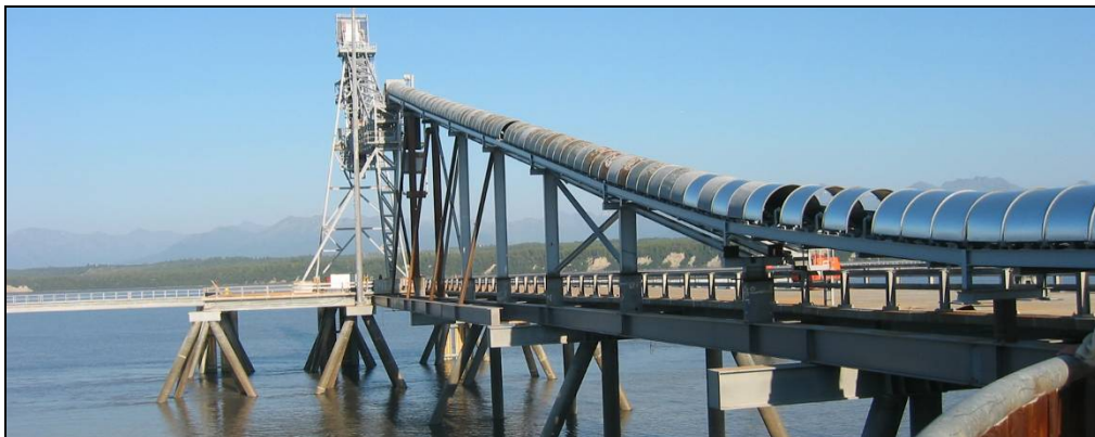
Figure 6.5.8: Dock and chip loading facility at Point MacKenzie.
