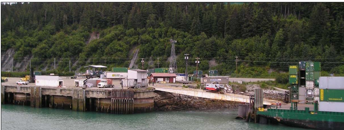
Figure 6.1.7: Existing heavy cargo dock (Lutak Dock) at Haines.
