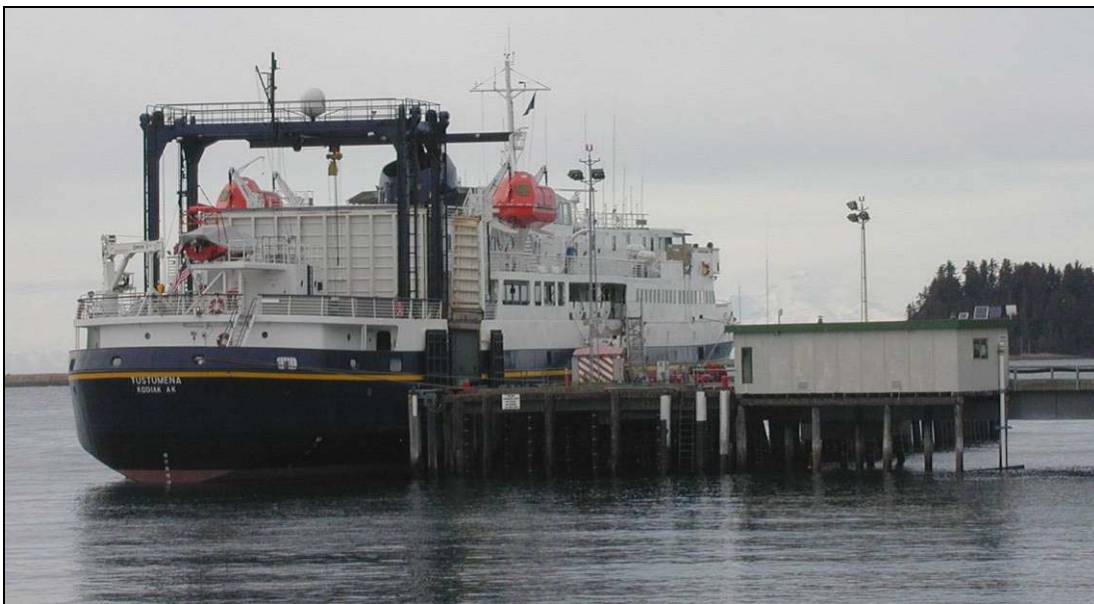
Figure 6.5.9: Pile supported dock at Seldovia.
