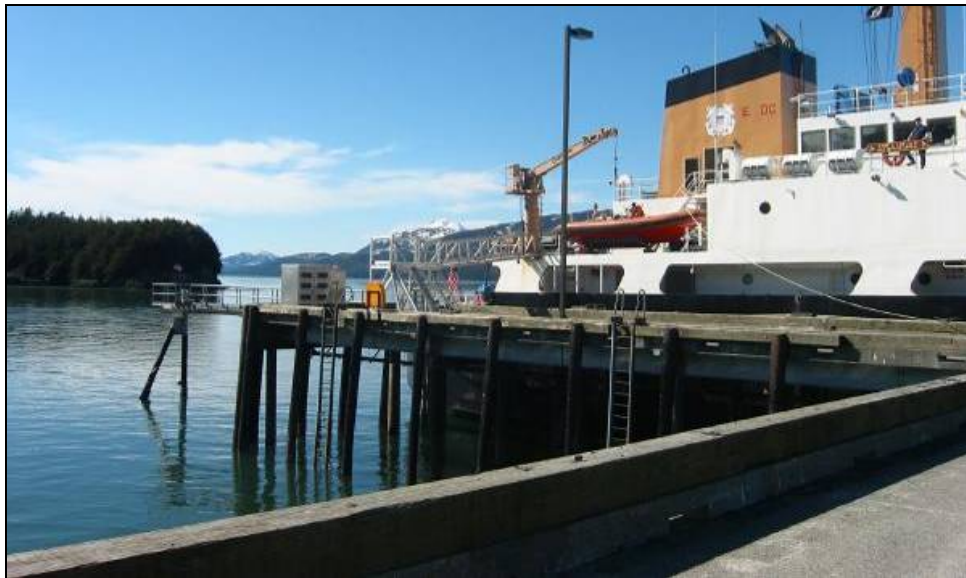
Figure 6.5.5: Pile supported concrete dock at Cordova, USCG Cutter moorage.
