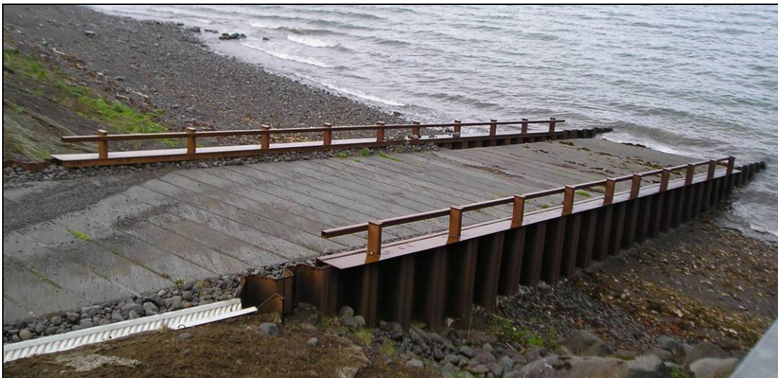
Figure 6.3.4: Concrete Launch Ramp (Heavy Haul-Out) Facility at Cold Bay.
