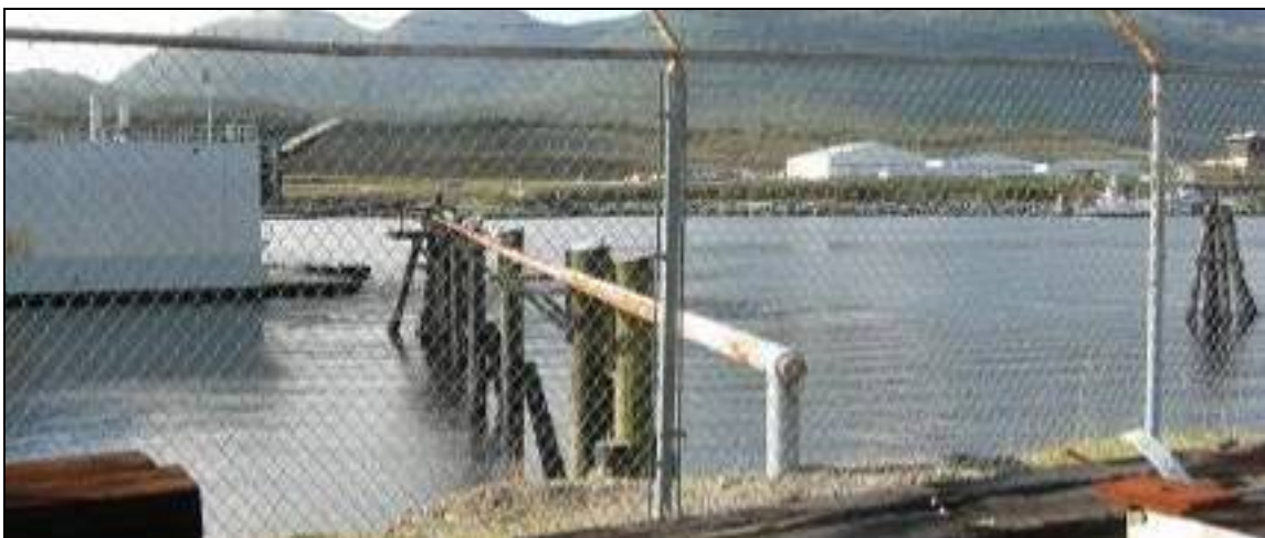
Figure 6.2.6: Fuel Line to Barge Berth at Ketchikan.
