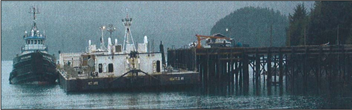
Figure 6.4.7: Existing Dock at Ouzinkie (©K-Sea Transportation Corp.).
