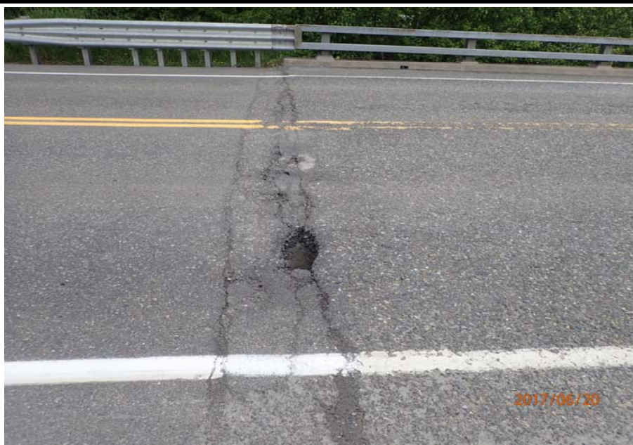
Bridge No. 0747 Br. Name Ward Creek Date 06/20/17 Inspector Manning / McRae Frame 15 FE joint, potholes in LT lane
