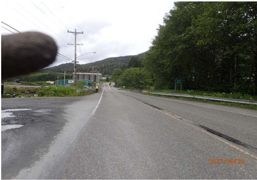
Bridge No. 0747 Br. Name Ward Creek Date 06/20/17 Inspector Manning / McRae Frame 1 Ahead at bridge
