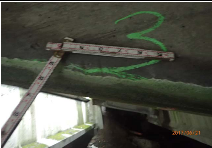
Bridge No. 0725 Br. Name Hoadley Creek Date 06/21/17 Inspector Manning / McRae Frame 27 US cantilever support side 3 crack
