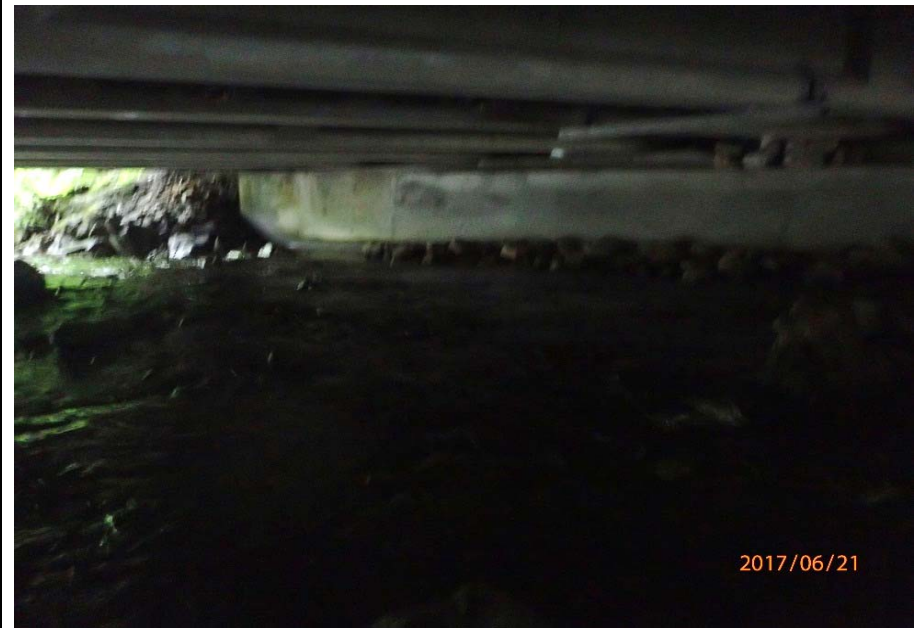
Bridge No. 0725 Br. Name Hoadley Creek Date 06/21/17 Inspector Manning / McRae Frame 12 FE abutment (DS)
