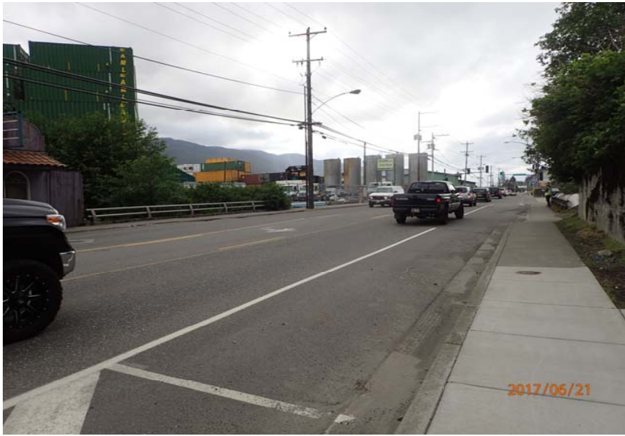
Bridge No. 0725 Br. Name Hoadley Creek Date 06/21/17 Inspector Manning / McRae Frame 1 Ahead at bridge
