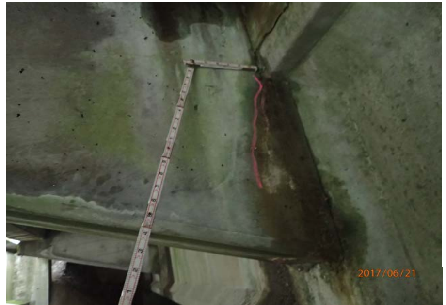
Bridge No. 0725 Br. Name Hoadley Creek Date 06/21/17 Inspector Manning / McRae Frame 26 US cantilever support side 3 crack
