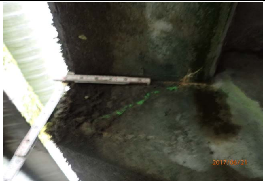
Bridge No. 0725 Br. Name Hoadley Creek Date 06/21/17 Inspector Manning / McRae Frame 28 US cantilever support side 3 crack
