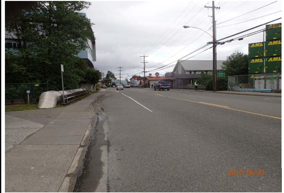
Bridge No. 0725 Br. Name Hoadley Creek Date 06/21/17 Inspector Manning / McRae Frame 2 Back at bridge
