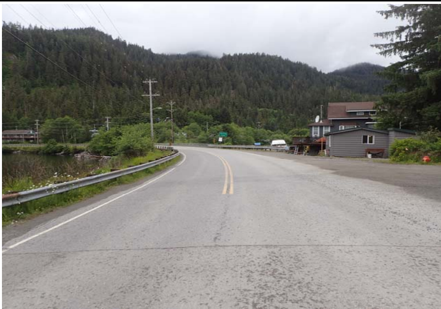
Bridge No. 0253 Br. Name Herring Cove Date 06/25/17 Inspector Manning / Escamilla Frame 3 Back at bridge
