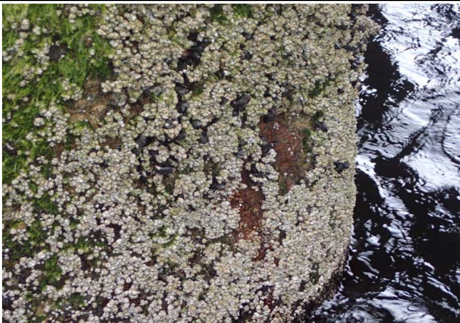
Bridge No. 0253 Br. Name Herring Cove Date 06/25/17 Inspector Manning / Escamilla Frame 23 Pier 2 NE LT spall has exposed rebar
