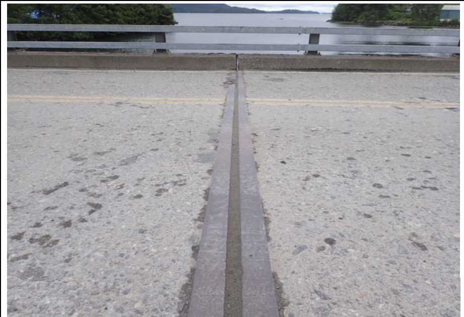
Bridge No. 0253 Br. Name Herring Cove Date 06/25/17 Inspector Manning / Escamilla Frame 16 Pier 2 joint
