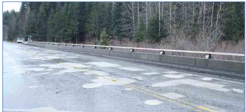
Figure 1. Snow River West Deck Condition
