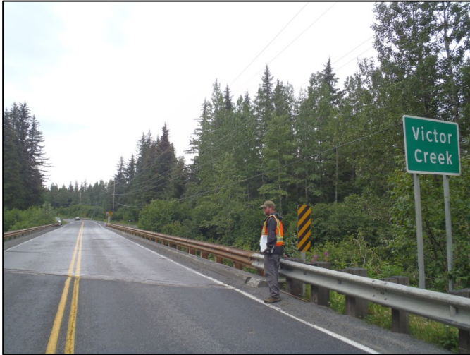
Figure 4. Victor Creek Bridge
