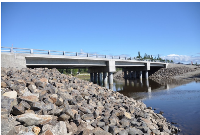
Figure 2 Typical CFST Substructure Units
