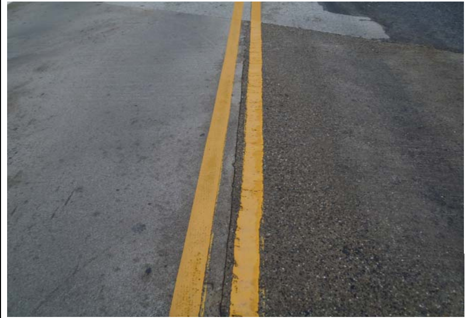
Bridge No. 1141 Br. Name Antler Creek Date 07/16/17 Inspector Murray / Knapp Frame 6 NE Approach Slab
