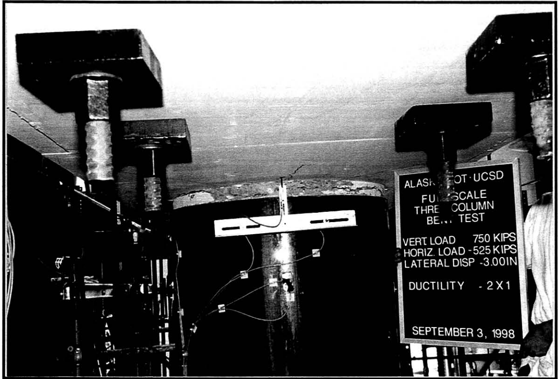
Fig.7-16 Extent of Spalling of Cover Concrete at \mu_d = \pm 2x1 - Interior Column IC
