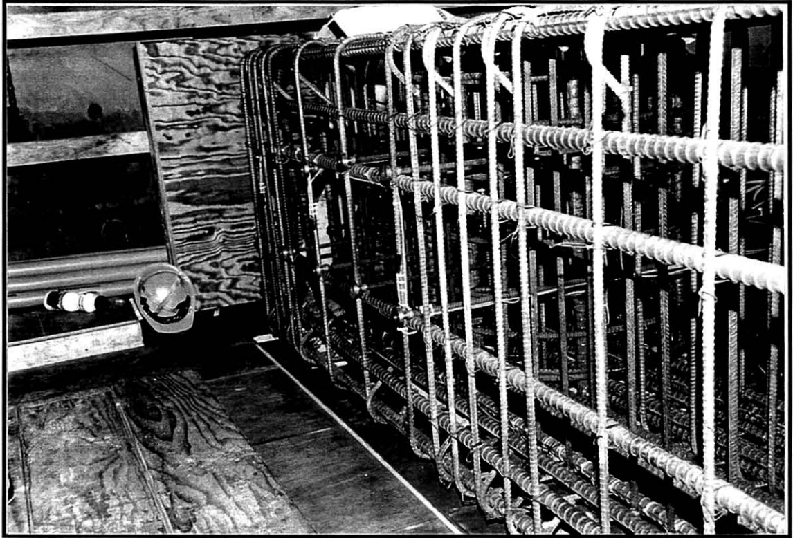
Fig.5-9 Side View of the Completed Reinforcement Detail Near Exterior Joint KJI
