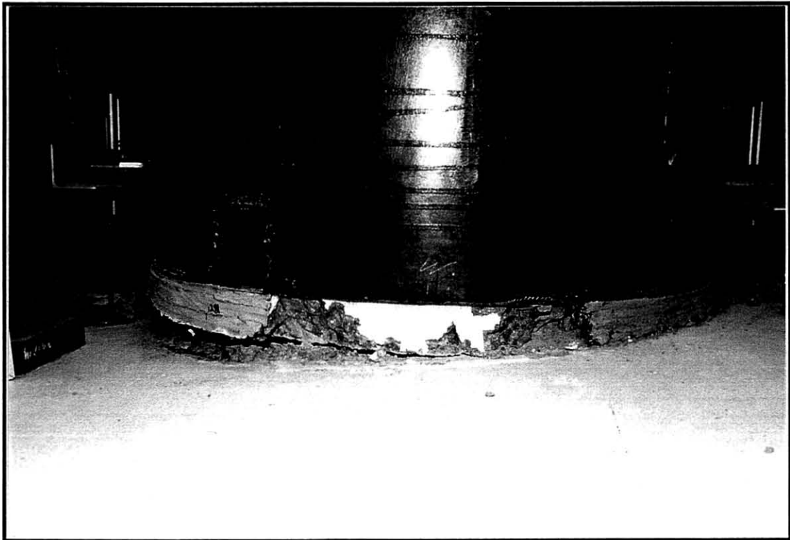
Fig.7-33 Extent of Spalling - Typical at Base of All Three Columns
