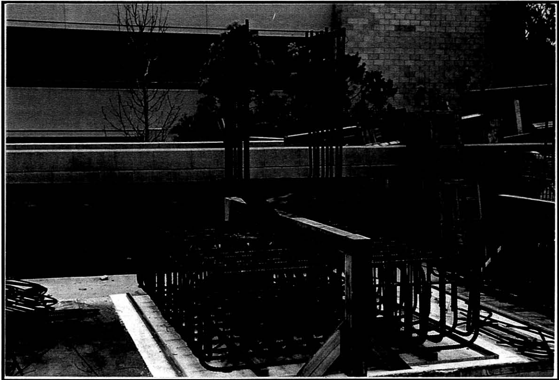
Fig.5-1 A Completed Footing Reinforcement Cage Prior to Casting
