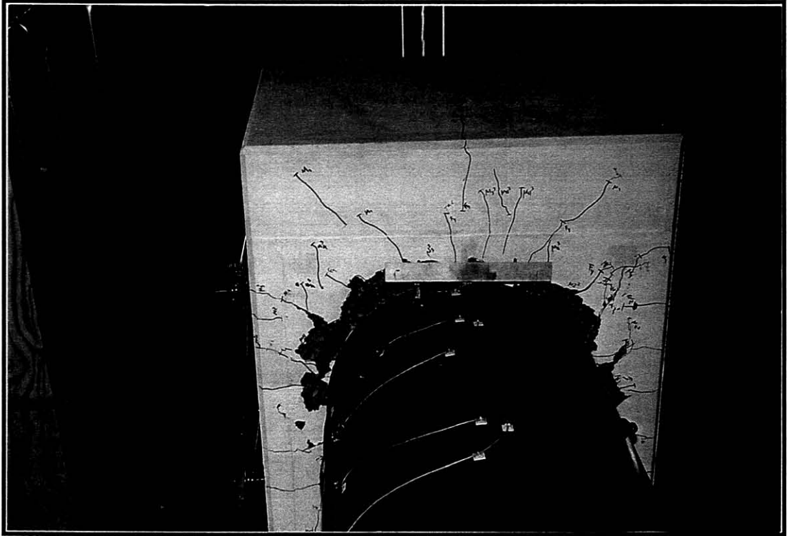
Fig.7-28 Strain Penetration Damage at \mu_d = -10x2 ( Pull ) - Exterior Joint KJ1
