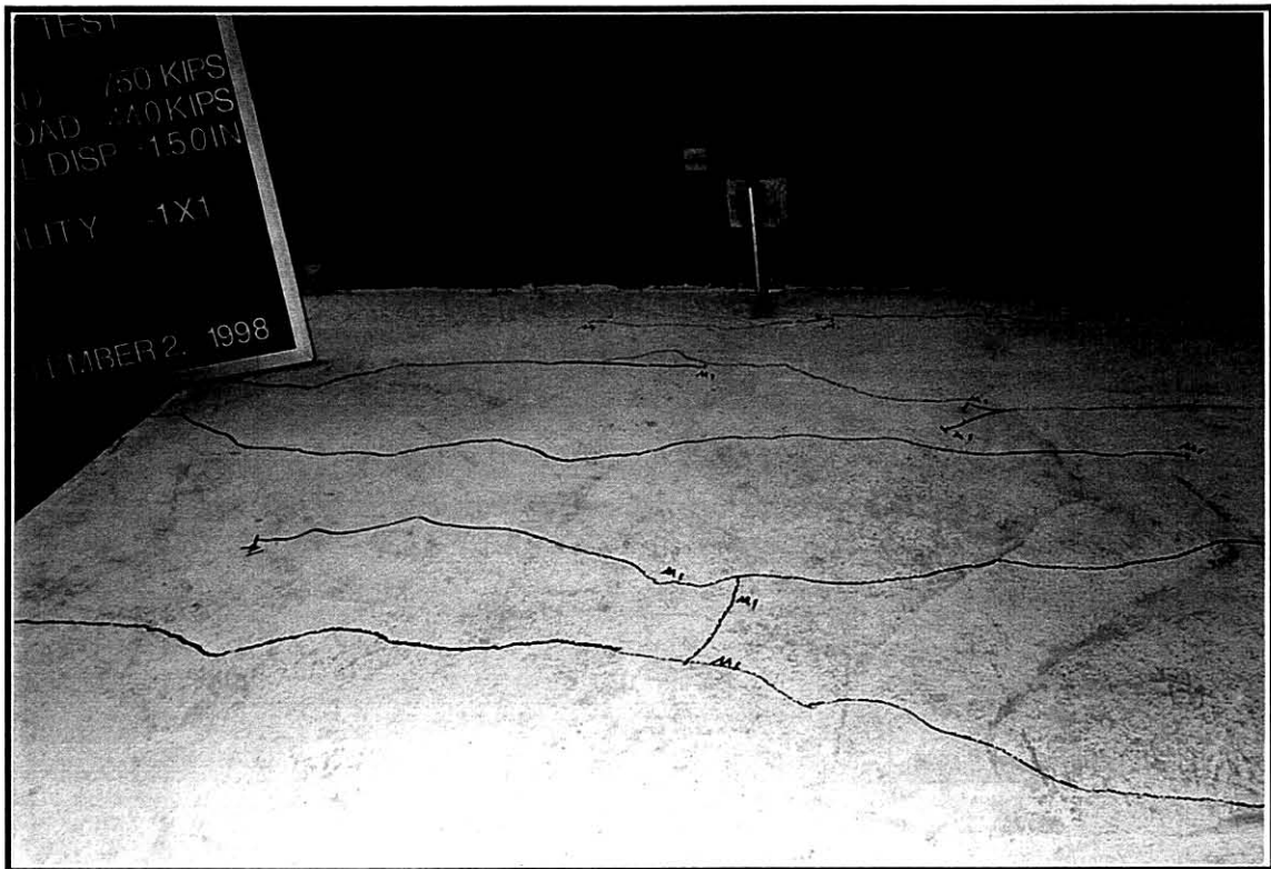
Fig.7-13 Flexural Cracks on Top of the Cap Beam - Exterior Joint KJI
