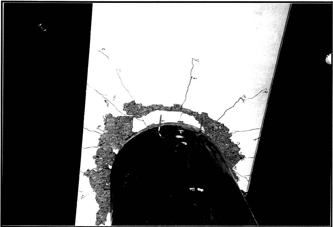
Fig.7-31 Strain Penetration Damage at \mu_d = -10x2 ( Pull ) - Interior Joint TJ
