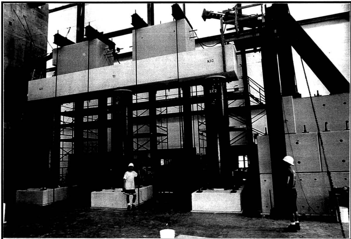
Fig.5-14 Completed Test Unit Prior to Testing
