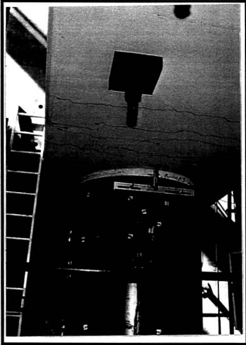
Fig.5-20 Top of Column External Instrumentation
