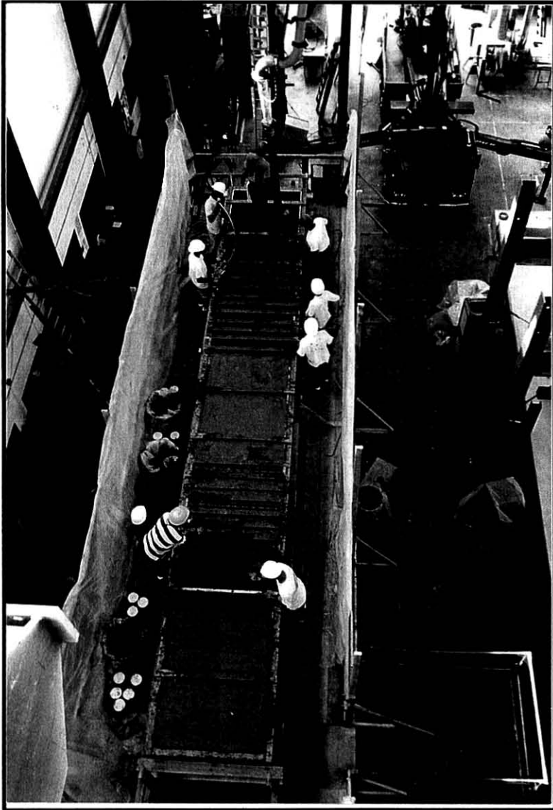
Fig.5-12 Casting of the Cap Beam
