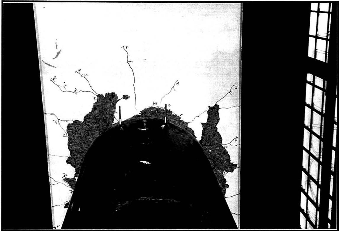
Fig.7-30 Strain Penetration Damage at \mu_d = +10x2 ( Push ) - Interior Joint TJ
