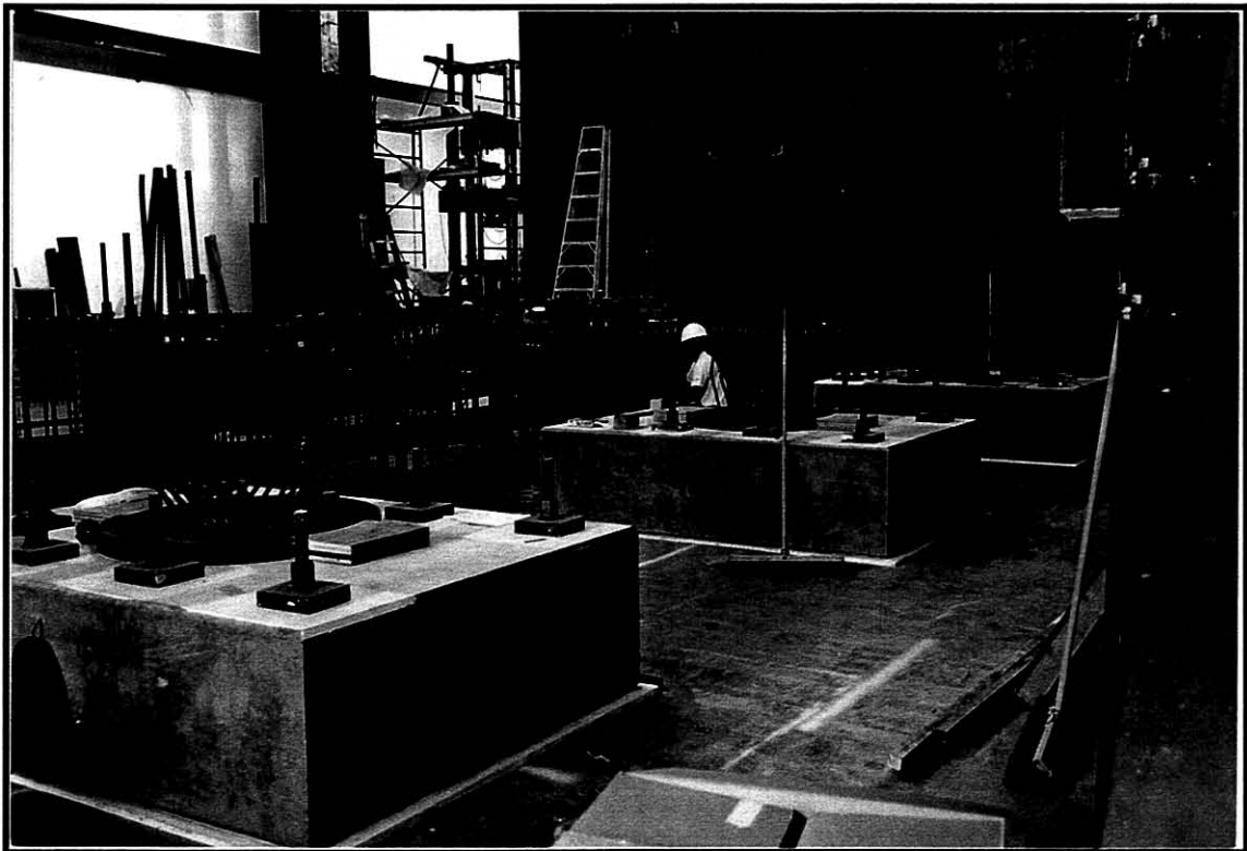
Fig.5-2 Footings in Place Prior to Construction of Columns
