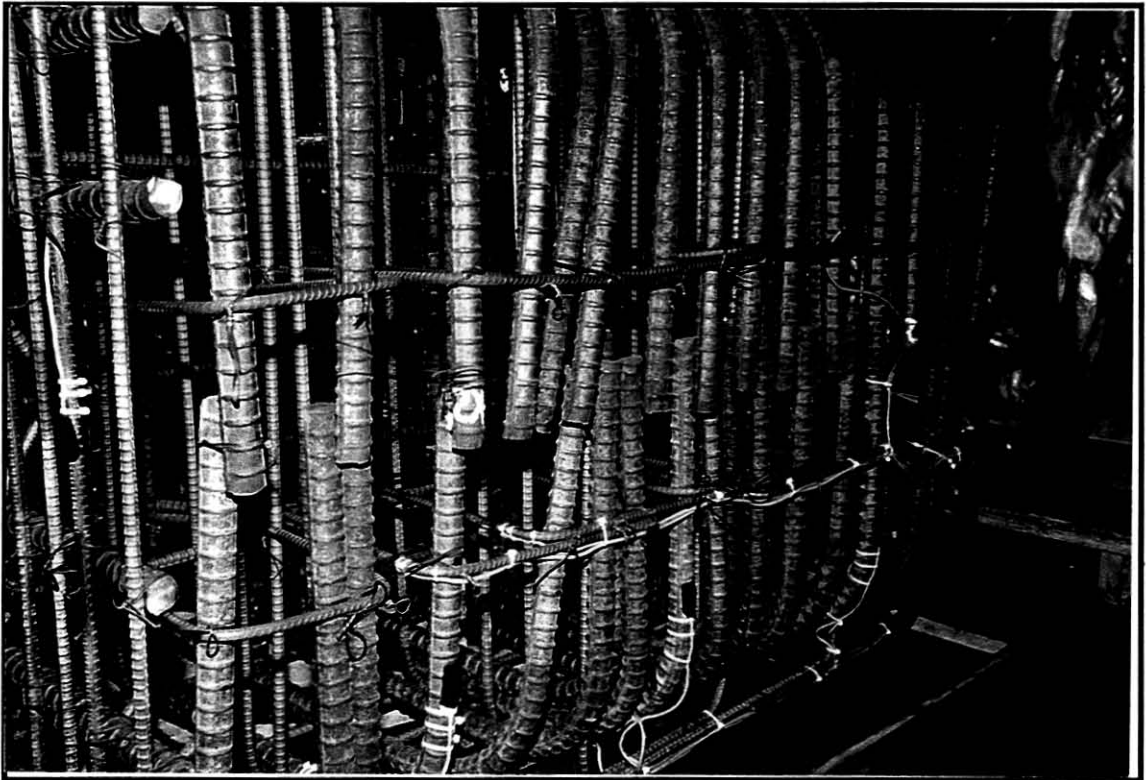
Fig.5-10 Reinforcement Detail at End of Cap Beam With Horizontal U-Pins in Place
