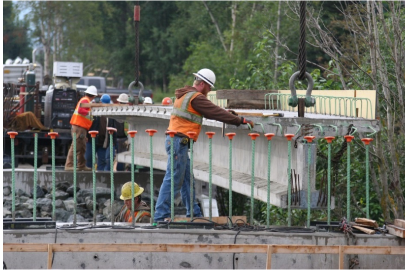
Figure 3 "Alaska-Style" Prestressed Girder Installation
