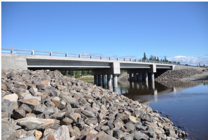
Figure 2 Typical CFST Substructure Units
